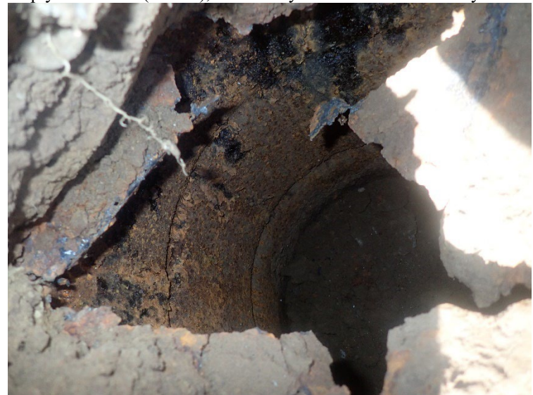
Close-up view inside the empty drum.
