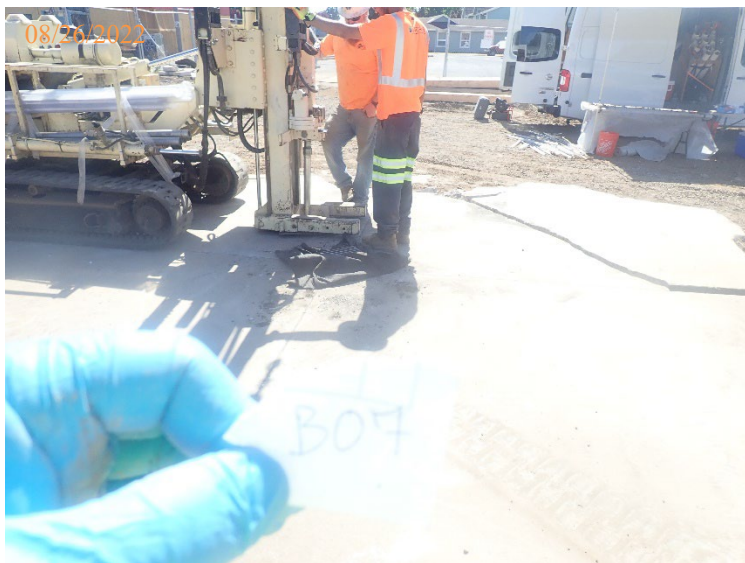
Drilling B07 near the storm water catch basin.
