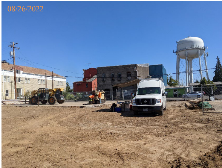
Drilling B07, midway along the southeastern site boundary.
