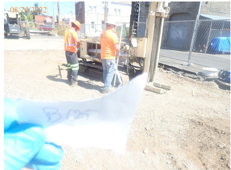
Boring B05 near the S corner of the site – view east.
