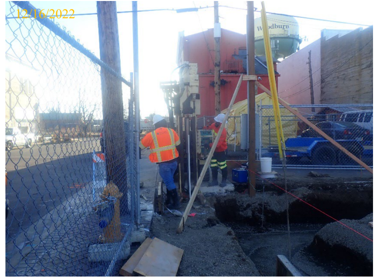
Direct-push drill rig set up at B12 – view southeast.
