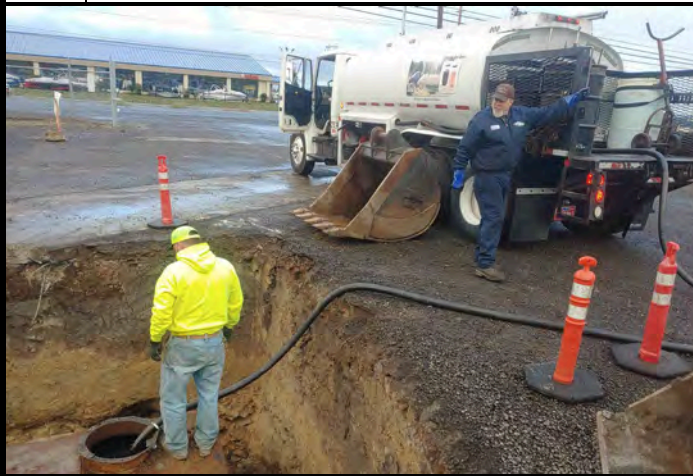
Photo #5: ORRCO Pumping Out Tank Liquids
