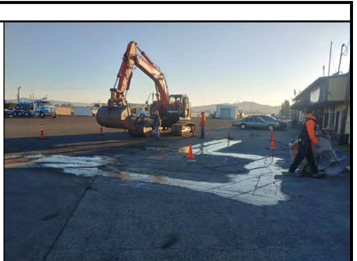
Photo #2: Concrete Cutting
