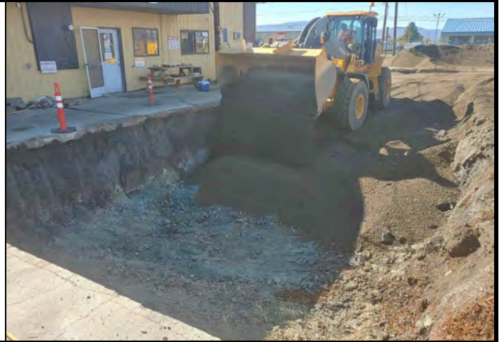
Photo #14: Backfilling Product Line Trench
