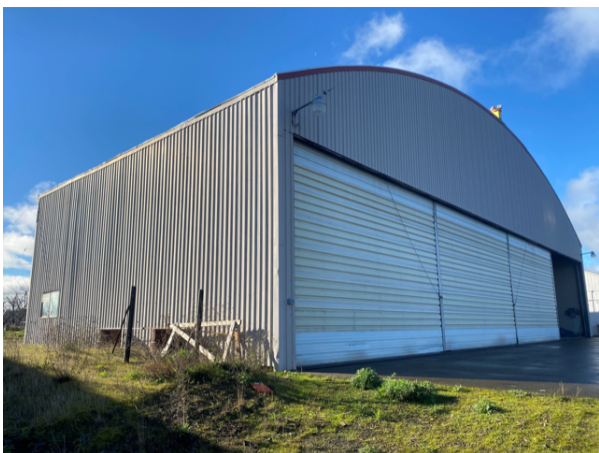
Photo 1. Hangar at 3604 Airport Drive in Hood River, OR. The UST is roughly halfway down left side of hangar. View is to the SW.
