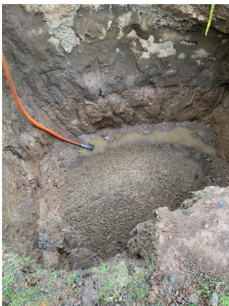
Photo 15. Drained tank pit from Photo 14.
