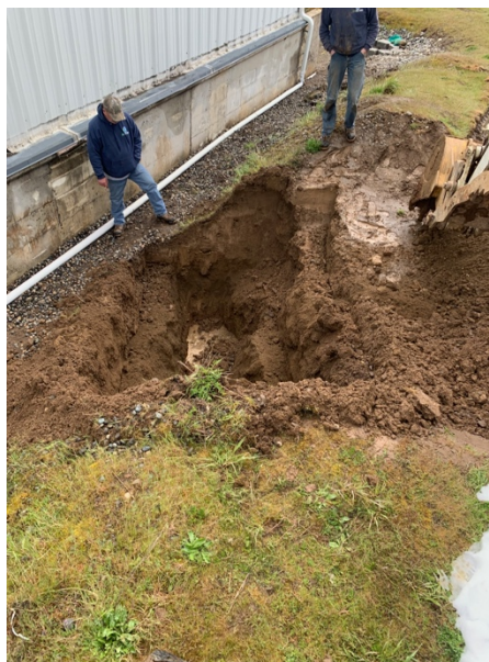
Photo 18. Groundwater recovery trench to the NE of the former tank excavation pit. View is to the SE.
