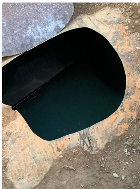
Photo 8. Water recharging the tank through holes after pumping the fuel and triple-rinsing the interior.
