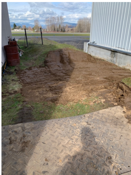
Photo 17. Tank excavation pit restored to grade with clean soil. View is to the NNE.
