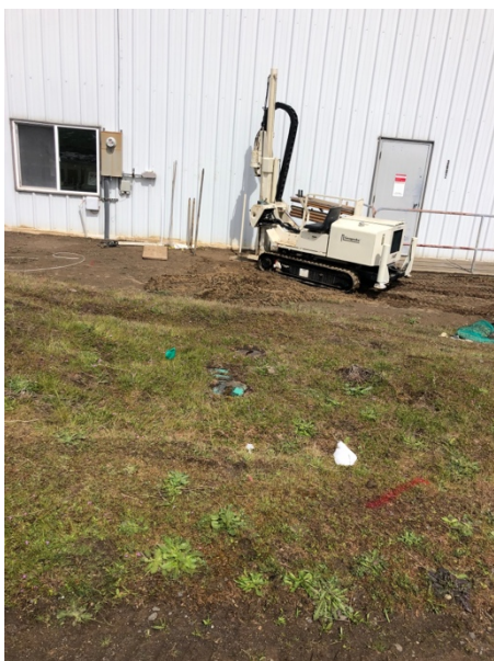
Photo 23. Geoprobe completing boring 15 on the S side of 3602 Airport Drive, to the SE of the removed tank area.
