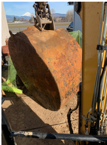
Photo 10. UST being removed from the tank pit. Tank was cut in half for removal.
