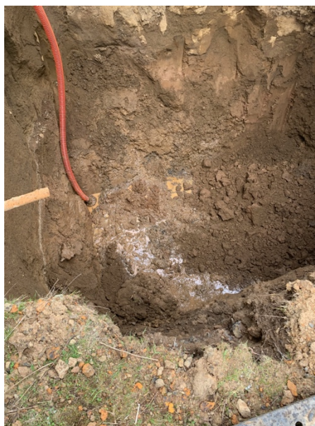
Photo 12. ORRCO pump hose removing groundwater in the tank pit.
