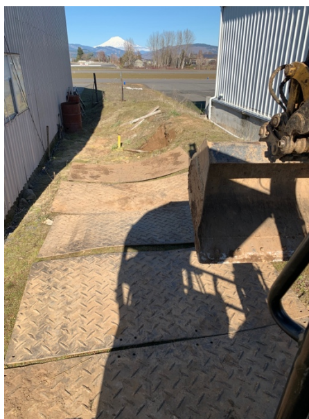
Photo 4. Location of UST before digging. View is to the N. Mt. Adams in background for reference.
