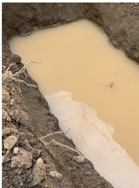
Photo 20. Groundwater recharge trench full of groundwater. No oily sheen or smell was observed.
