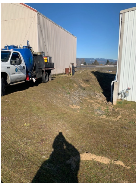
Photo 3. Wider view of UST site. View is to the NNW. Notice slope is towards the hangar on the right.
