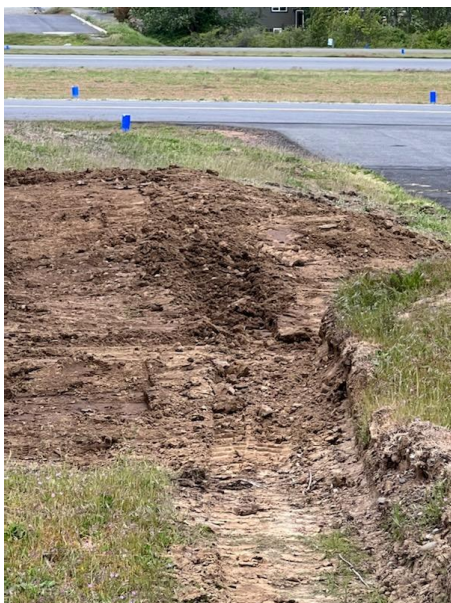
Photo 21. Groundwater recovery trench backfilled and restored to grade with clean overburden.
