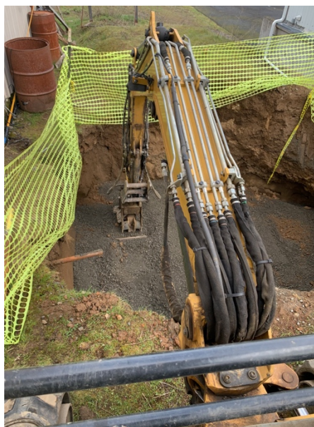
Photo 16. Compacting gravel during backfilling process of the tank pit.
