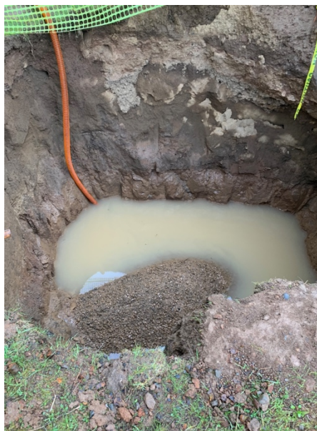
Photo 14. Groundwater in tank pit with ORRCO pumping hose.
