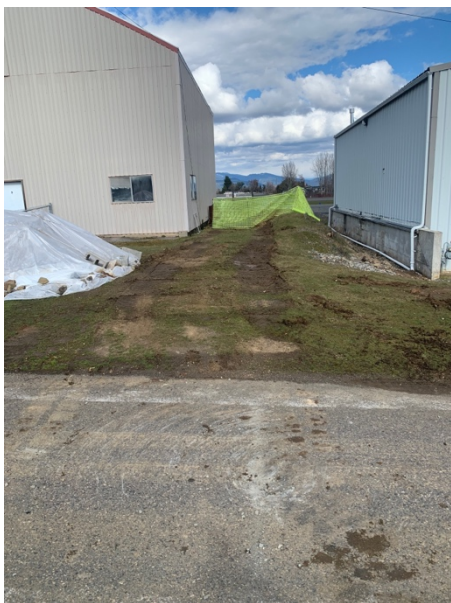
Photo 13. Overview of site. UST excavation fenced off in center of photo. Contaminated soil on left side of photo under white tarp.
