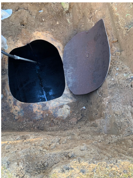
Photo 7. Triple-rinsing the interior of the UST after pumping the fuel found inside.
