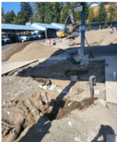
Photo #5 Former dispenser area
