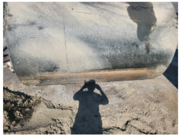
Photo #4 2,000-gallon diesel UST. Minimal rust on bottom of UST. No holes observed
