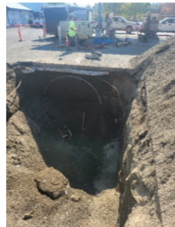
Photo #2 UST pit: 5,000-gallon gasoline UST pit
