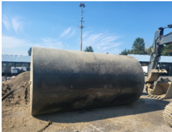
Photo #3 5,000-gallon gasoline UST. No visual corrosion
