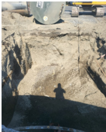
Photo #1 UST pit: 2,000-gallon diesel UST
