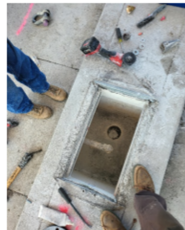
Photo #6 Clean sump under former dispenser location
