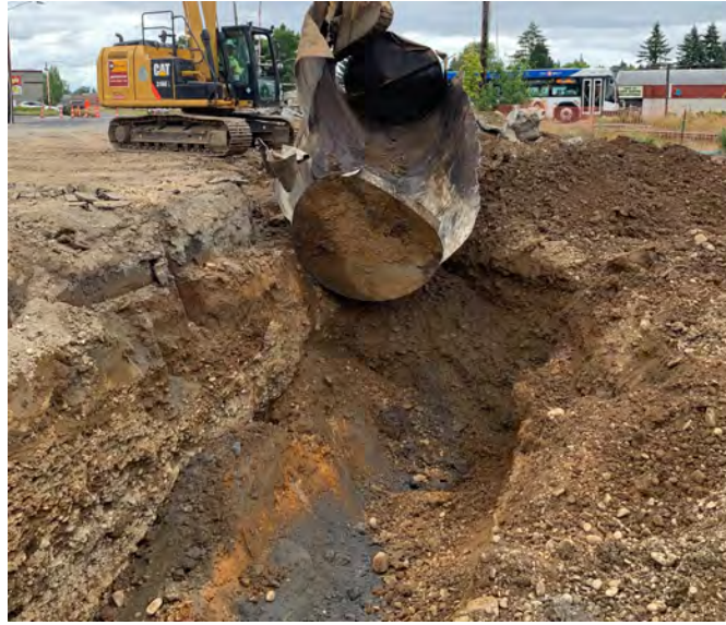
Tank 3 was removed from the ground.
