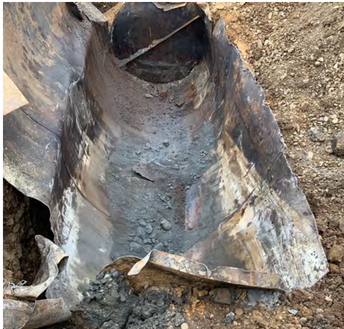
Tank contents were removed and interior thoroughly cleaned.
