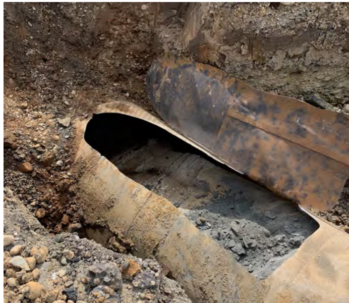
The tank was found filled with concrete slurry.
