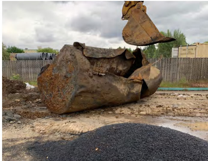
Tank 1 and associated piping were removed from the ground.
