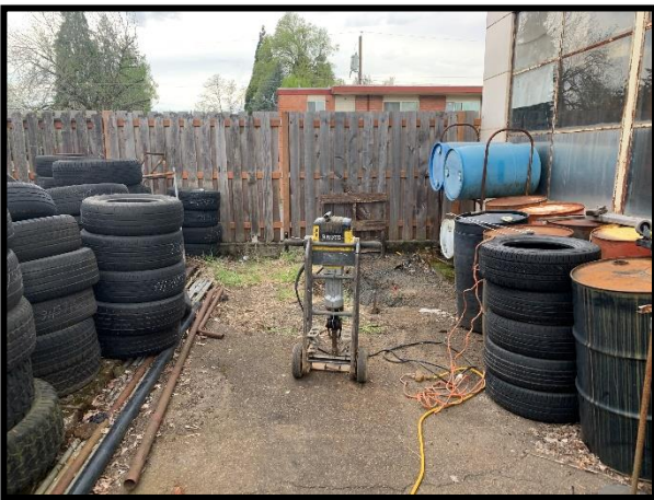
PHOTOGRAPH NO. 3 – Sampling waste oil tank location with GeoProbe sampler and jack hammer.
