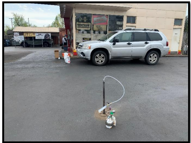
PHOTOGRAPH NO. 4 – Location of SG1 west of former UST pit.
