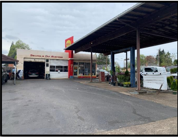
PHOTOGRAPH NO. 1 – View of Building.
