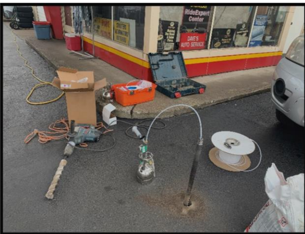
PHOTOGRAPH NO. 5 – Location of SG2 near corner of building and southwest of former UST pit.
