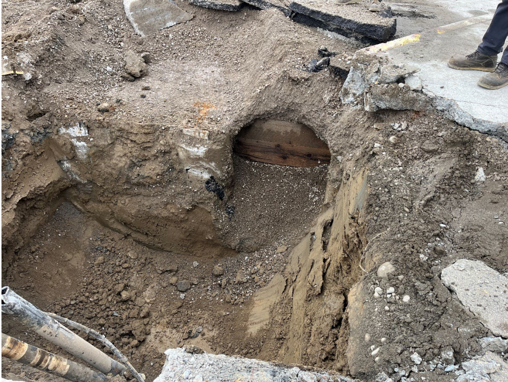
Photo 4: Excavation extended below the product lines and sluffing pea gravel from the tank nest.
