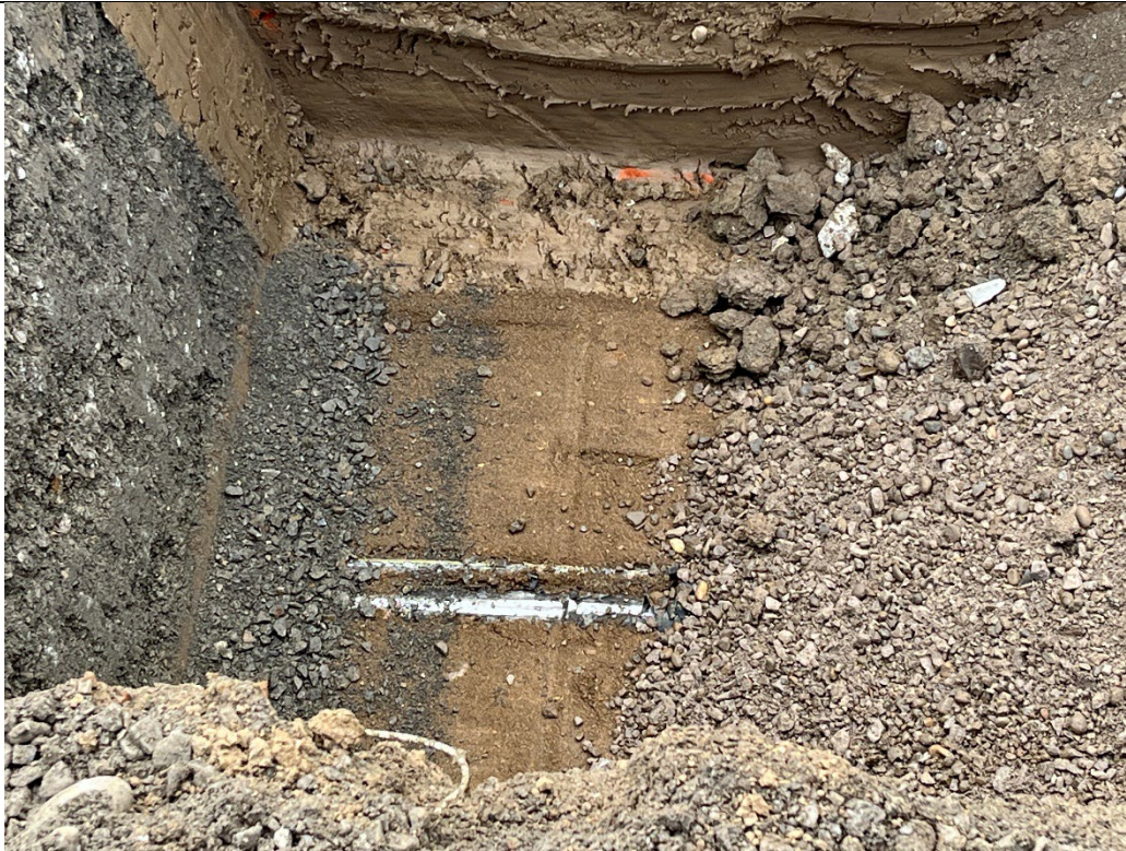
Photo 1: Exposed product lines in excavation.
