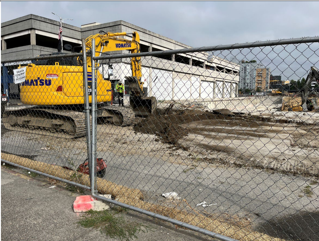
Photo 5: Backfilling of the excavation with removed soil.
