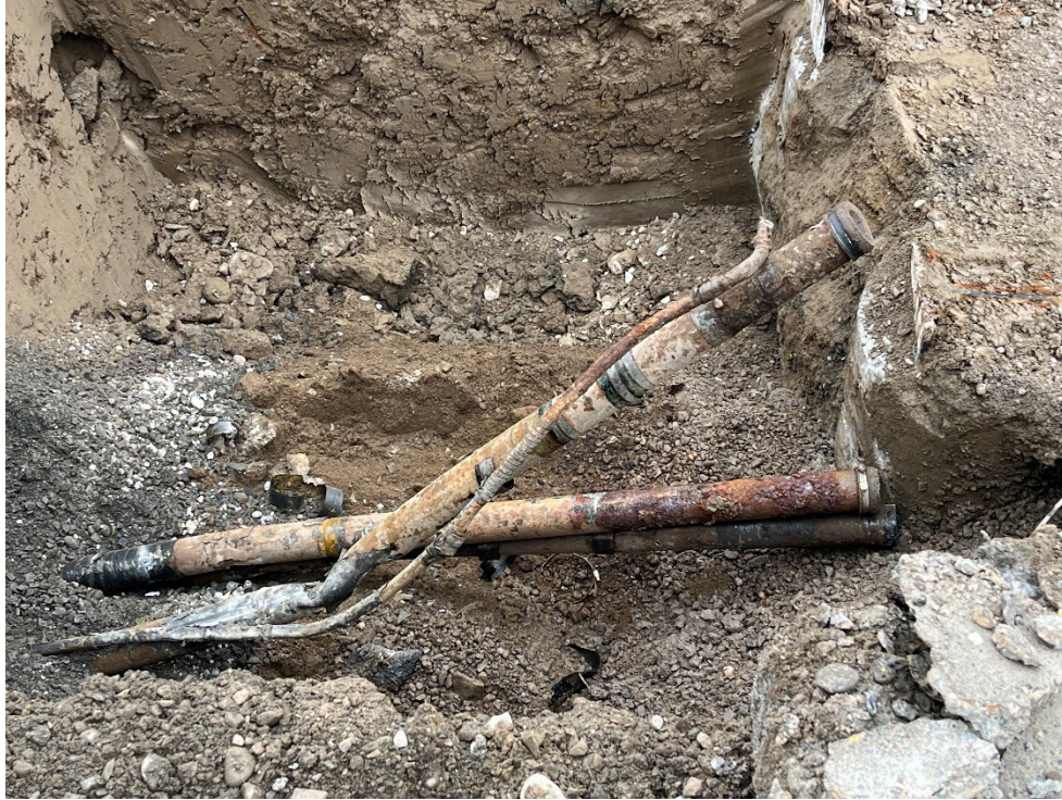
Photo 2: Removal of exposed product lines.
