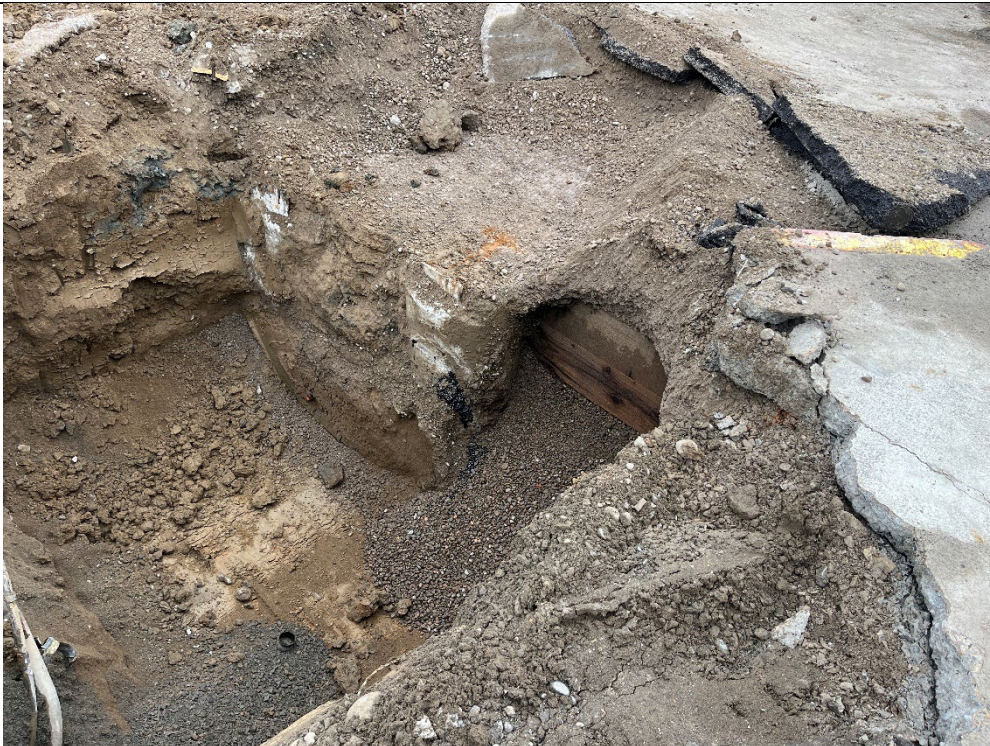
Photo 3: Excavation below the product lines. Note the concrete piles and wood tank nest shoring
