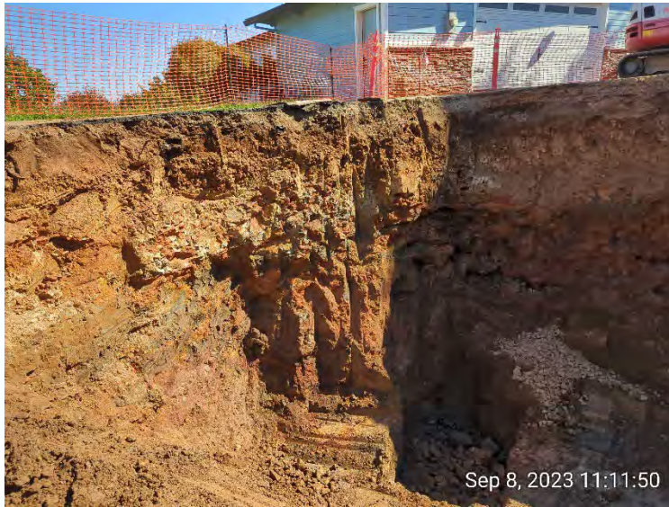
Sump excavated in the NE corner of EX01.
