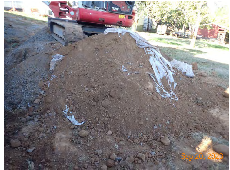
Based on confirmation test data, removed overburden soil from EX02 was loaded into trucks and transported to Hillsboro Landfill for disposal September 22, 2023.
