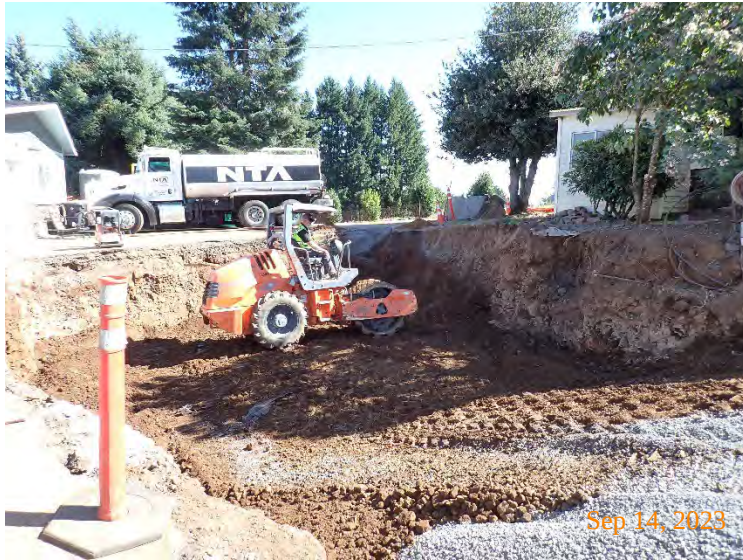
After analysis showed the overburden soil was clean, Stockpiled overburden soil was placed and compacted above the crushed rock.
