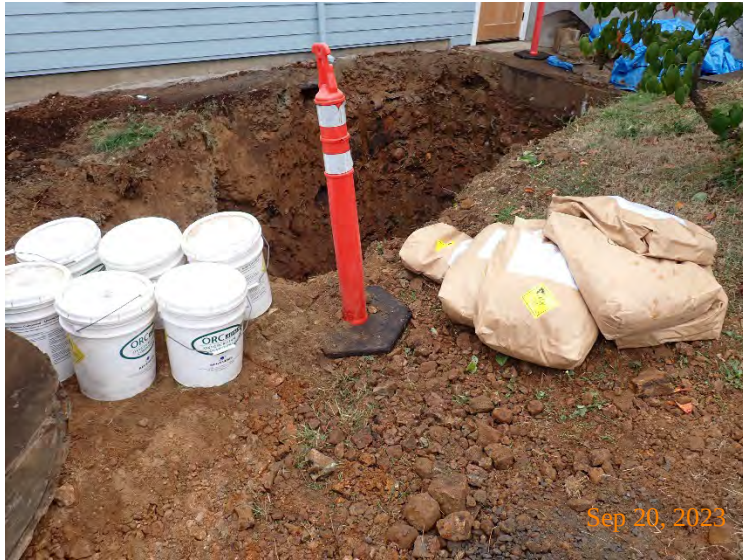
495.9 lbs of Persulfox, 150 lbs of ORC, 120 lbs of Regenox Part A, and 150 lbs of Regenox Part B were added to EX02.
