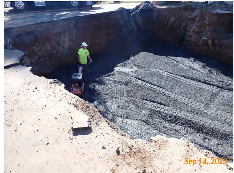
Compacting ¾-minus crushed rock in lifts above the larger diameter aggregate layer to a level of approximately 8 feet below finish grade.
