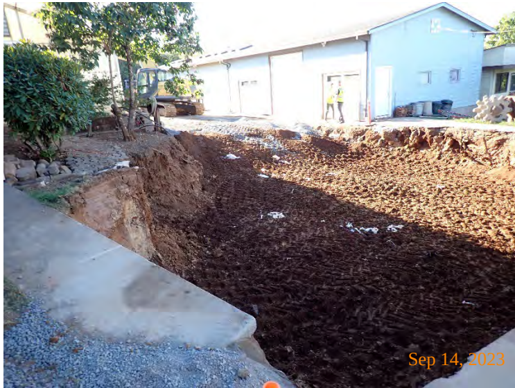
Stockpiled clean overburden soil was brought up to a level of approximately 3 feet below finish grade.
