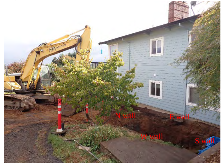
Confirmation samples were collected from the floor (GS34), N wall (GS35), S wall (GS36), E wall (GS37), and W wall (GS38) at depths ranging from 15.5 to 18' bgs.
