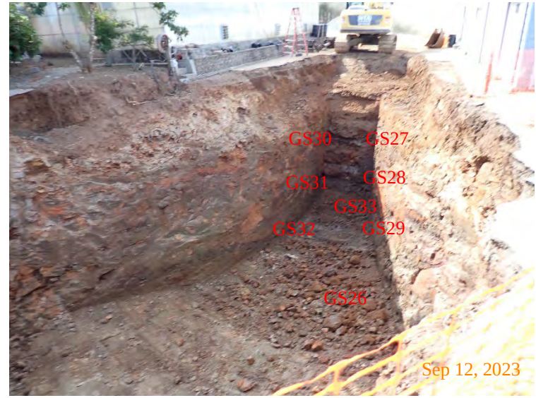
Collection of GS26@20', GS27@10', GS28@14', GS29@18', GS30@10', GS31@14', GS32@18', and GS33@21' at east end of EX01.
