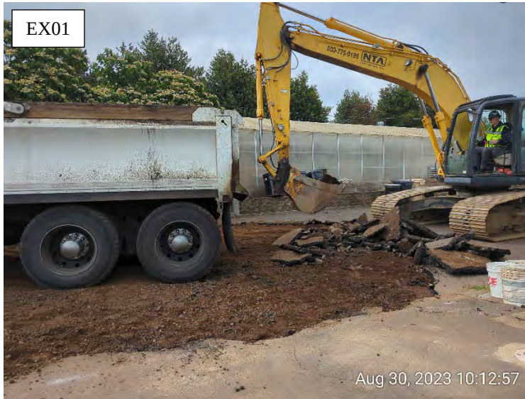
NTA loading asphalt into WTF dump truck to be taken offsite for disposal - view southwest.
