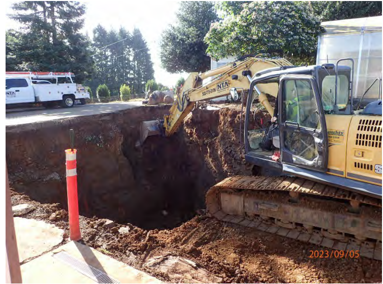
NTA set up excavator on west bench to excavate east side of EX01, where PID detected >5000 ppm volatiles.
