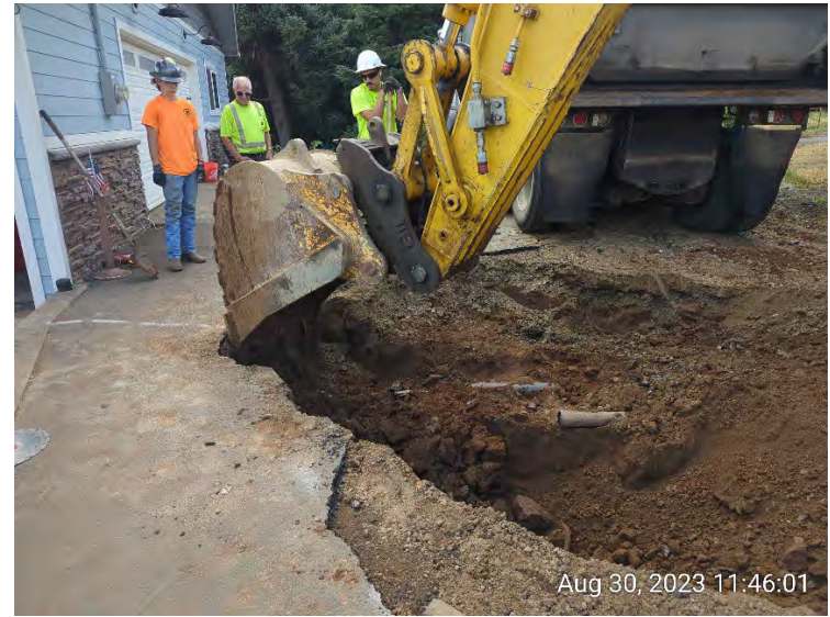
Two buried power conduits were encountered when excavating near the southwest corner of the house – view facing east.
