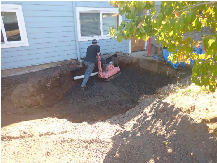
Crushed aggregate was compacted in lifts.
