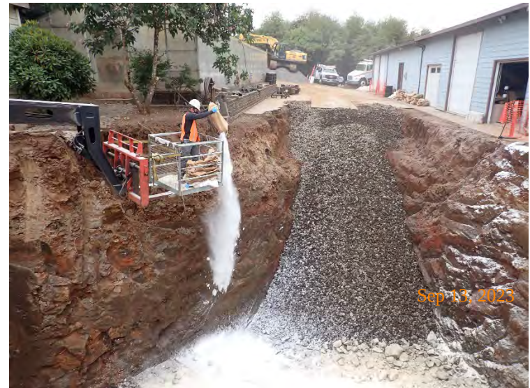
Application of 2,865.2 lbs of Persulfox oxidizer and 400 lbs of Oxygen Release Compound (ORC) in EX01.
