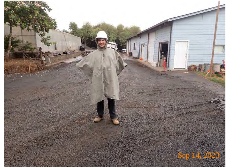
EX01 completely backfilled with compacted crushed rock to subgrade, i.e., 3 inches below finish grade. New asphalt pavement to be installed.
