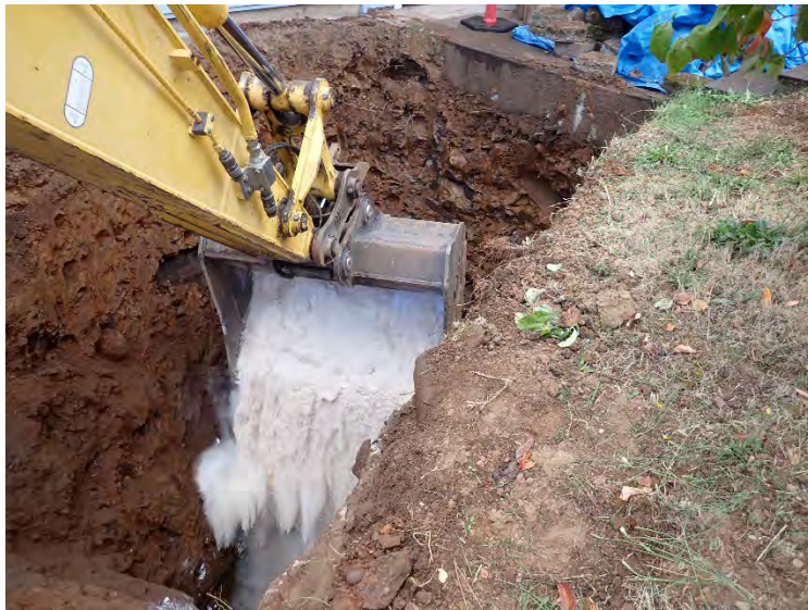
These oxidizers were mixed in a bucket and applied on the floor of EX02.
