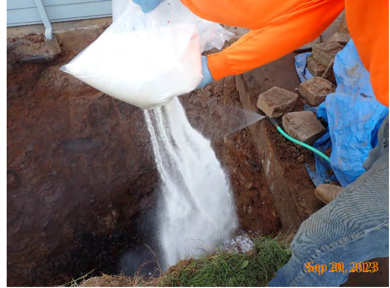
Additional PersulfoX and ORC wetted with water were interlayered with clean aggregate as EX02 was backfilled.
