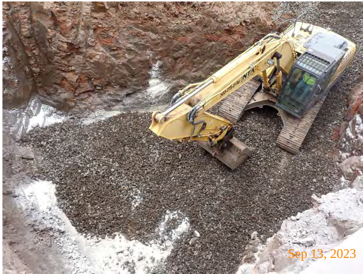
Spreading clean aggregate over the Persulfox and ORC layer up to 17 feet bgs.
