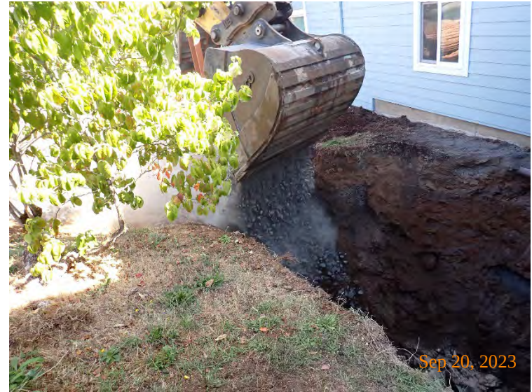
Clean aggregate backfill added to EX02.
