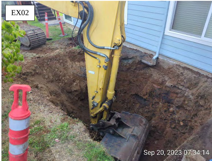
Excavation EX02 on the west side of the house at former location of UST T1 – view facing northeast.
