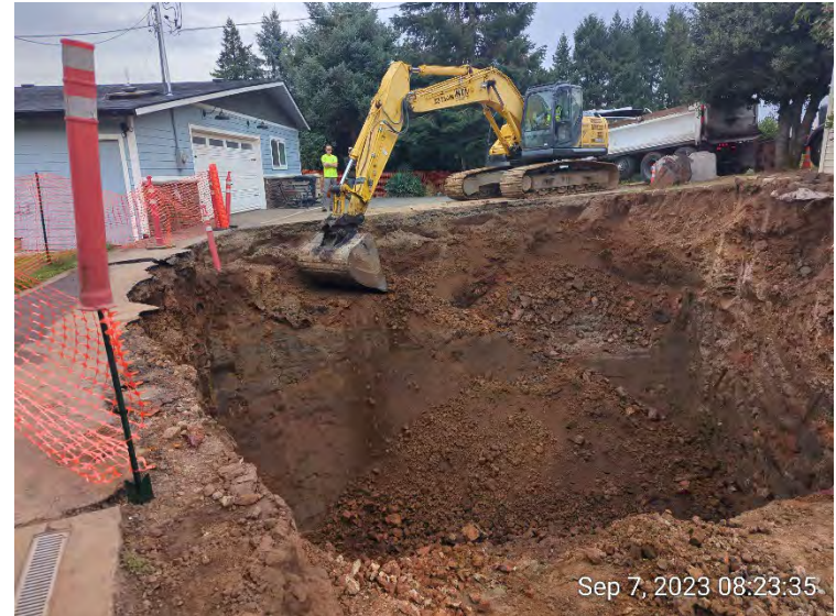
PCS removal along the east wall of EX01.
