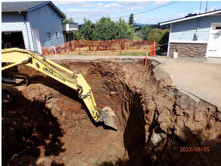
Field headspace volatiles were 150 ppm@9', 250 ppm@12', and 180 ppm at 17' at center of north wall (GS04, GS05, and GS06).
