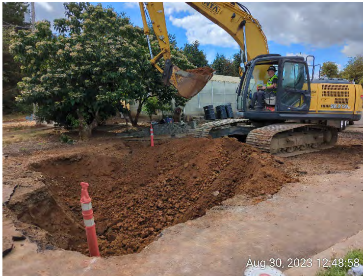
Removing clean overburden down to 5 feet bgs, which was temporarily stockpiled at the site.
