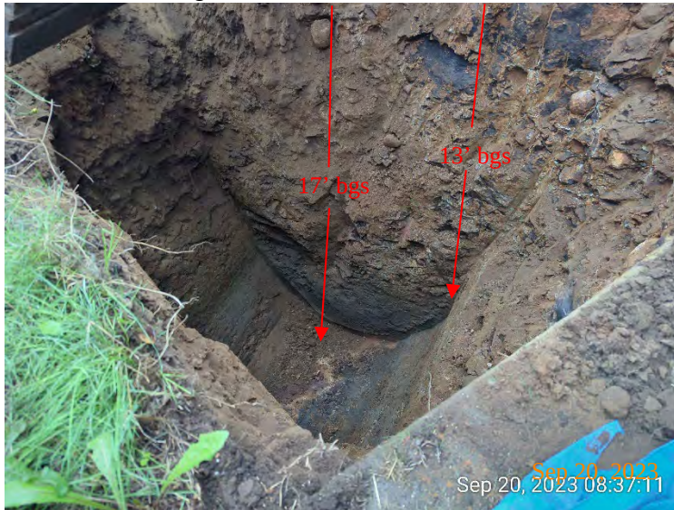
Gray petroleum-stained soil was encountered in EX02 from approximately 13 to 17 feet bgs.
