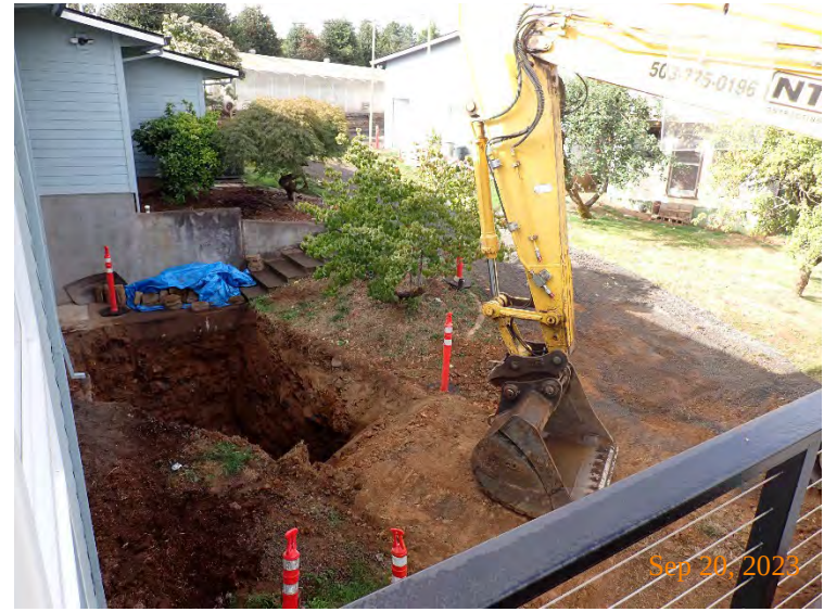
Following over-excavation of PCS, EX02 was approx. 14' to 15.5'-long by 6' to 10'-wide by 18'-deep.
