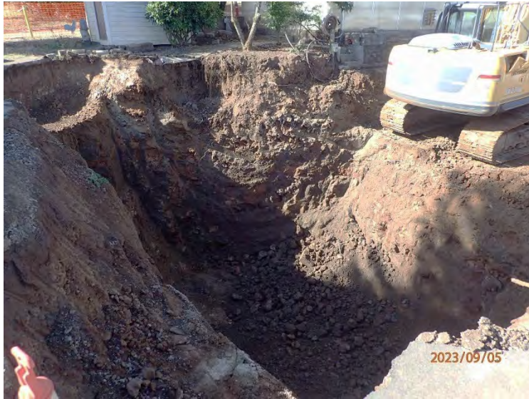
Collected GS03 at the soil/ water interface (SWI) at 17' bgs at the base of the south wall.
