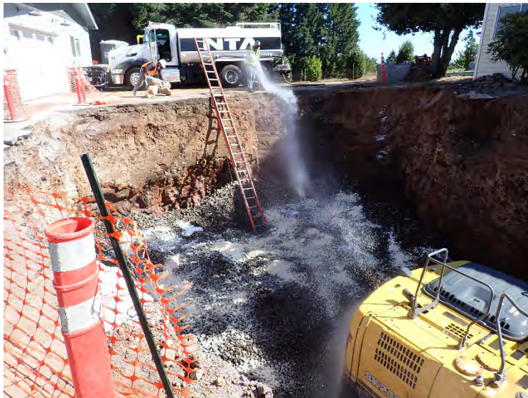
An additional 8,265 lbs of Persulfox and 1,120 lbs of ORC were applied over the aggregate layer, and wetted.
