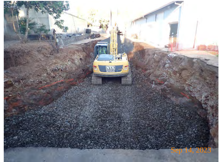
Aggregate was brought up to a level of 12 feet below finish grade.
