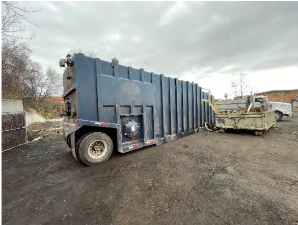
Photo #7 Baker Tank for water from tank nest excavation.
