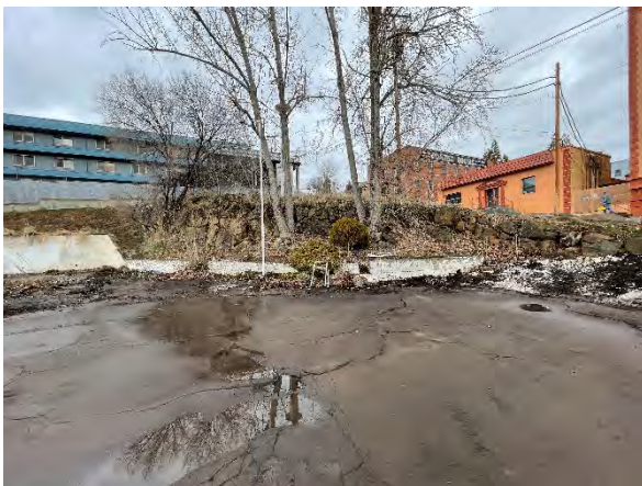
Photo #5 Northwest portion of subject property showing outcropping basaltic andesite bedrock and retaining wall.
