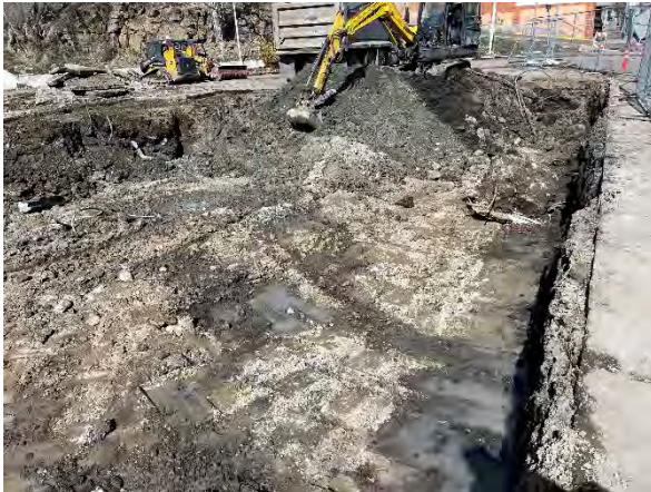
Photo #25 Remedial excavation extending to the north.
