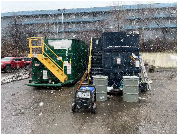
Photo #17 Baker Tank staging area and water treatment system.
