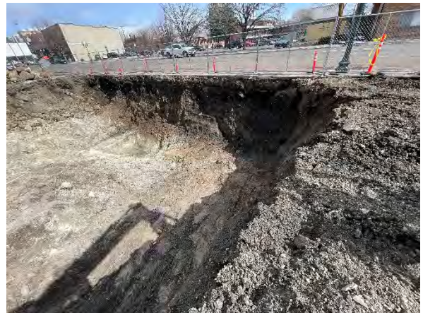
Photo #28 Excavation looking northeast toward Main Street – east sidewall shown.
