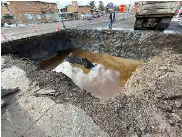
Photo #9 Ponded water remaining in tank nest excavation following UST removal.
