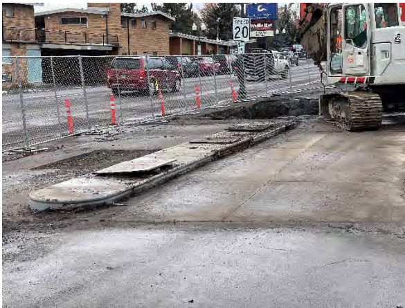
Photo #3 East pump island with two fuel dispenser sumps.
