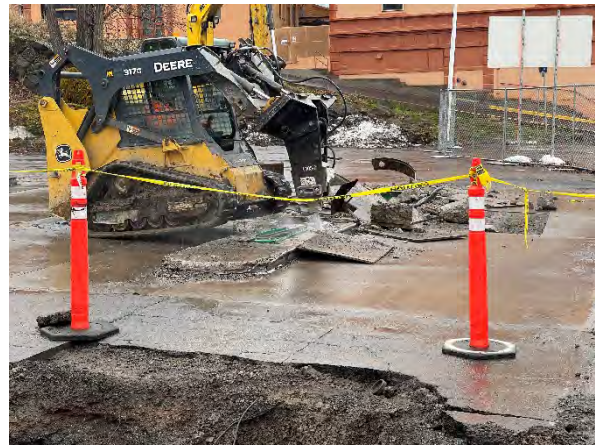
Photo #16 ES&S breaking apart concrete pump island.
