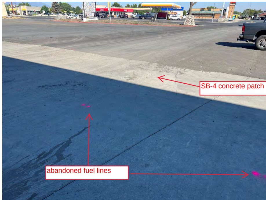
Photo 5. The abandoned fuel lines associated with the decommissioned underground storage tanks (USTs) are visible in pink paint. A large concrete patch associated with Broadbent and Associates' (Broadbent) SB-4 boring is visible a few feet to the north of the abandoned lines.
