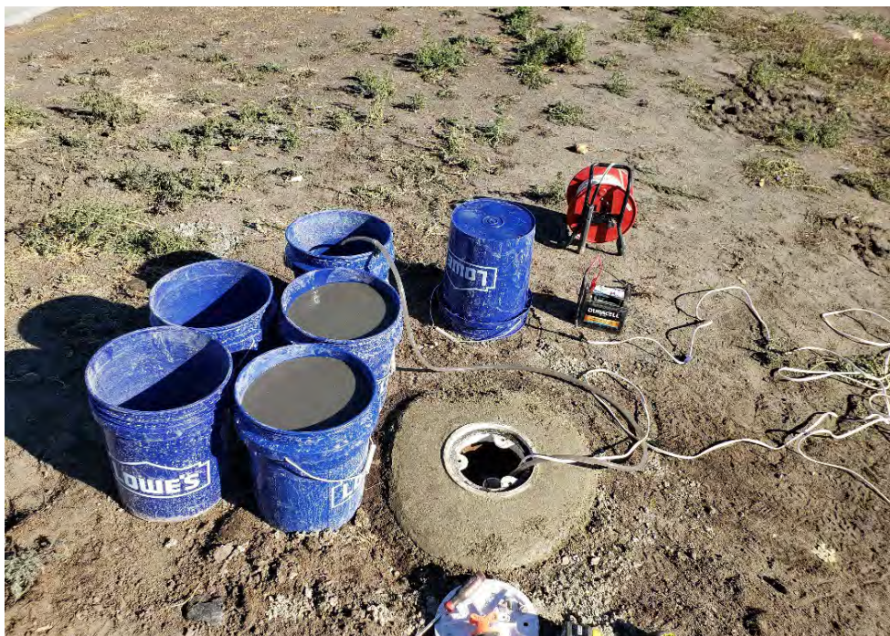
Photo 13. Monitoring wells were developed using a whale pump and steel bailer.
