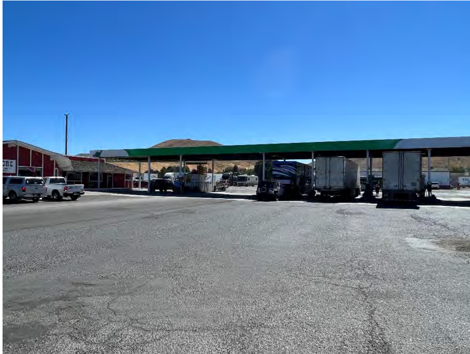
Photo 3. Looking south toward the semi-truck diesel pumps. The entrance to the convenience store, trucker lounge, and store offices is visible to the east of the pumps.
