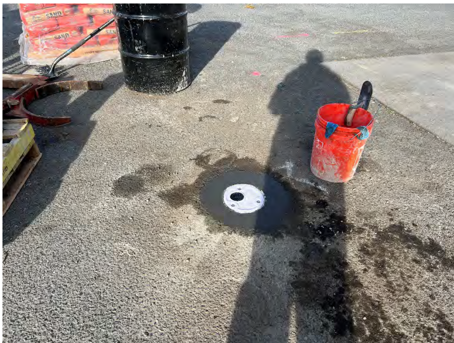
Photo 11. Monitoring wells were finished with heavy duty rated flush mount monuments.
