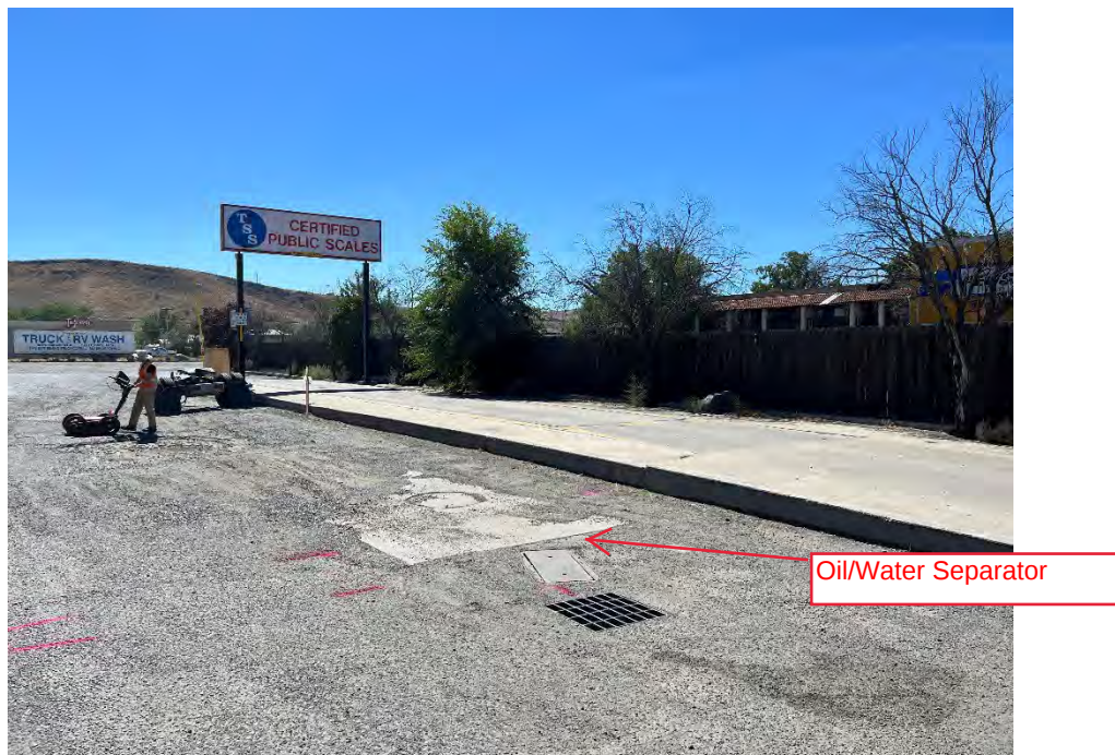
Photo 2. View of the truck scale, situated along the western property boundary. Pacific Geophysics is visible in the background scanning for and marking subsurface utilities that could act as preferential pathways. The oil/water separator is visible in the foreground.
