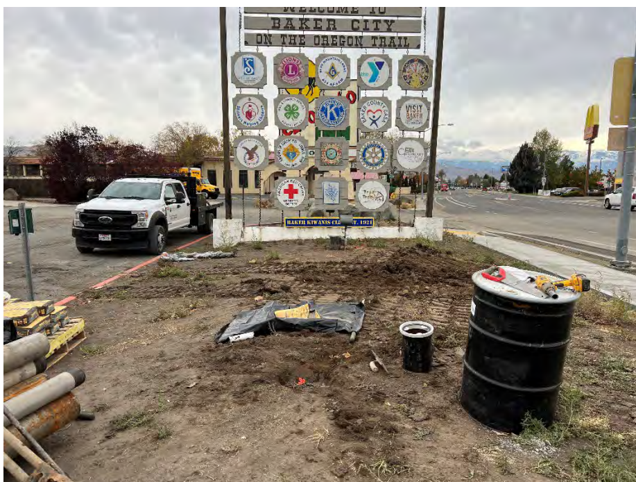
Photo 10. Monitoring well MW-10 being installed near the northern property boundary.
