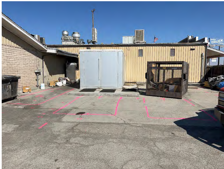
Photo 6. The decommissioned USTs marked out in pink paint from the geophysical survey are visible immediately south of the restaurant and east of the trucker lounge and employee offices.
