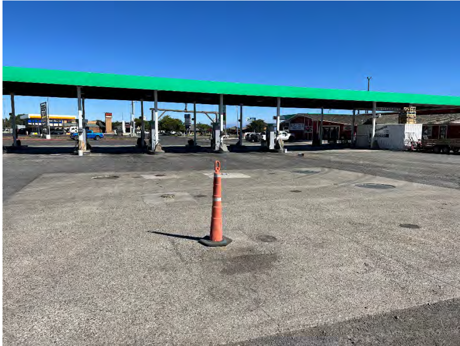
Photo 7. Looking north toward the three active USTs, with the semi-truck fueling station in the background.
