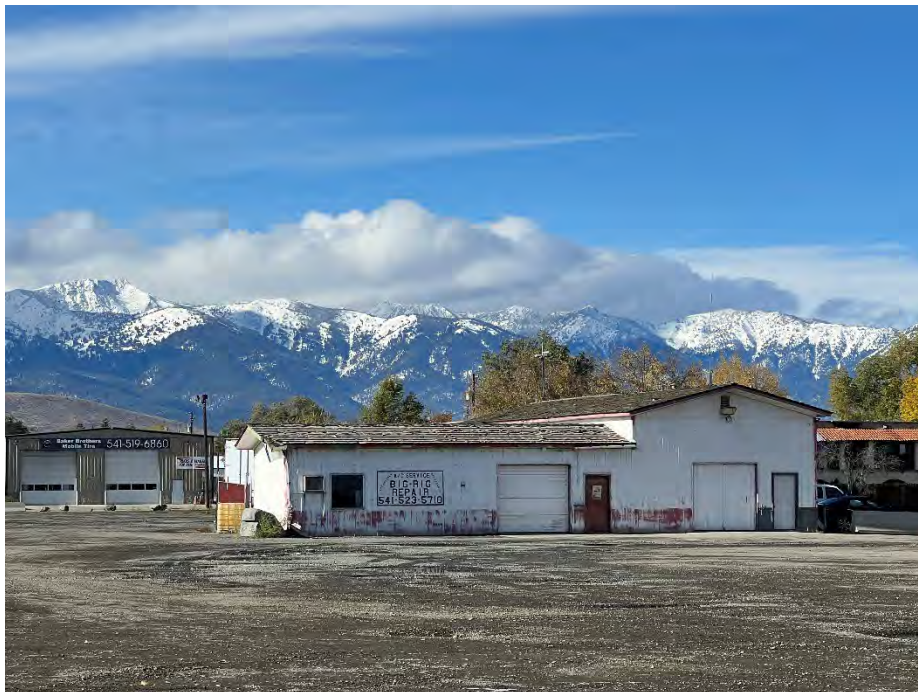
Photo 8. Looking west toward the former tire shop garage, which is now only utilized for storage.
