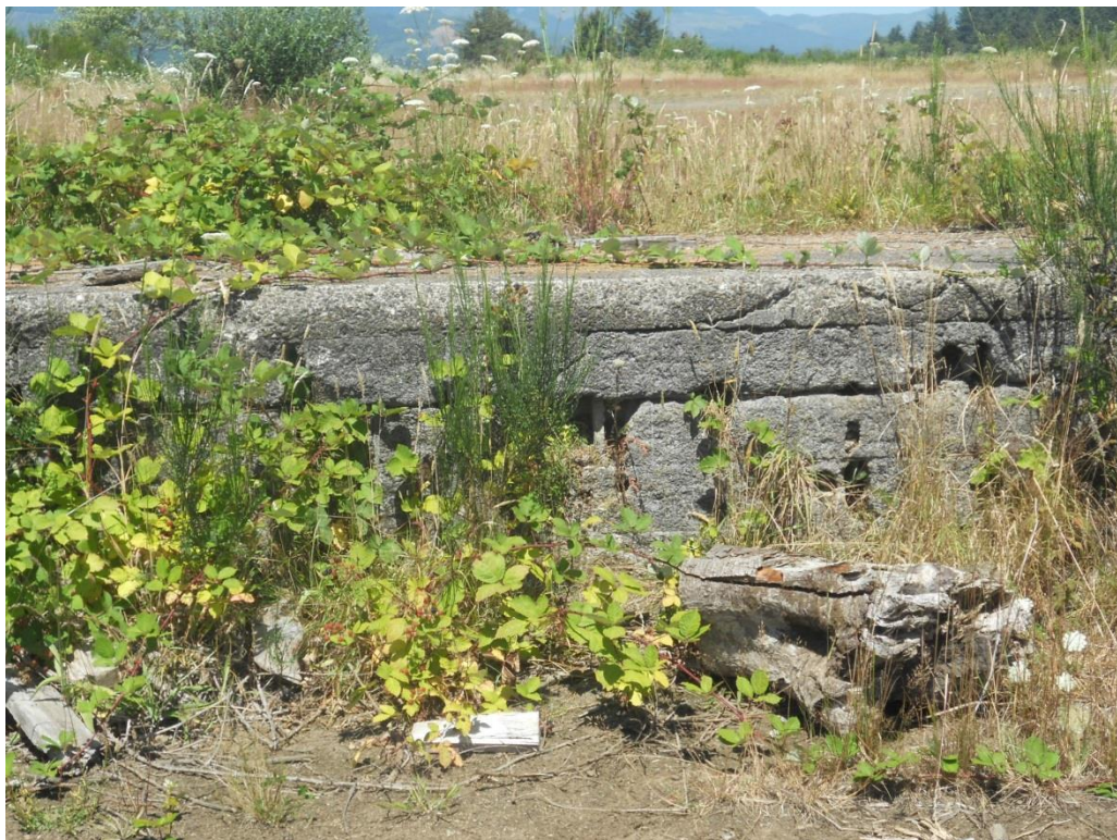
Photo 4. 3-foot concrete wall on concrete slab, facing north.
