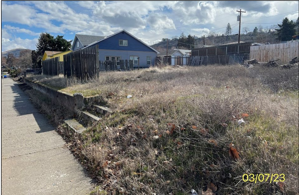
Photo 2: Current conditions of the subject property, taken from the northwest corner along East 12 th Street (facing southeast), with the existing retaining wall (photo left) .
