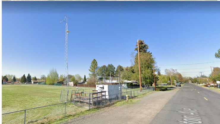
Klamath Falls KFP Air Monitoring Station.
