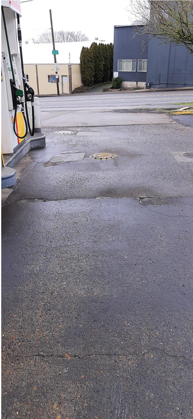
3: Diesel and regular tank nest looking North
