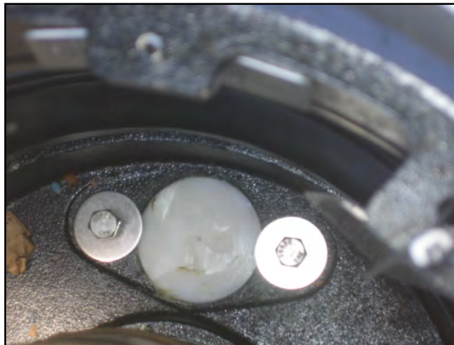
Figure 1-4 1DP-2100 Field Installed Drain Plug
