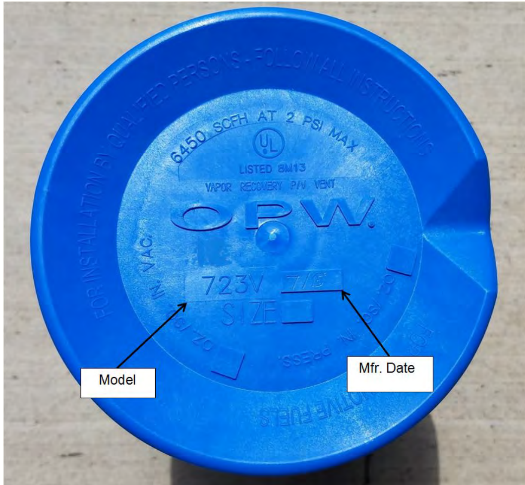
OPW Model 723V P/V Vent Valve
