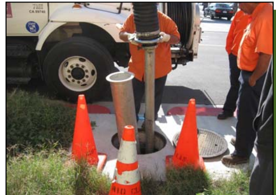
Insertion of vacuum hose into separation chamber.
