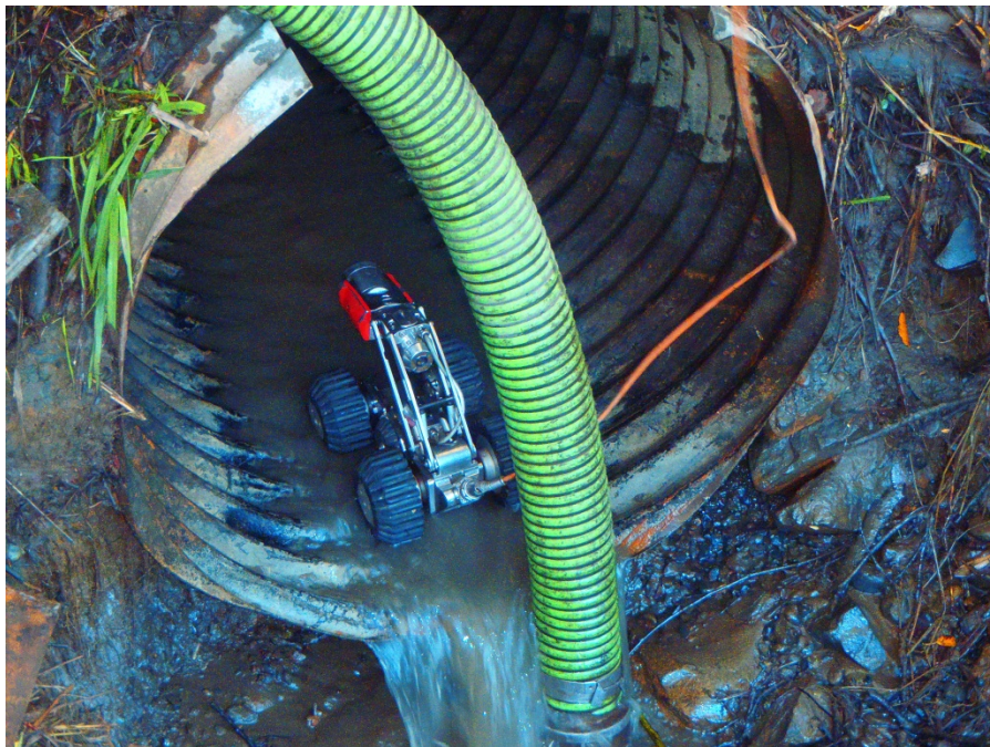
P-10: Remote controlled wheel camera unit enters the culvert to perform post cleanup inspection.
