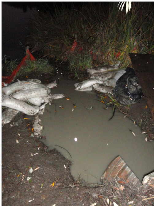
P-6: Highly turbid water observed entering Johnson Lake during the clean out of the eastern portion of the culvert.
