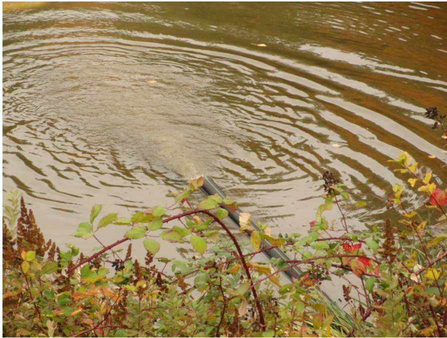
P-3: Water pump discharge from the storm water outfall into Johnson Lake.
