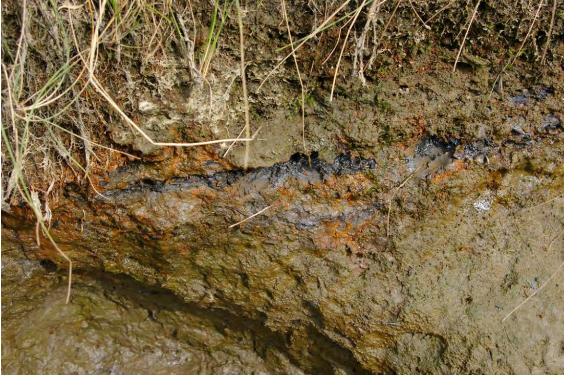
Photo 9 Close-up of seep showing contamination seam
