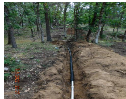
3" Shield pipe thru swale
