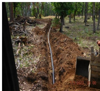
Effluent line continued
