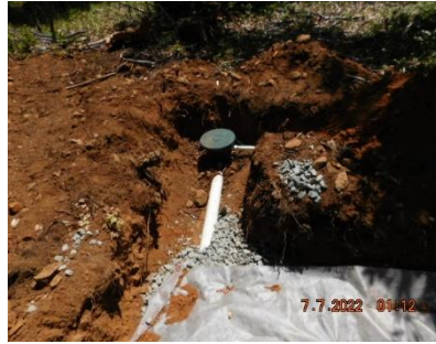
Effluent Line into Drop Box to Field
