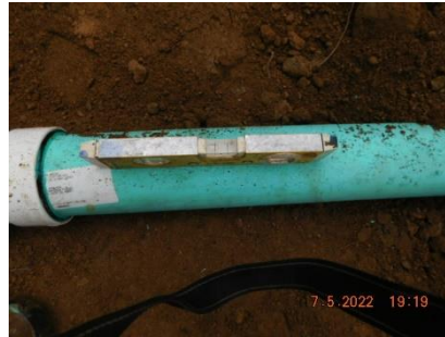
2% grade into tank
