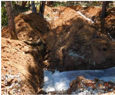
Top Line of Loop 1 – total 130 feet
