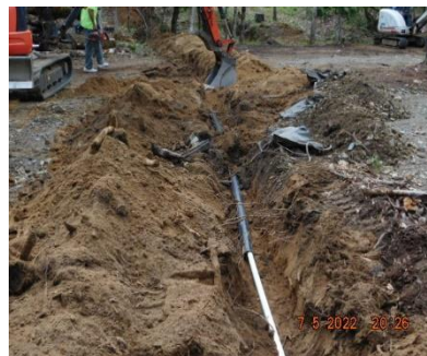
3" ABS Shield Pipe under driveway
