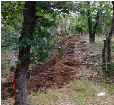
Effluent Line continued
