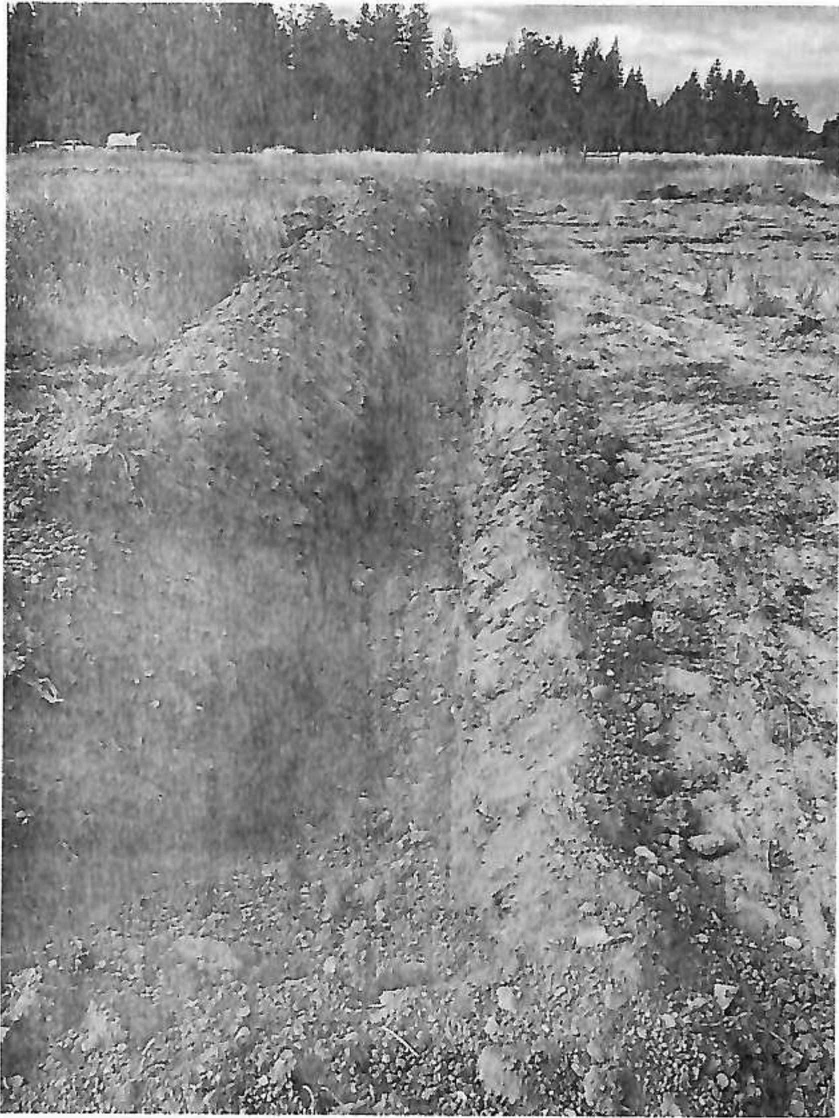
Trench before lay
