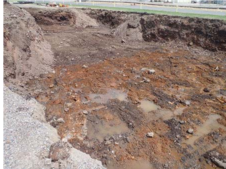
Photograph 14. . June 23, 2014 – Initial excavation of Phase 1 excavation area; central area looking southeast.
