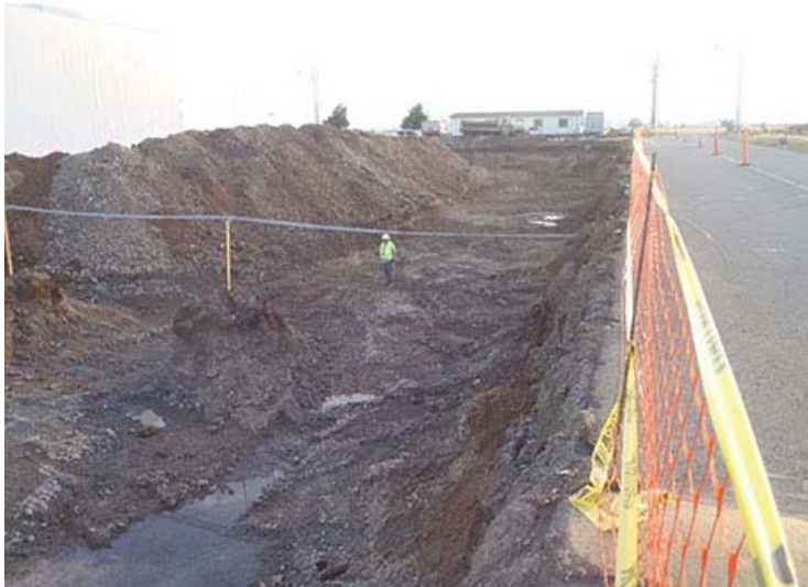
Photograph 21. June 31, 2014 – Final excavation of Phase 1 excavation area; looking east.
