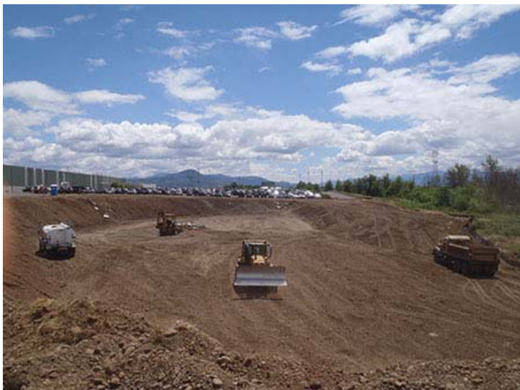
Photograph 5. May 28, 2014 – Whetstone fill area after grubbing; looking south.
