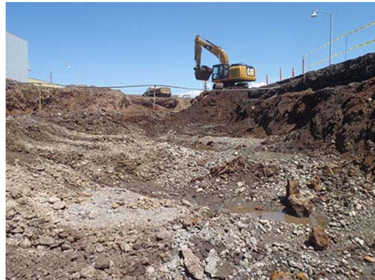
Photograph 16. June 28, 2014 – Further excavation of Phase 1 excavation area; looking east.
