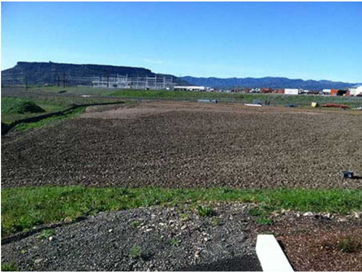
Photograph 41. March 18, 2015 – Completed expansion area parking lot; looking west at area just north of new parking lot.
