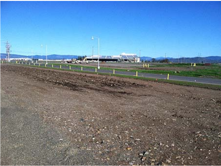
Photograph 42. March 18, 2015 – Phase 1 excavation area backfilled; looking southeast.
