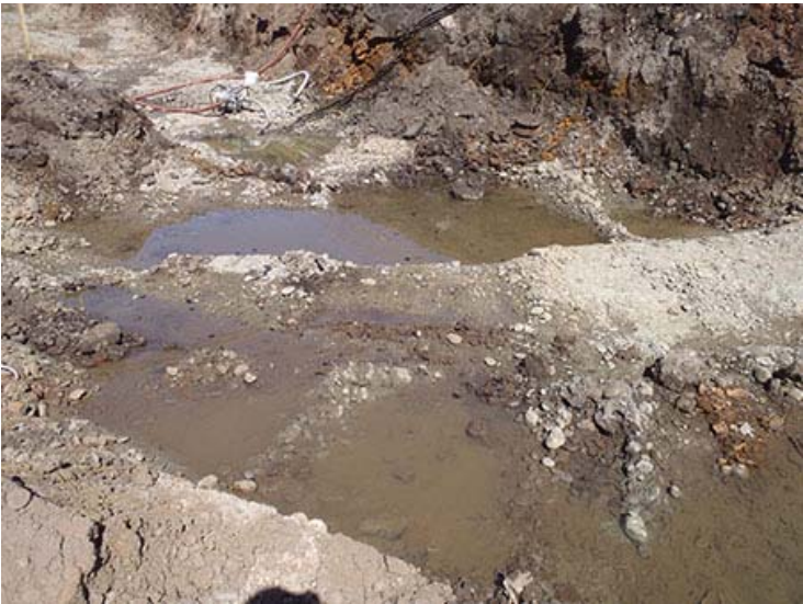
Photograph 18. June 29, 2014 – Further excavation of Phase 1 excavation area; central area looking at seep water.
