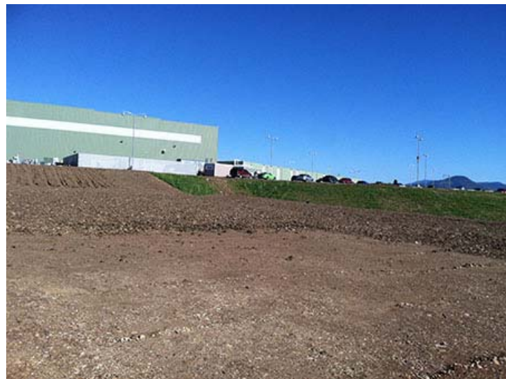
Photograph 40. March 18, 2015 – Area north of completed expansion area parking lot; looking east.
