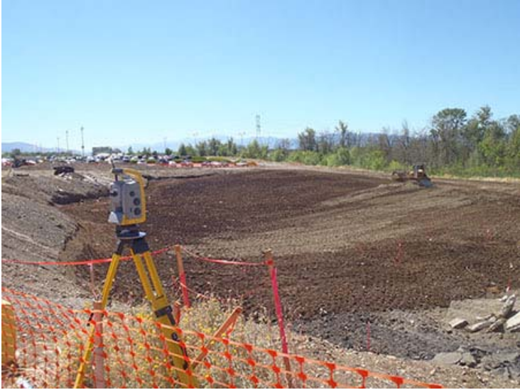
Photograph 27. June 23, 2014 – Whetstone landfill area placement of excavation filling; looking southwest.
