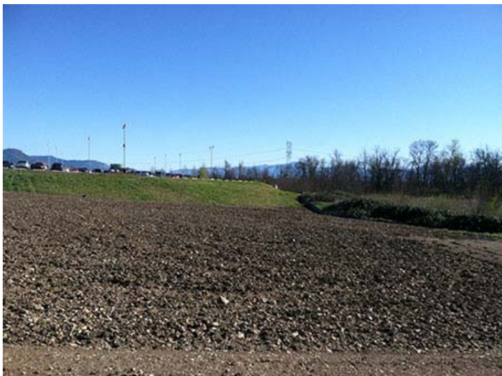
Photograph 39. March 18, 2015 – Area north of completed expansion area parking lot; looking south.
