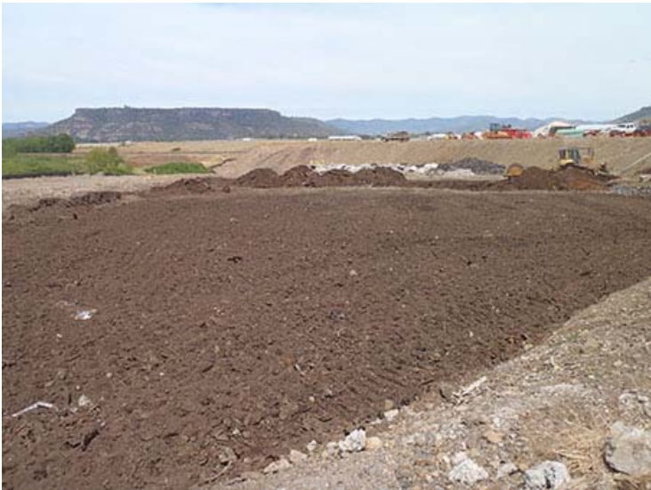
Photograph 25. June 22, 2014 – Whetstone landfill area placement of excavation filling; looking southwest.
