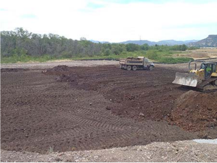
Photograph 28. June 28, 2014 – Whetstone landfill area placement of excavation filling; looking northwest.
