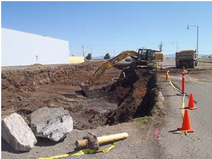
Photograph 15. June 28, 2014 – Further excavation of Phase 1 excavation area; looking east.
