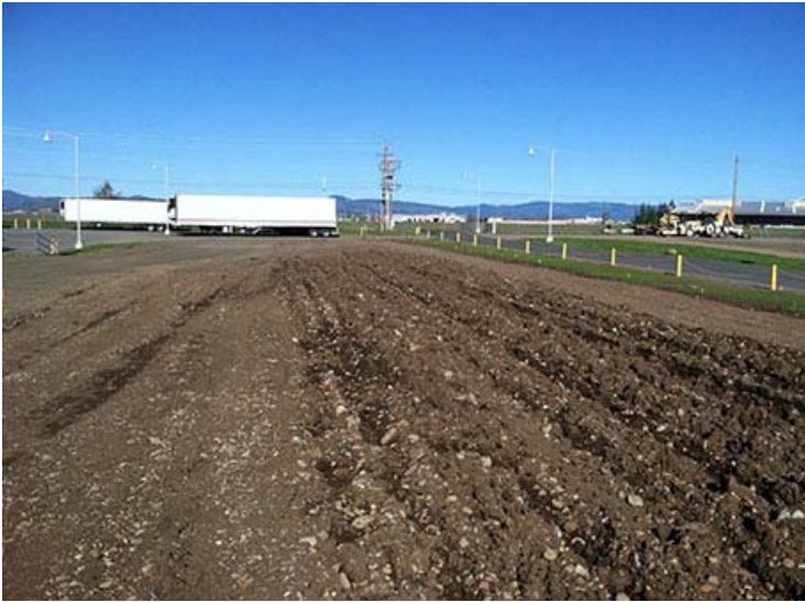
Photograph 43. March 18, 2015 – Phase 1 excavation area backfilled; looking east.
