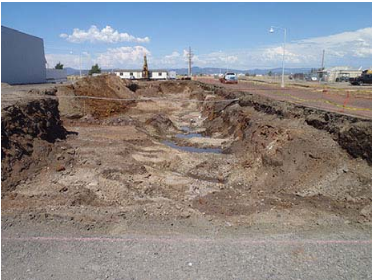
Photograph 17. June 29, 2014 – Further excavation of Phase 1 excavation area; looking east.
