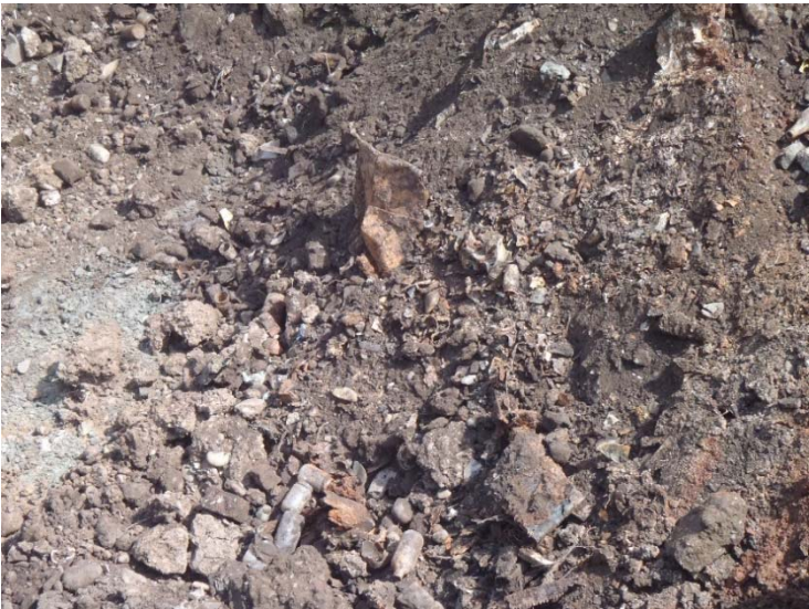
Photograph 10. June 22, 2014 – Excavation western area of Phase 1 excavation area; waste debris – metal and glass.
