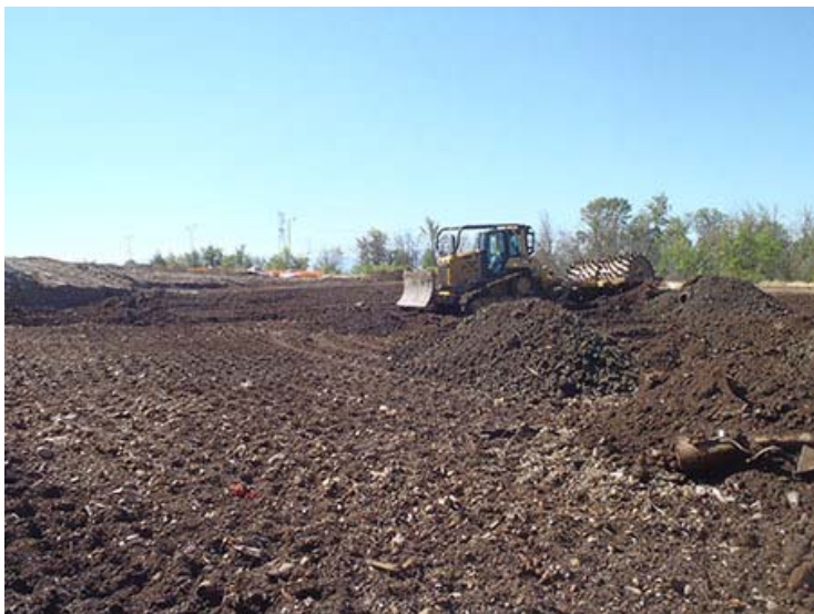
Photograph 29. June 29, 2014 – Whetstone landfill area placement of excavation filling; looking southwest.
