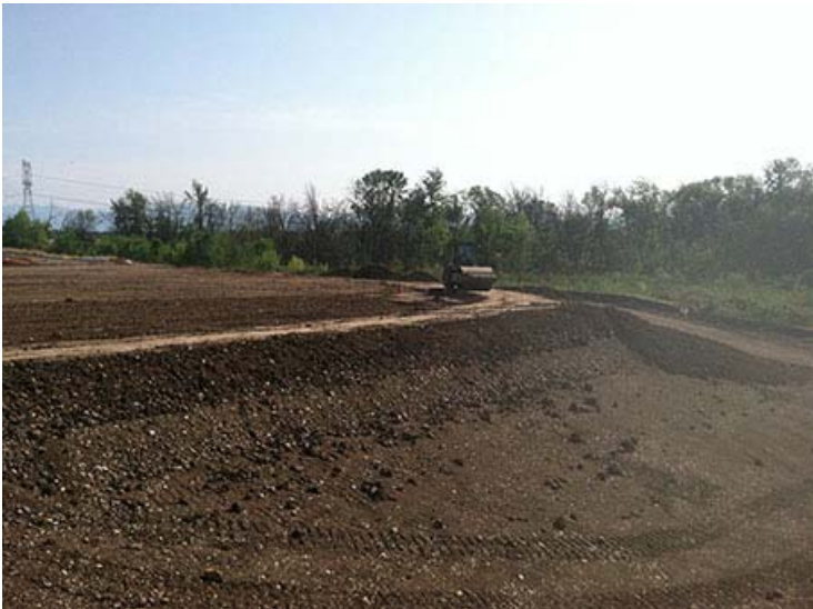
Photograph 33. June 31, 2014 – Whetstone landfill area placement of excavation filling; looking southwest.
