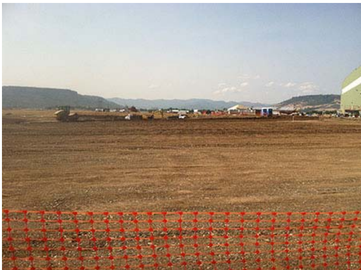
Photograph 31. June 31, 2014 – Whetstone landfill area placement of excavation filling; looking north.
