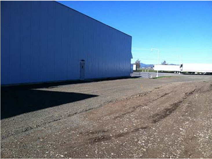
Photograph 44. March 18, 2015 – Phase 1 excavation area backfilled; looking northwest.
