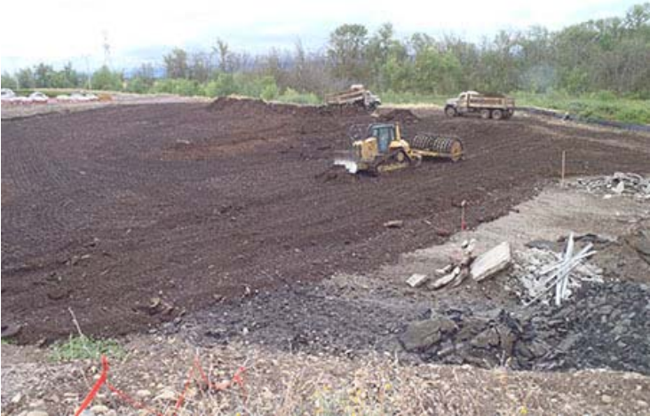
Photograph 26. June 23, 2014 – Whetstone landfill area placement of excavation filling; looking southwest.
