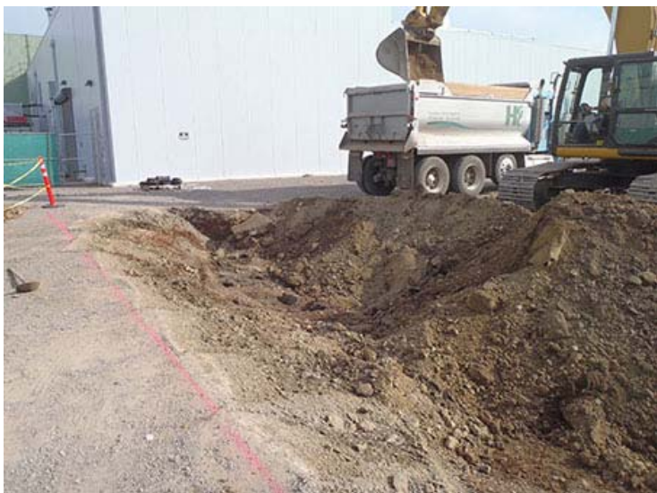
Photograph 7. June 22, 2014 – Initial excavation west end of Phase 1 excavation area.
