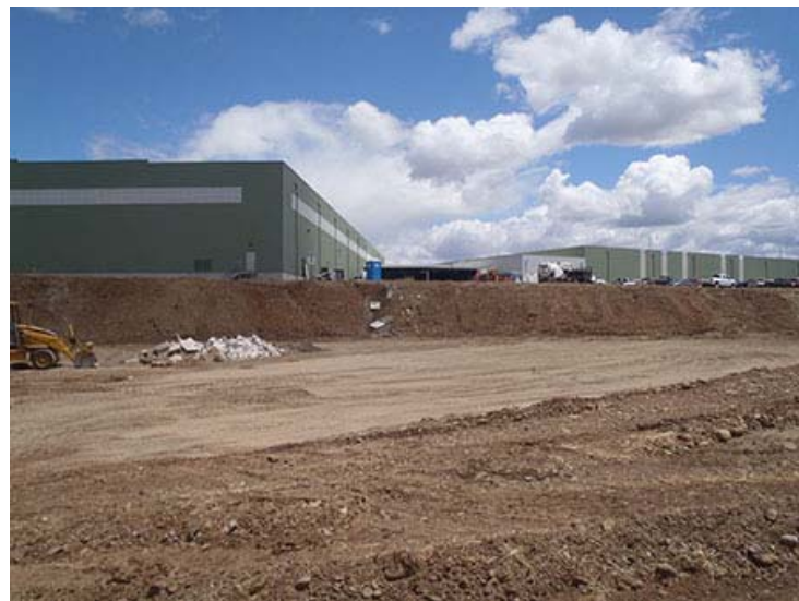
Photograph 6. May 28, 2014 – Whetstone fill area after grubbing; looking east.
