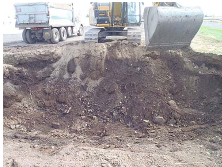
Photograph 8. June 22, 2014 – Initial excavation west end of Phase 1 excavation area; waste exposed.
