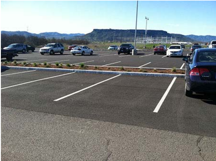
Photograph 36. March 18, 2015 – Completed expansion area parking lot; looking north at old and new parking lot asphalt line.
