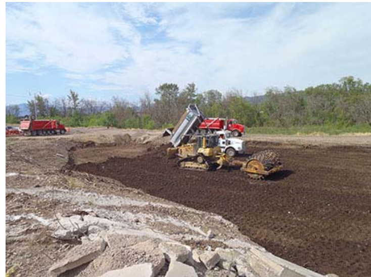
Photograph 24. June 22, 2014 – Whetstone landfill area placement of excavation filling; looking southwest.
