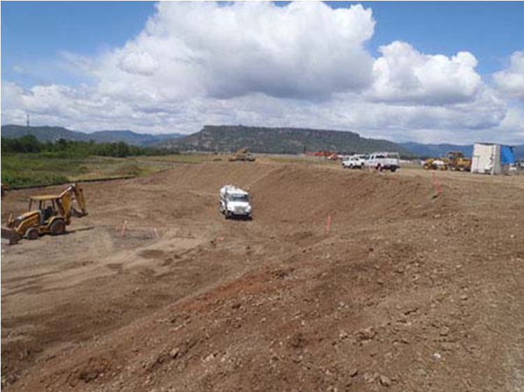
Photograph 4. May 28, 2014 – Whetstone fill area after grubbing; looking north.
