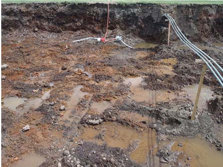
Photograph 13. June 23, 2014 – Initial excavation of Phase 1 excavation area; central area looking south.
