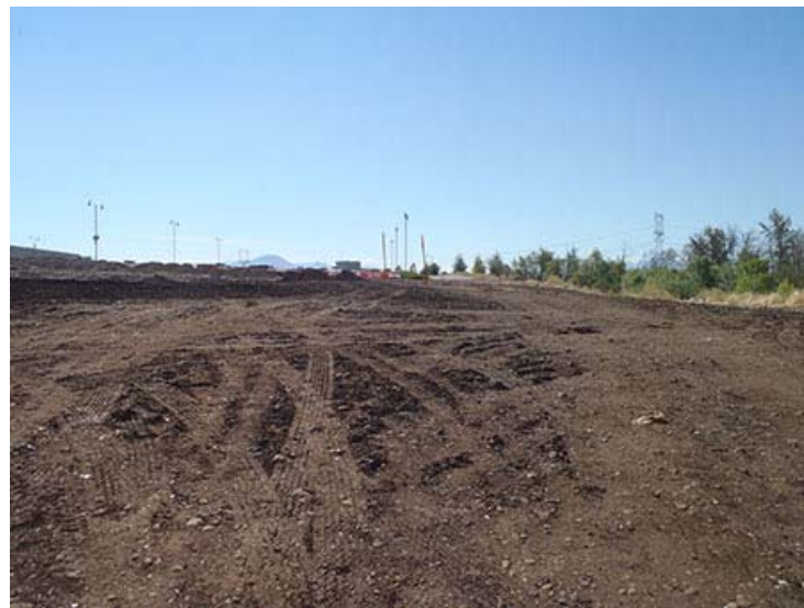
Photograph 30. June 30, 2014 – Whetstone landfill area placement of excavation filling; looking south.
