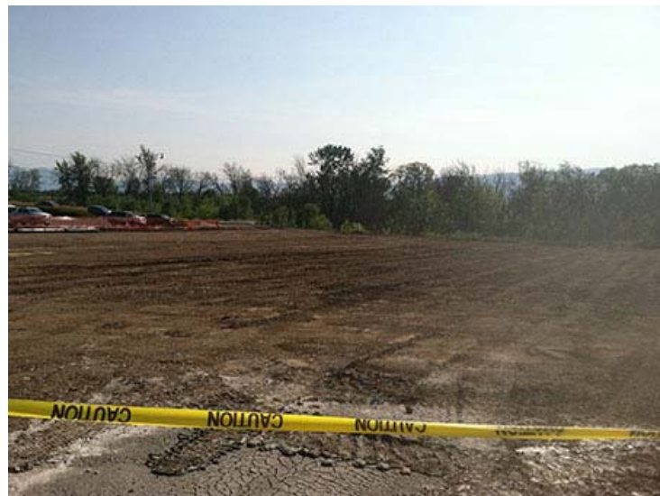
Photograph 32. June 31, 2014 – Whetstone landfill area placement of excavation filling; looking southwest.
