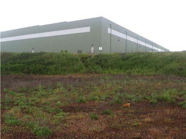
Photograph 2. May 8, 2014 – Whetstone fill area prior to site work; looking east.
