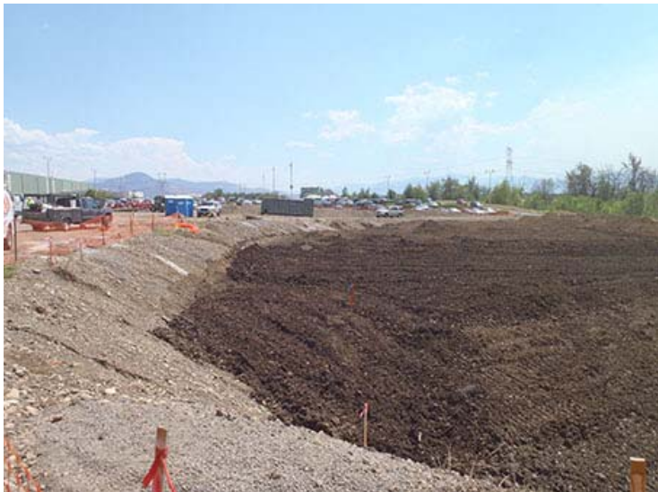
Photograph 23. June 22, 2014 – Whetstone landfill area placement of excavation filling; looking south.
