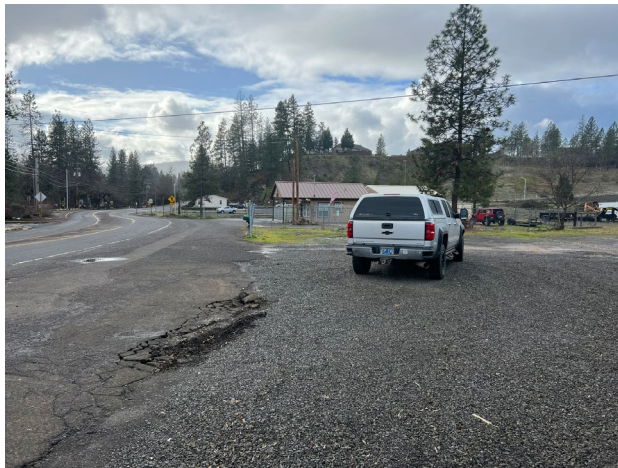
2. The Subject Property and Neighboring Properties – view to the west, truck parked on former UST pit.
