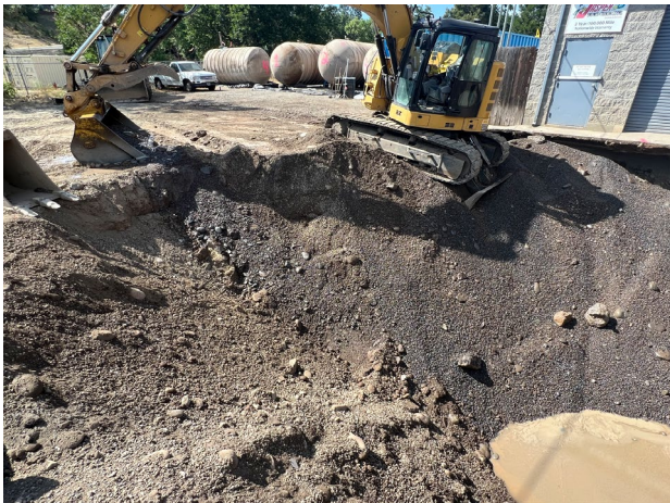
14. The Subject Property – Decommissioning by removal.
