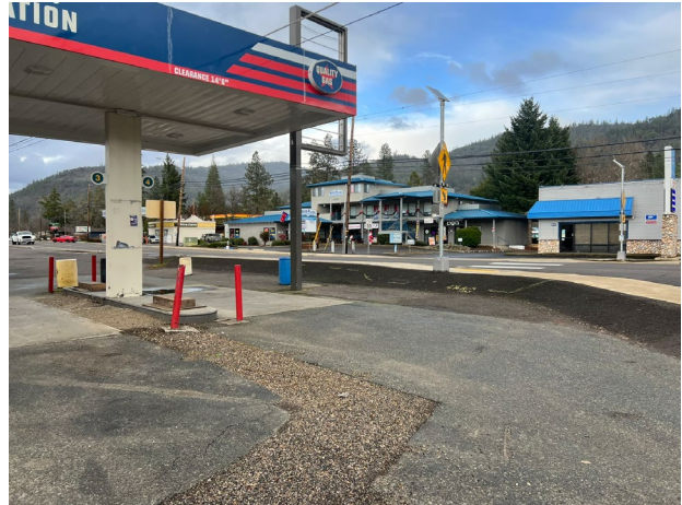
4. The Subject Property and Neighboring Properties – view to the southeast, canopy and former dispenser island.
