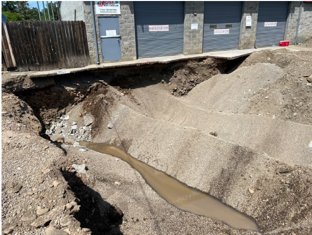
13. The Subject Property – Decommissioning by removal.
