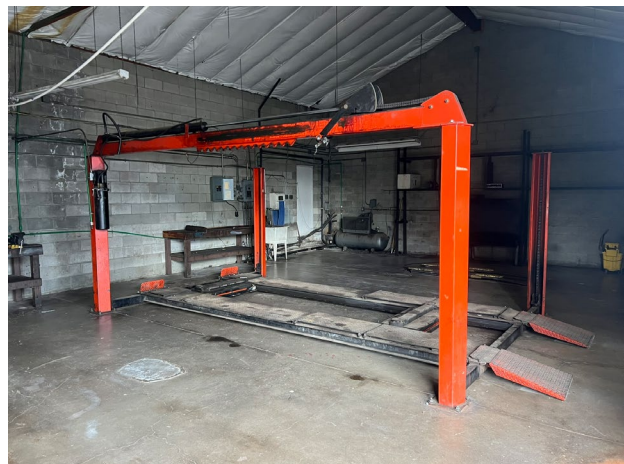
6. The Subject Property – former garage shop interior, above-ground hoist.
