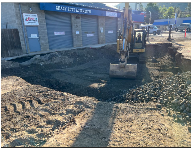
15. The Subject Property – Backfill and compaction.
