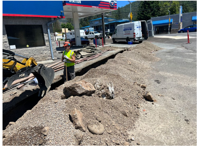
16. The Subject Property – Piping Trench.
