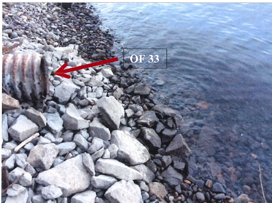
Outfall 33 Photo from Shoreline – June 13, 2018
