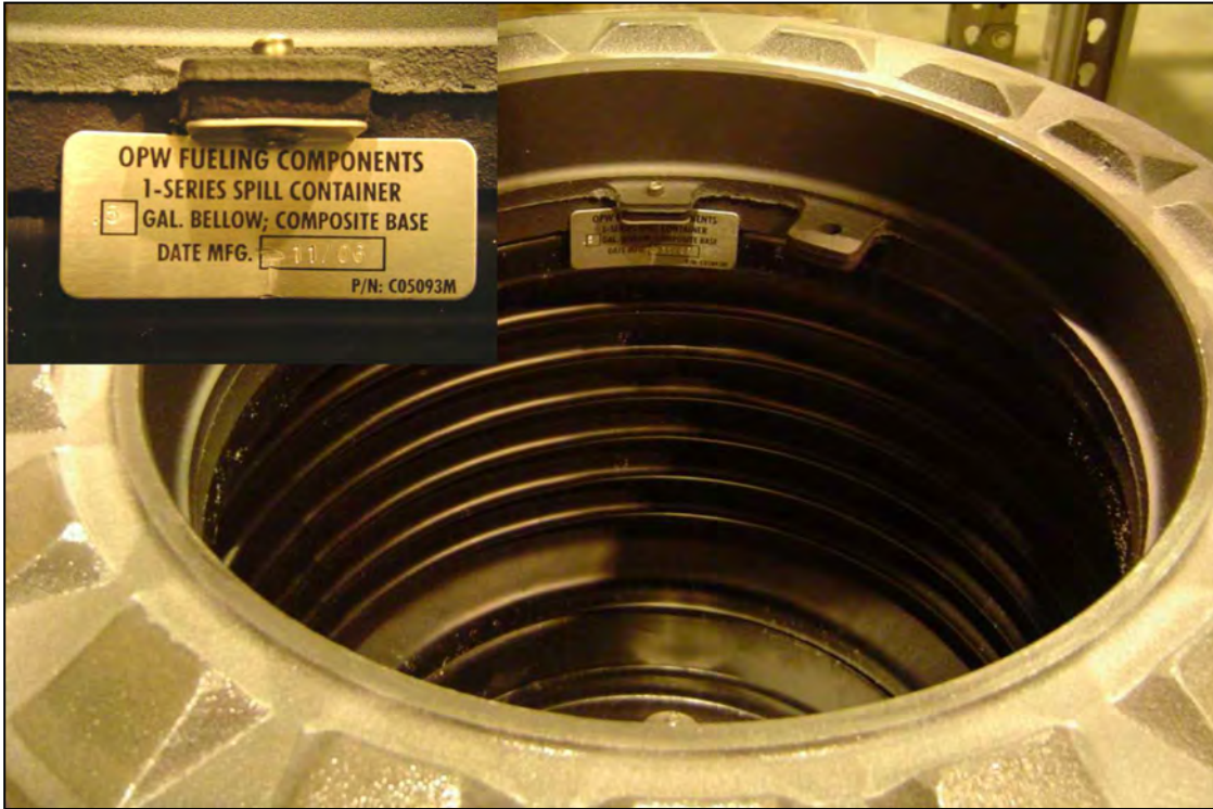
Figure 1-1 Direct Bury Spill Container OPW 1-Series (GAS/E85)
