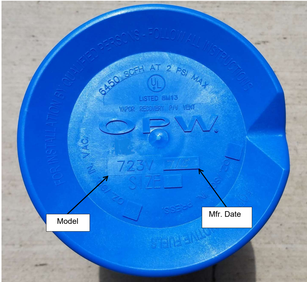
OPW Model 723V Pressure/Vacuum Vent Valve
