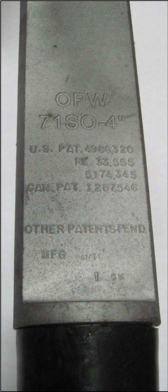
Figure 1-26 OPW 71SOM-412C Overfill Prevention Device
