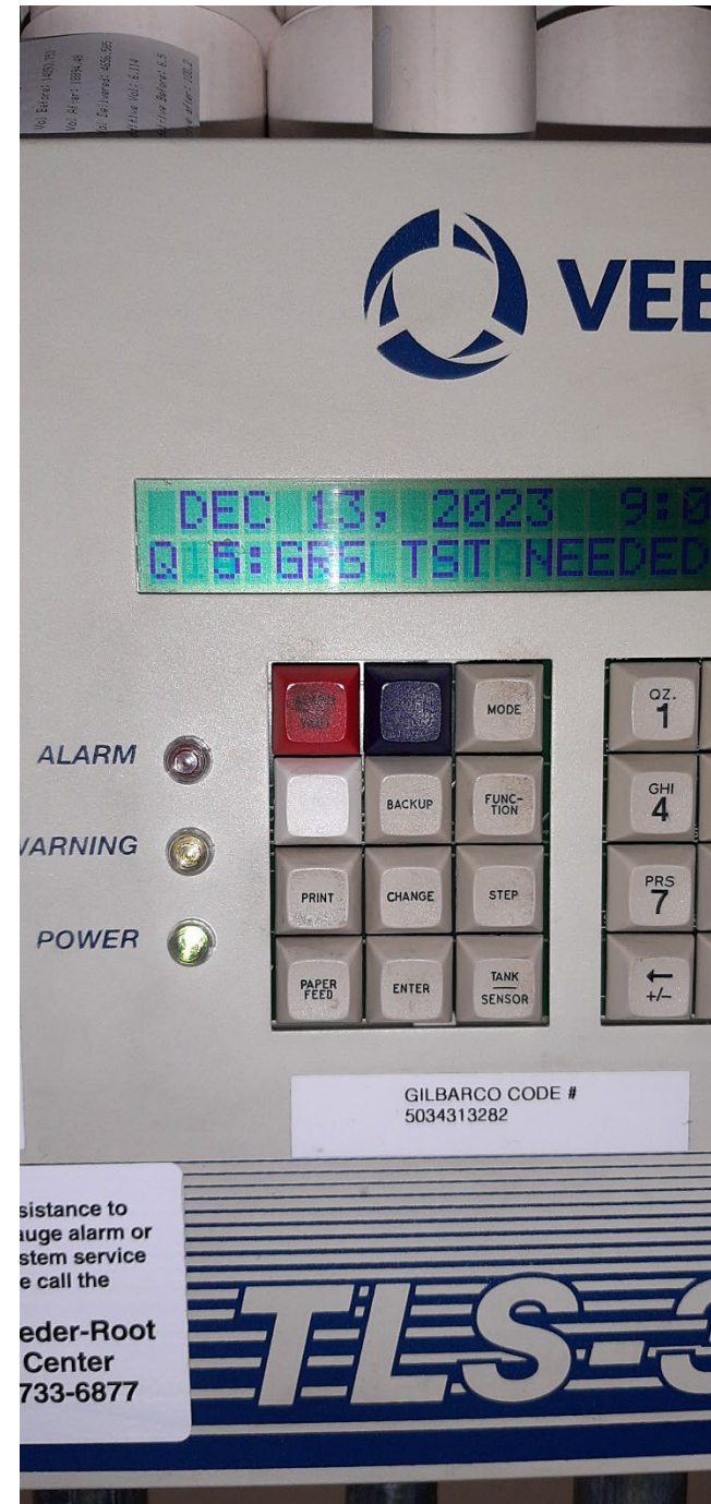
21: GRS Alarm on Q5 Ultrazol tank
