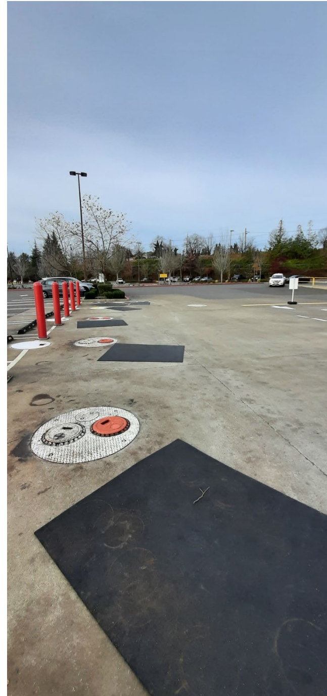
2: Tank nest looking West
