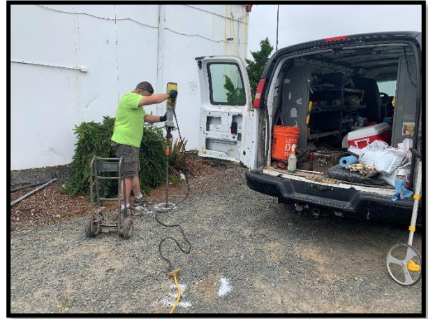
PHOTOGRAPH NO. 2 – Drilling Boring B1.
