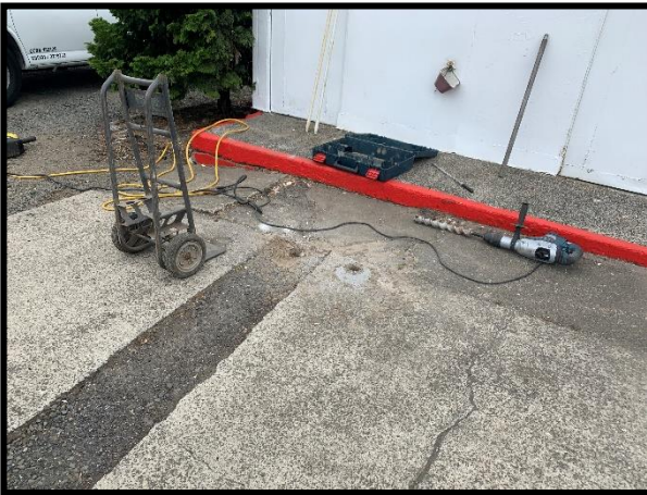
PHOTOGRAPH NO. 3 – Refusal in two attempts at proposed location of Boring B3.
