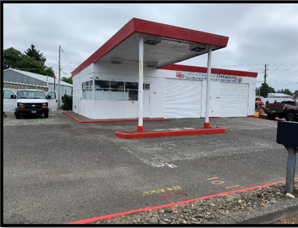
PHOTOGRAPH NO. 1 – Front view of building.
