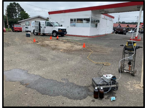
PHOTOGRAPH NO. 6 – Groundwater sampling in Boring B5.
