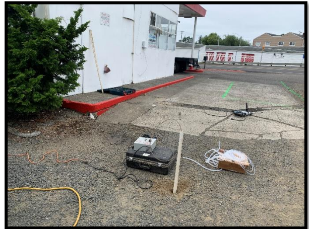
PHOTOGRAPH NO. 4 – Groundwater sampling in final location of Boring B3.
