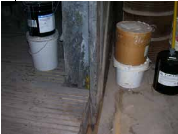
Close-up of the break in the floor between silvering room (left) and the rest of the building.
