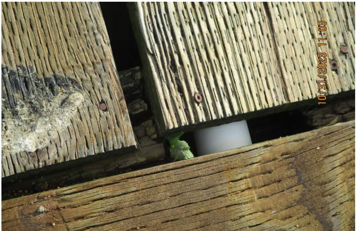
Photo 14: Example of cut stringer to allow for water pipe to be installed below the deck.
