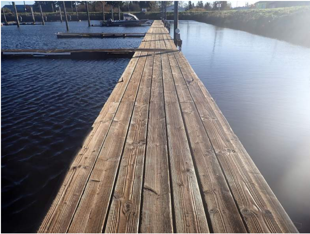
Photograph 7– Typical Main Floating Dock Condition
