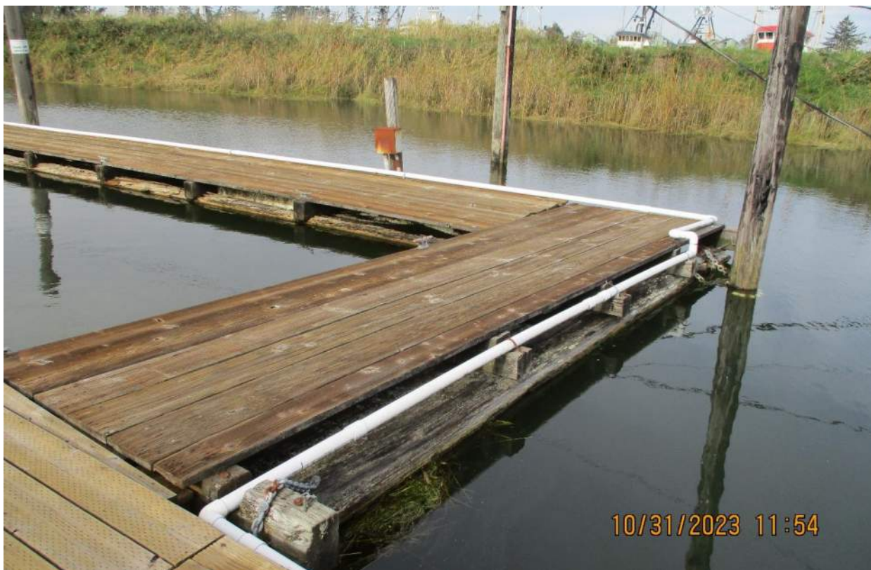
Photo 8: Corner where Dock M and N meet. Note the sag in the corner due to lack of float log buoyancy.
