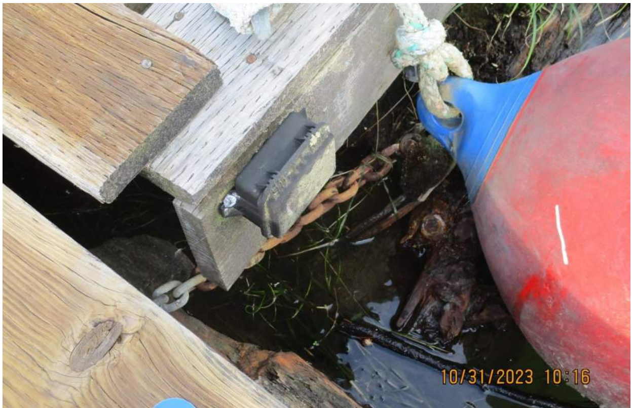
Photo 26: Decayed chain connect. Note corrosion in chain and heavily corroded hardware in float log.
