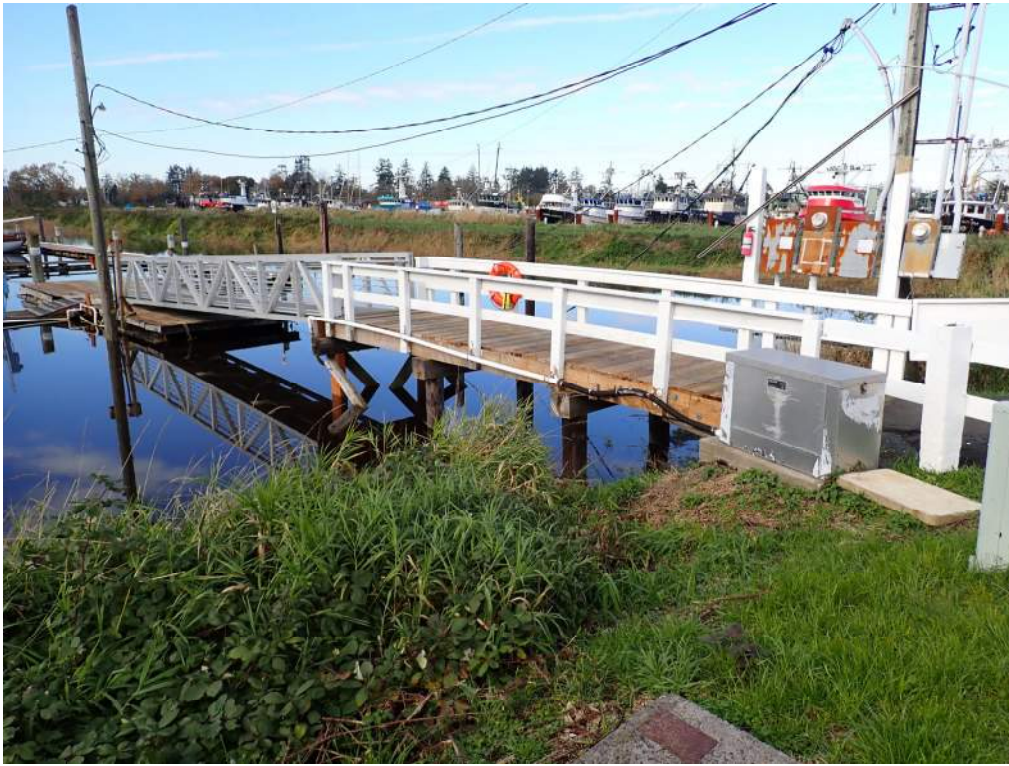
Photograph 3– Northeast Marina Entrance, Looking Northwest
