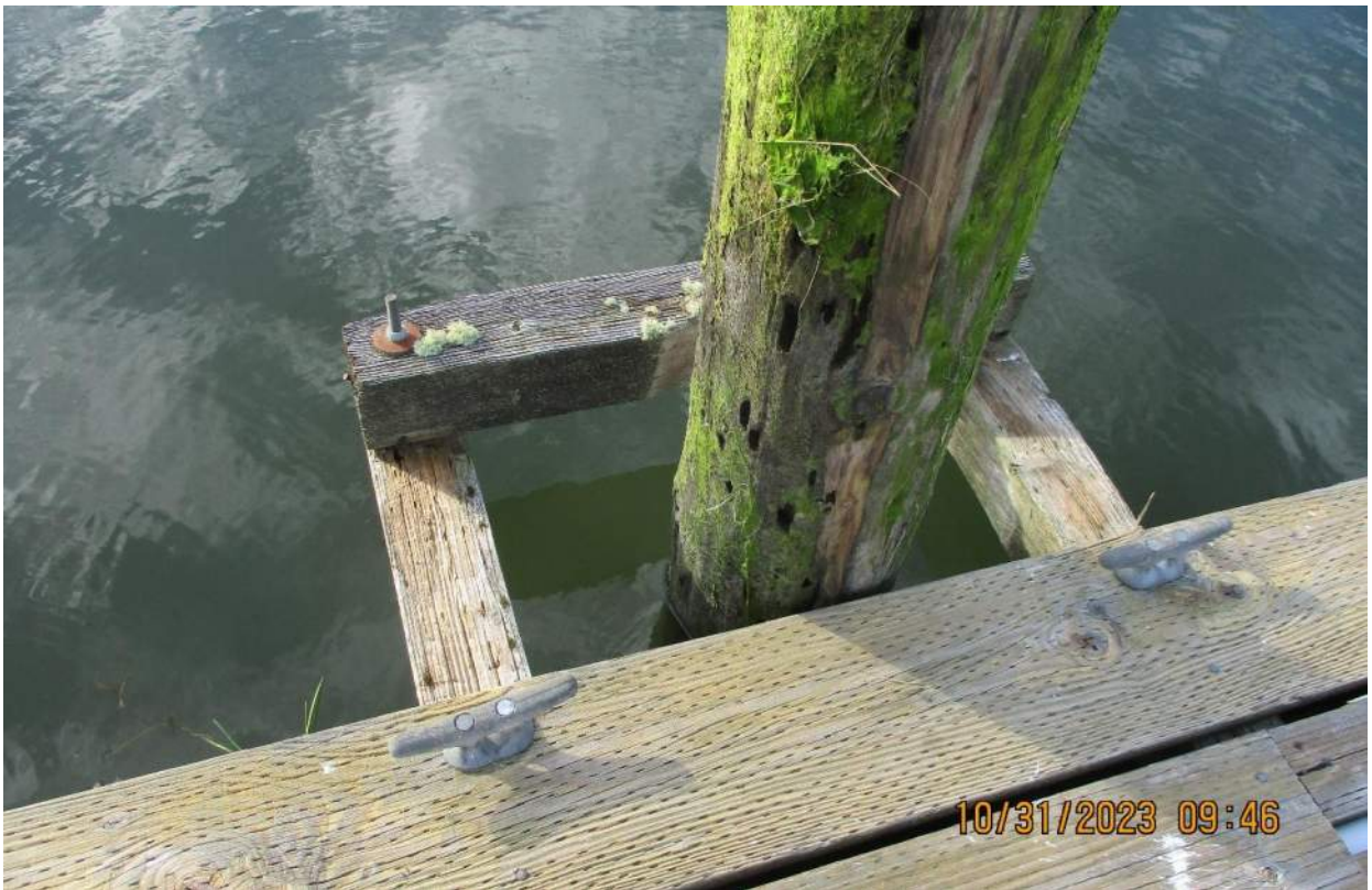
Photo 2: Close up showing possible marine borer activity.
