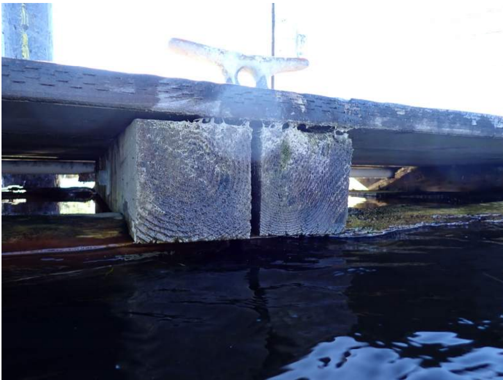
Photograph 16– Typical Transverse Timber Support
