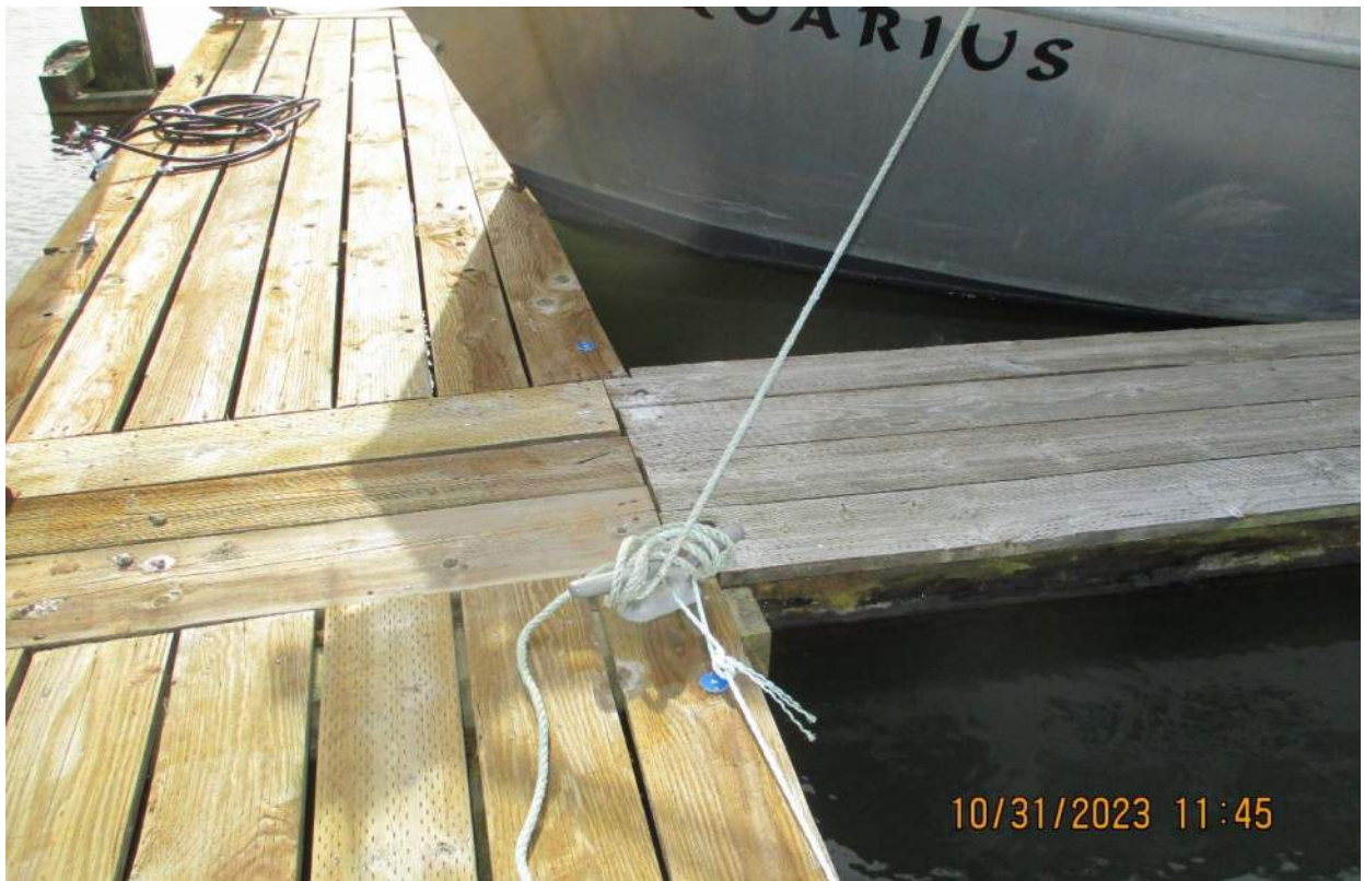
Photo 28: Ledger type connection where finger pier meets main walkway.
