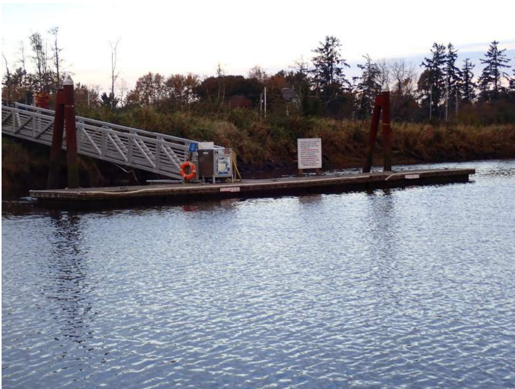
Photograph 6— Pump Out Dock, Looking Northwest
