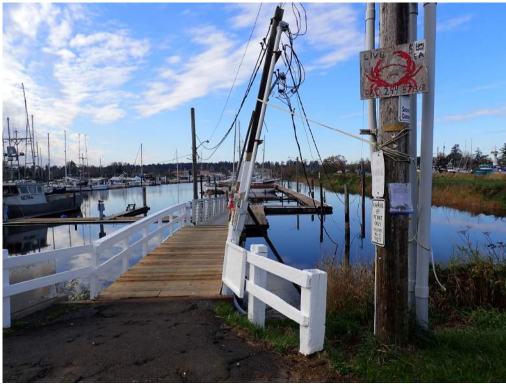
Photograph 17– Unstable Utility Line Post at Northeast Marina Entrance Looking West
