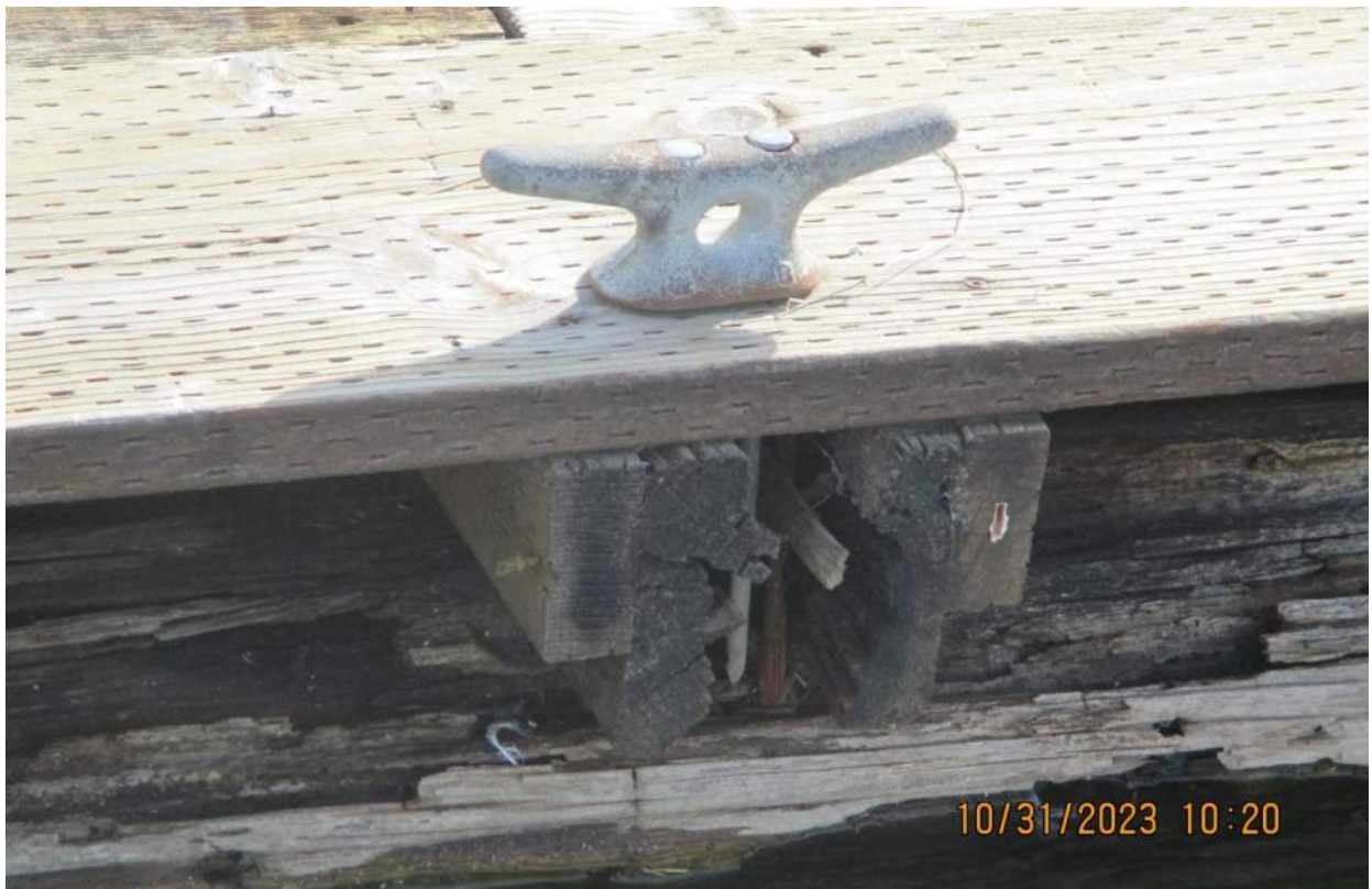
Photo 24: Typical condition of cleat. Cleat is only restrained by the deck, stringer below is decayed.
