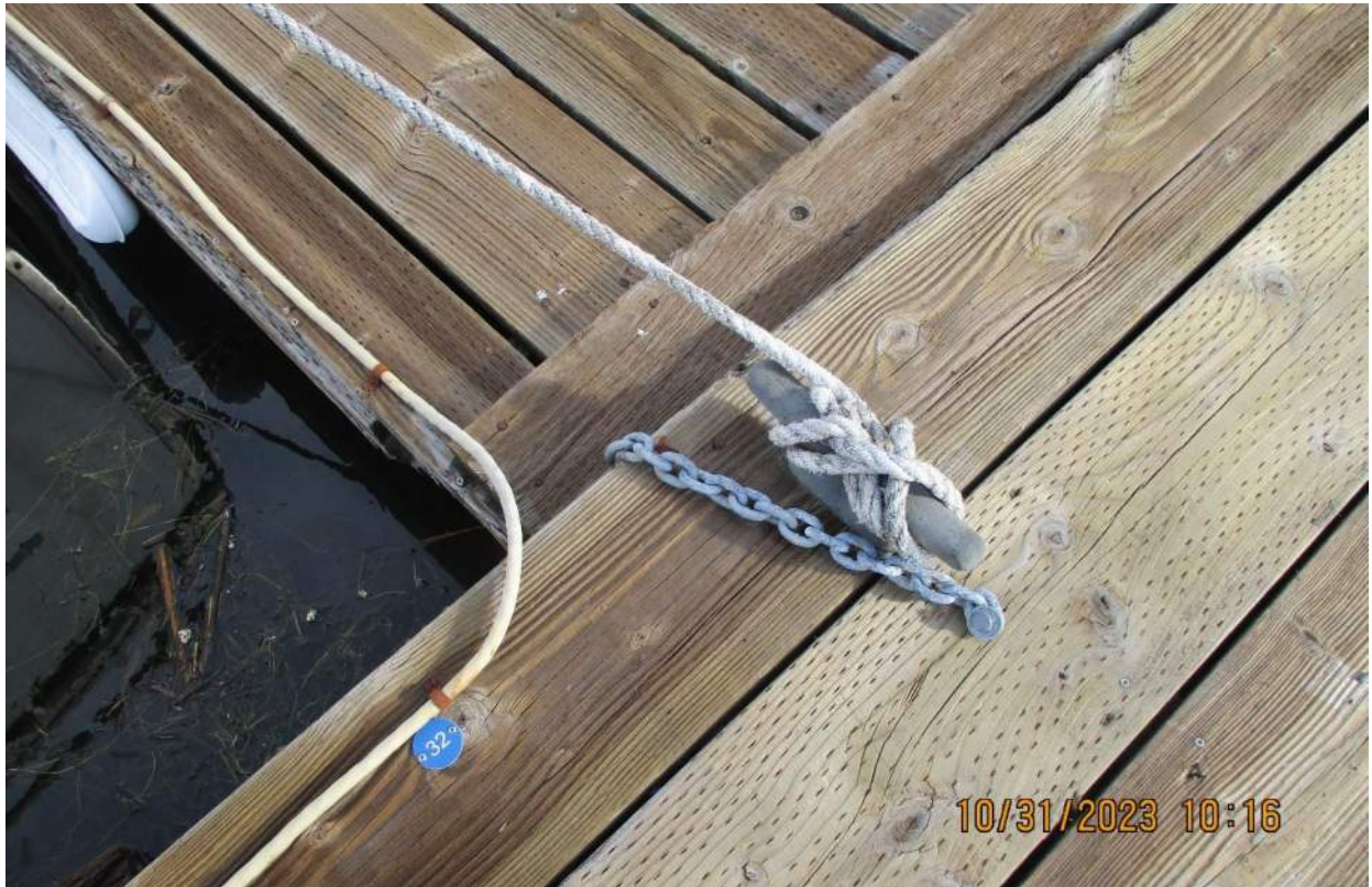
Photo 25: Chain connection, with lag bolt into the deck. Unclear if lag bolt is into stringer below.
