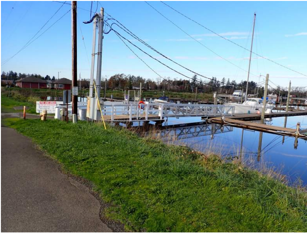
Photograph 5— Southwest Marina Entrance, Looking Northwest
