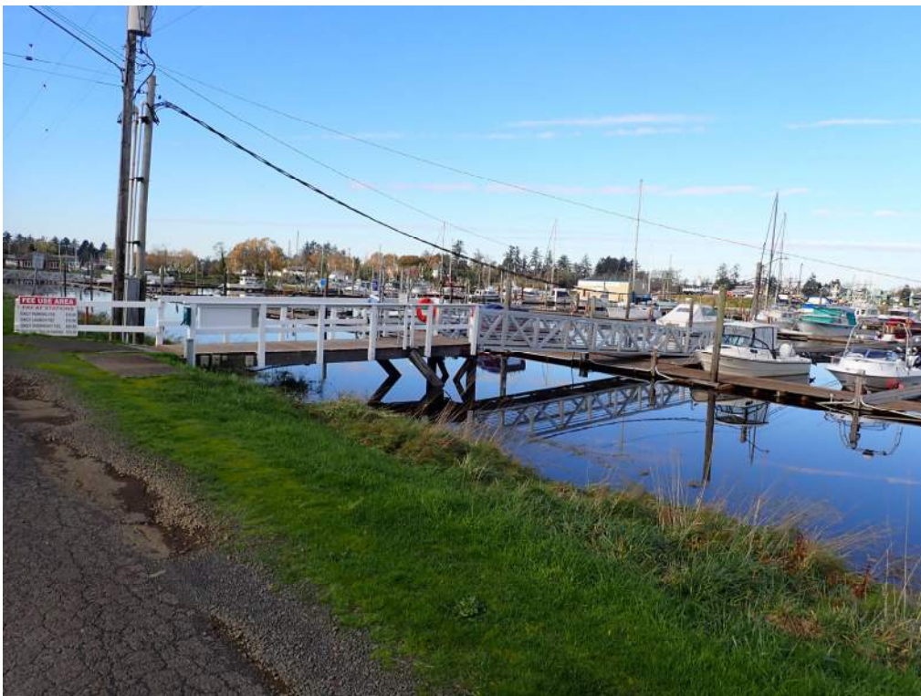
Photograph 4– Southeast Marina Entrance, Looking Northwest
