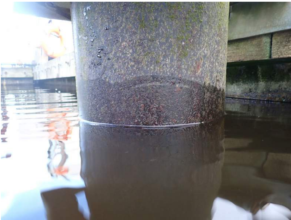
Photograph 12– Typical Steel Guide Pile at Waterline
