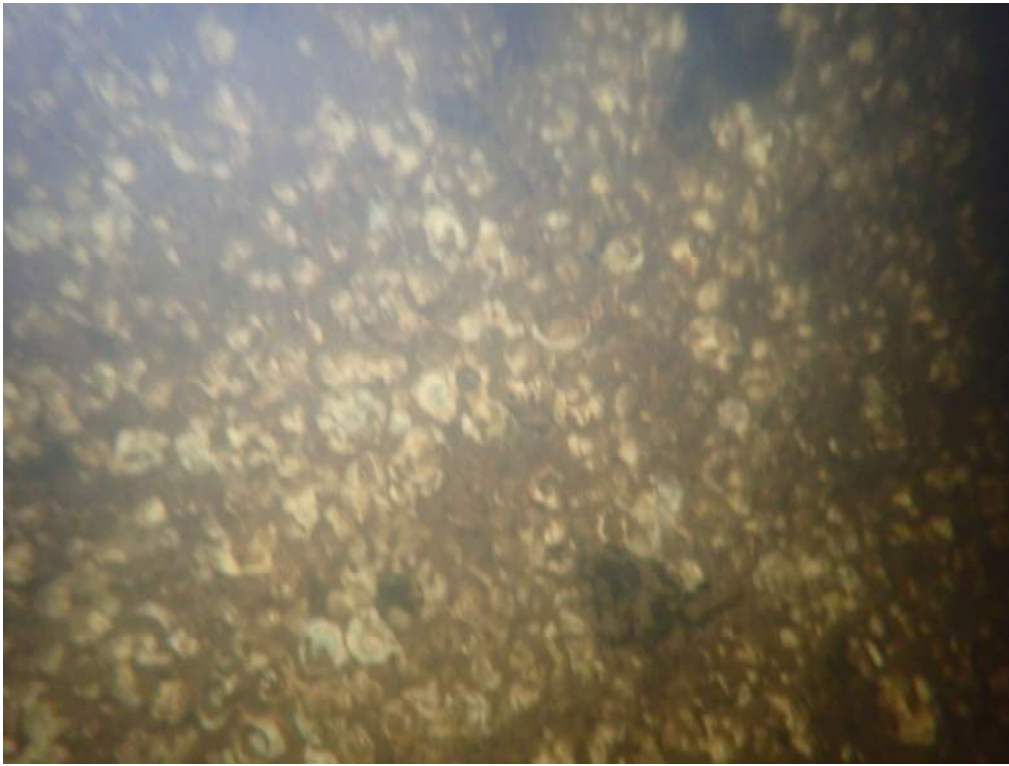
Photograph 13– Typical Marine Growth on Steel Guide Pile Underwater
