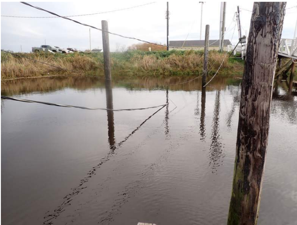
Photograph 32– Submerged Utility Line Near Northwest Marina Entrance
