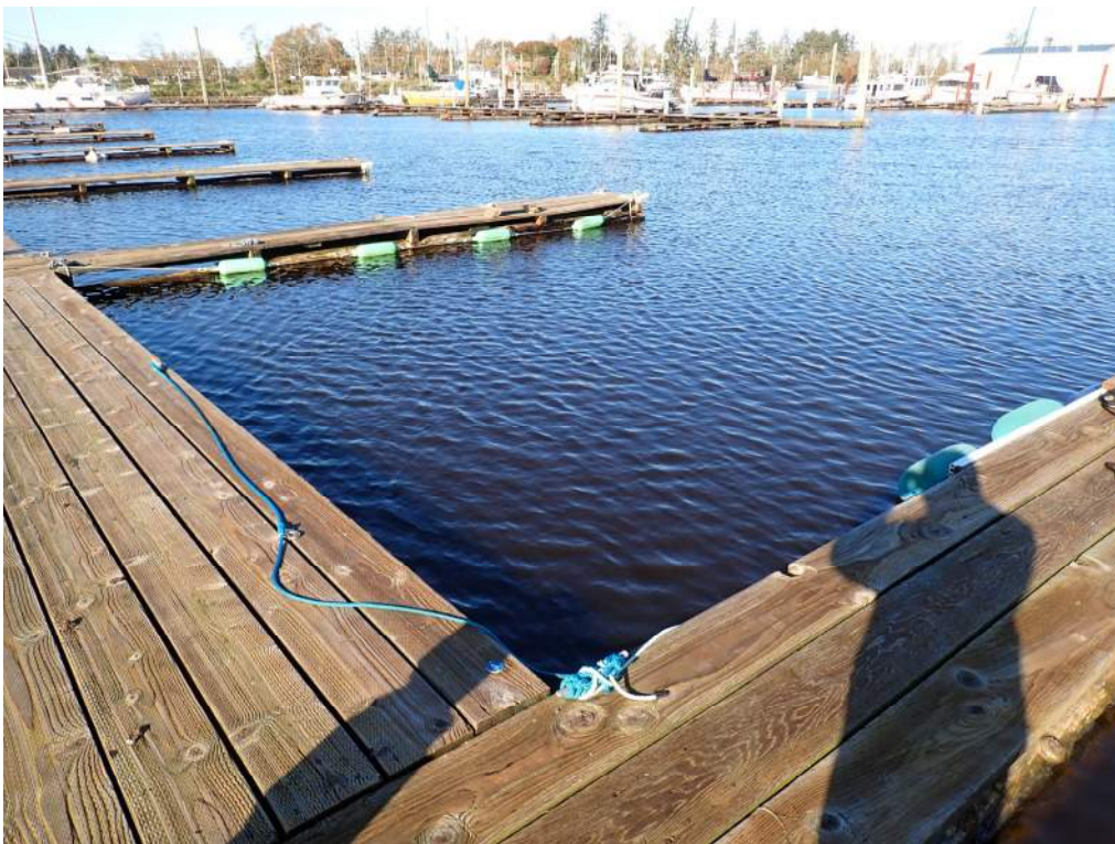
Photograph 8– Typical Finger Pier Condition
