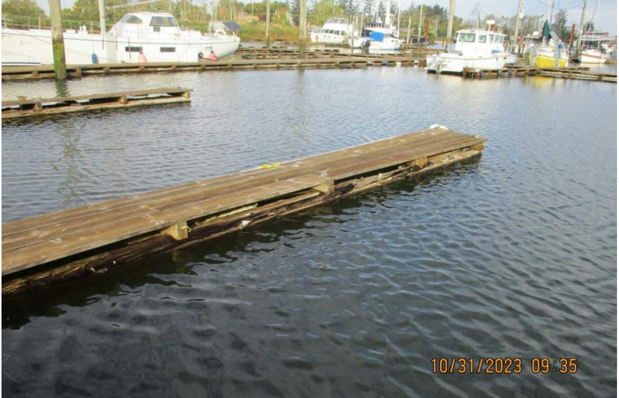
Photo 17: Typical condition of existing trestles. Note the decay in the timber piling.
