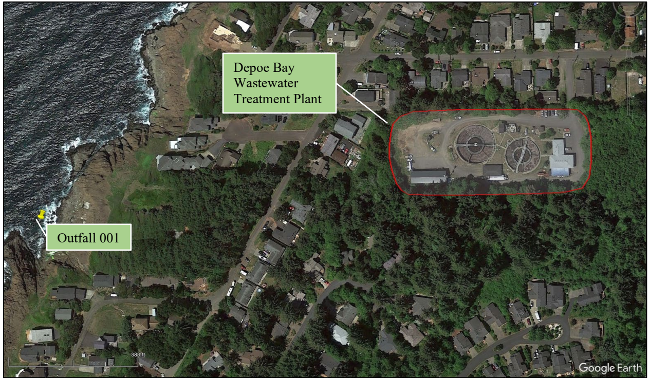
Figure 2-1: Aerial view of Depoe Bay Wastewater Treatment Plant and Outfall 001
