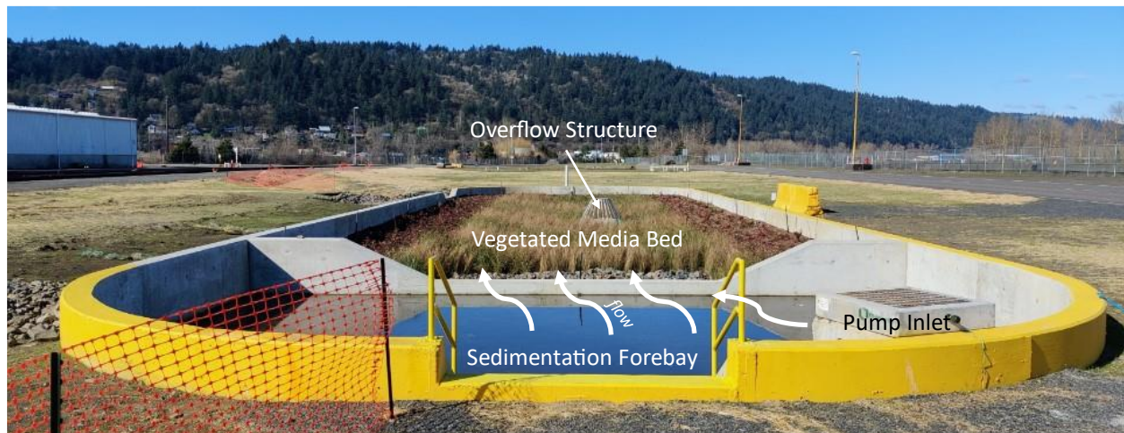
Figure 2: T4 Basin M Bioinfiltration Basin Overview
