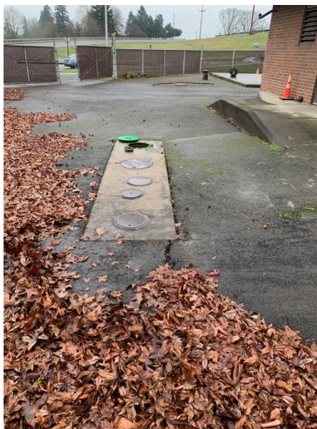
Photo 6. UST fill ports over UST. View is to the N.
