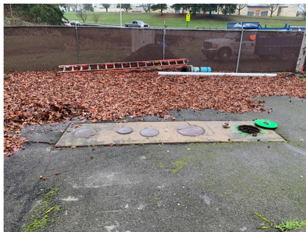
Photo 10. Location of the UST. View is to the NW.
