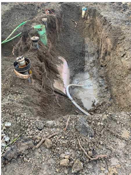
Photo 11. Exposed tank with groundwater in excavation. View is to the SW.
