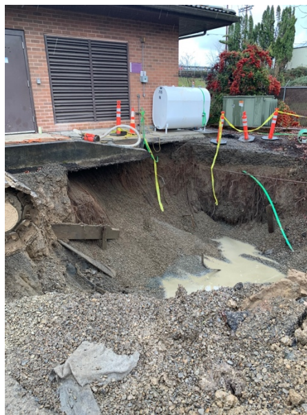
Photo 20. View of tank excavation pit with groundwater pumped out. View is to the SSE.
