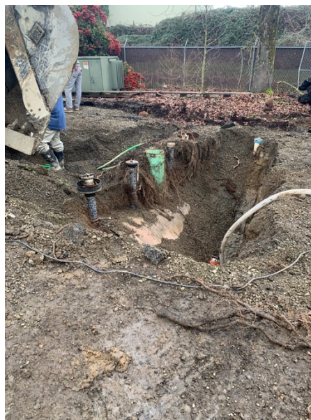
Photo 12. UST area view. View is to the S.
