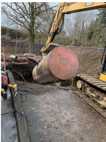
Photo 15. Removing the UST from the tank pit. View is to the SW.
