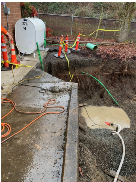
Photo 19. SE corner of excavation with groundwater pump in pit. View is to the SW.
