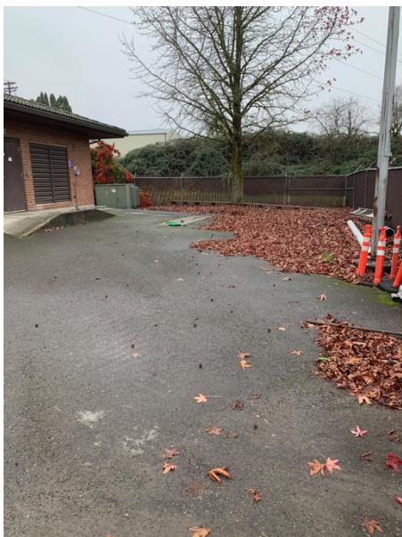
Photo 5. Asphalt parking lot covering UST. View is to the S.
