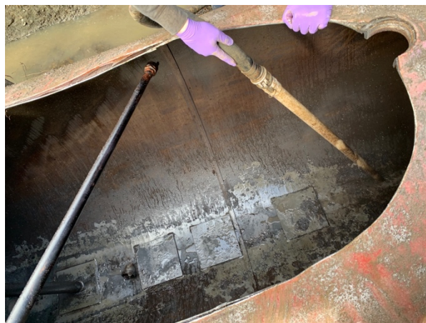
Photo 14. Triple-rinsing and pumping the interior of the tank.
