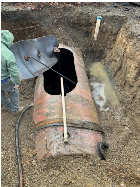
Photo 13. Cut tank top to inspect tank interior. View is to the SW.
