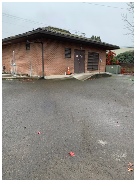
Photo 4. NW corner of pump station building. UST is located along right edge of photo. View is to the SE.
