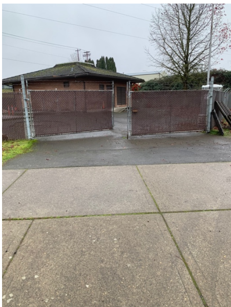
Photo 3. Gates securing the wastewater pump facility at 150 Newberg Highway.
