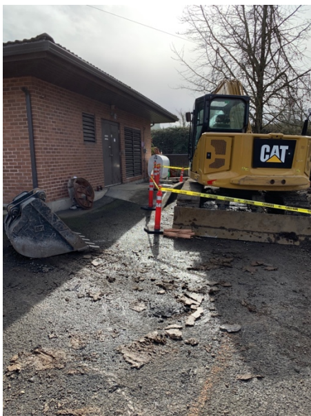
Photo 17. Proximity of excavation to pump station. View is to the S.
