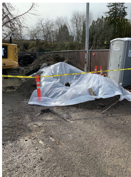
Photo 16. Stockpiled clean soil from excavation to the west of the tank pit. View is to the WSW.
