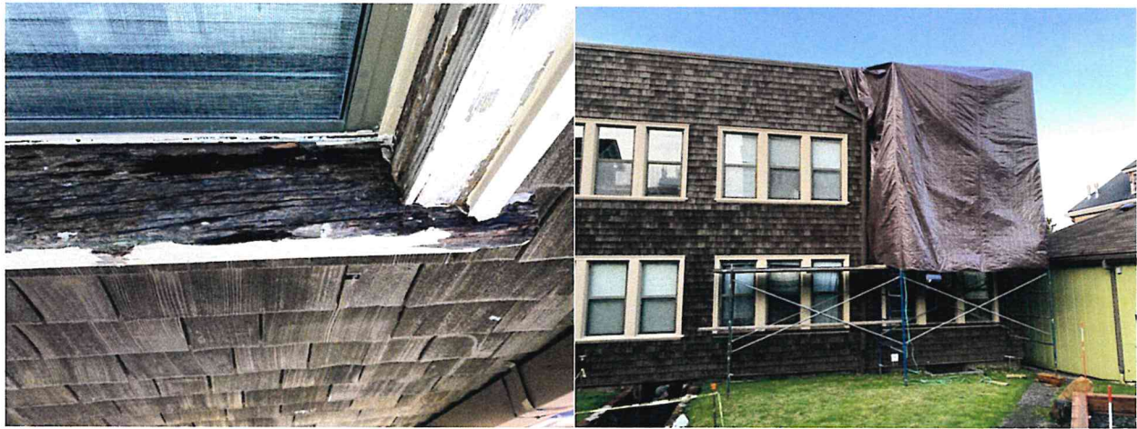
Figure 22. Window sill repair.
