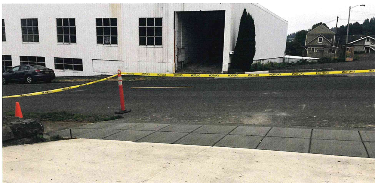
Figure 5. Finished driveway with repoured sidewalk section as per city specifications facing east.
