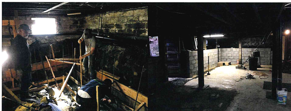
Figure 16. Setting forms and pouring concrete to stabilize the earthen dugout basement, November 2018 and nearing completion of basement stabilization, February 2019.
