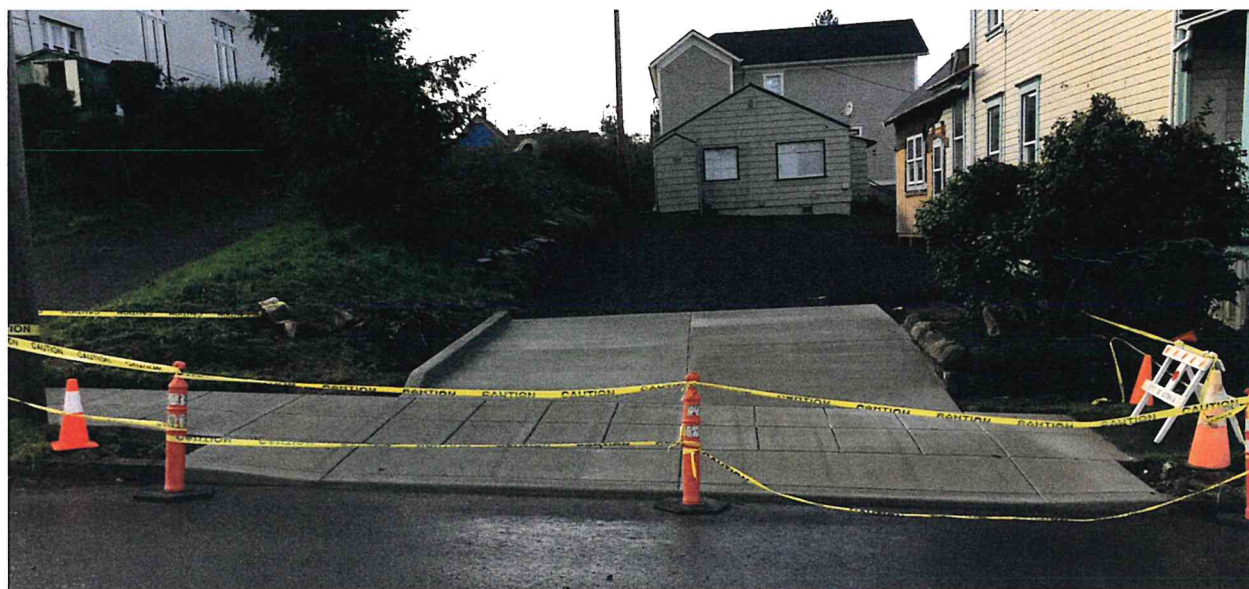
Figure 4. Finished driveway with sidewalk and concrete entry as per city specifications facing west.
