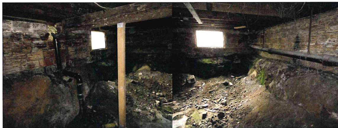
Figure 10. photos displaying poor condition of inadequately supported dugout basement with terracotta brick foundation 2018.
