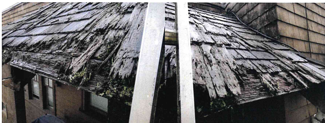
Figure 12. photos displaying rot and failure of hip roofs and gutters.
