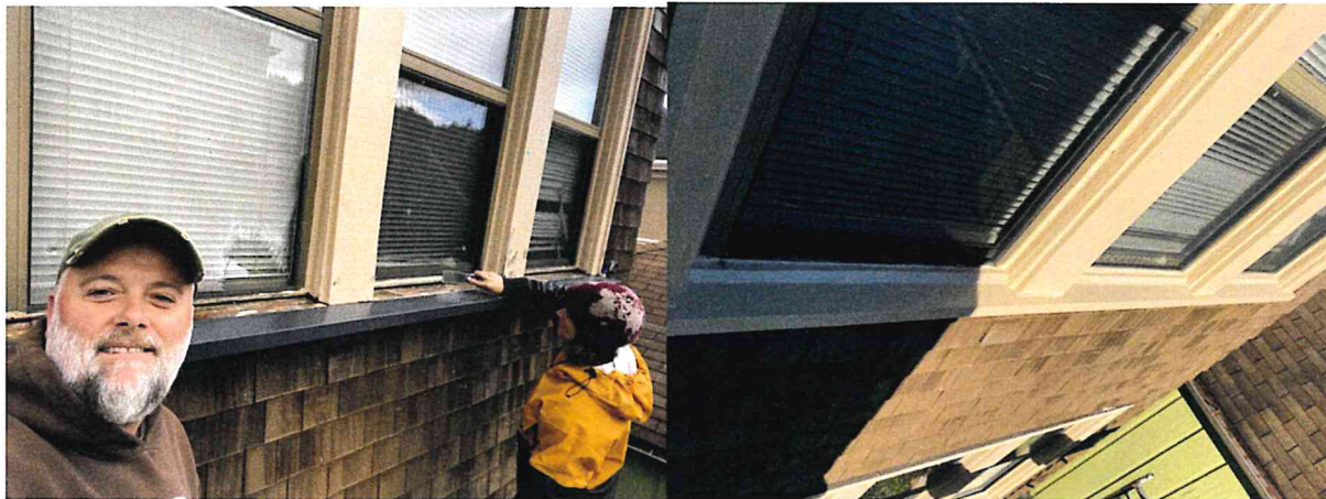
Figure 23. New metal (prior to cut and fitting) window sills installed and painted.
