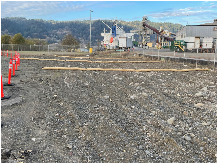
Newly completed BMPs
