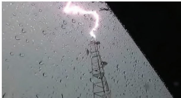
Photo: NOAA Figure 2: Lightning strikes a communications tower.
