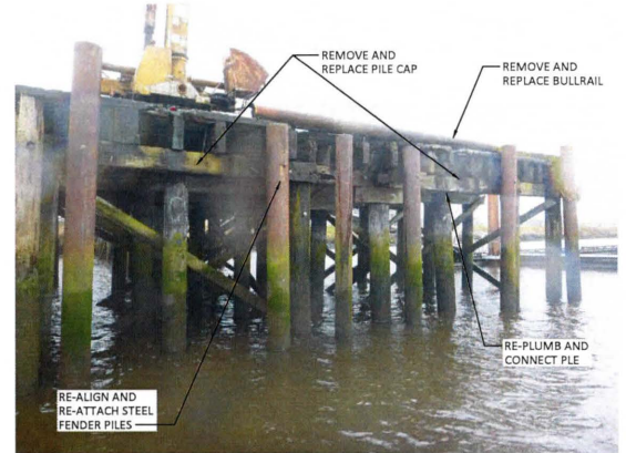
9 PHOTO - NORTH EDGE OF WEST TRESTLE SCALE: NTS
