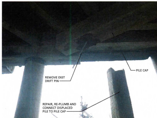
11 PHOTO - DISPLACED PILE AT WP31/D SCALE: NTS
