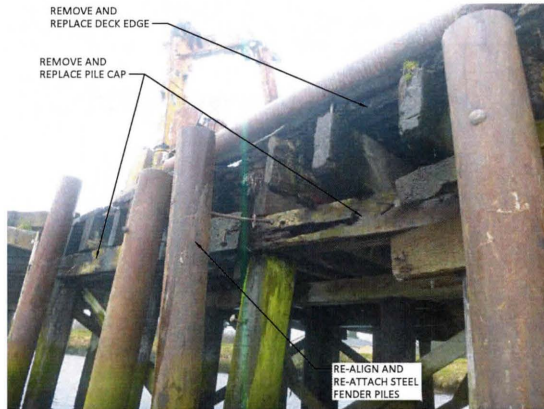
8 PHOTO - NORTH EDGE OF WEST TRESTLE SCALE: NTS
