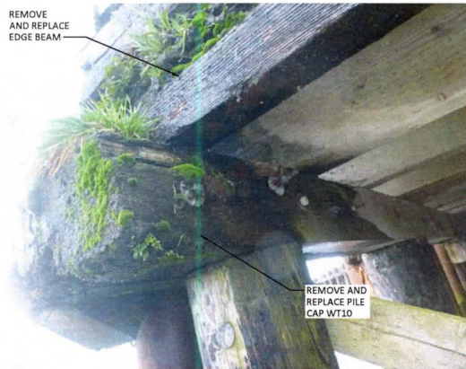
5 PHOTO - WEST TRESTLE PILE CAP WT10 SCALE: NTS
