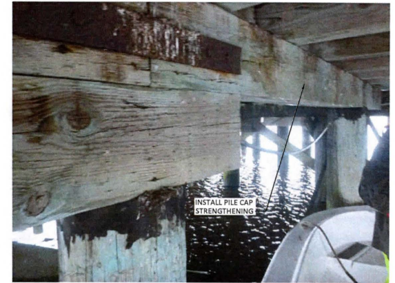
3 PHOTO - WORK PIER PILE CAP WP1 SCALE: NTS
