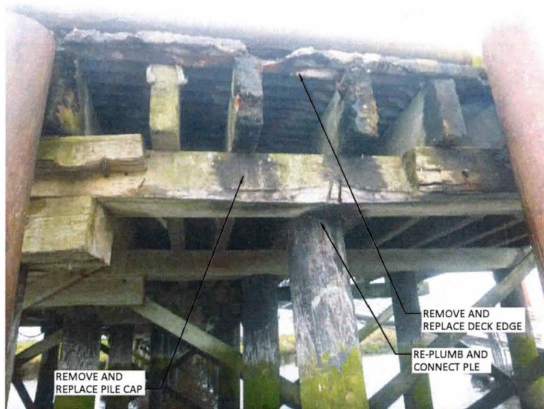
7 PHOTO - NORTH EDGE OF WEST TRESTLE SCALE: NTS
