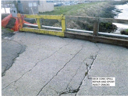
1 PHOTO - WEST TRESTLE DECK AT WT1 SCALE: NTS
