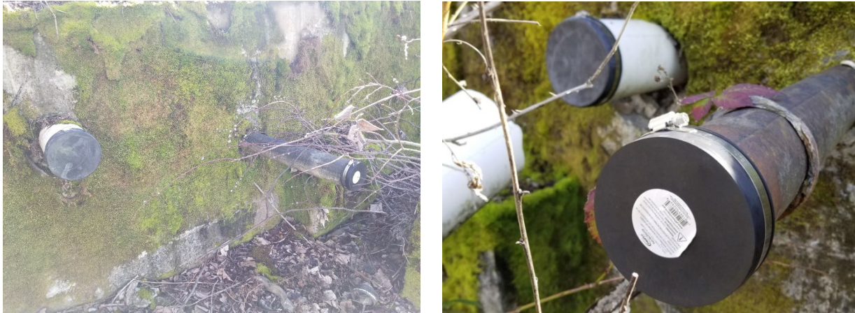
Figure 4. Basin D Stormwater SCMs (left: capped outfall STSOUT262 and STSOUT001057; right: capped outfall STSOUT263)
