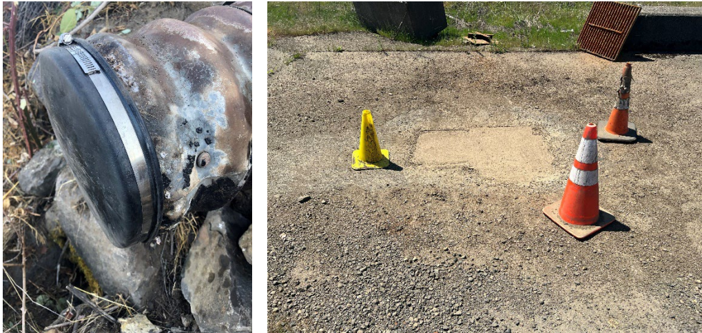
Figure 3. Basin J Stormwater SCMs (left: capped K2 outfall; right: decommissioned catch basin)
