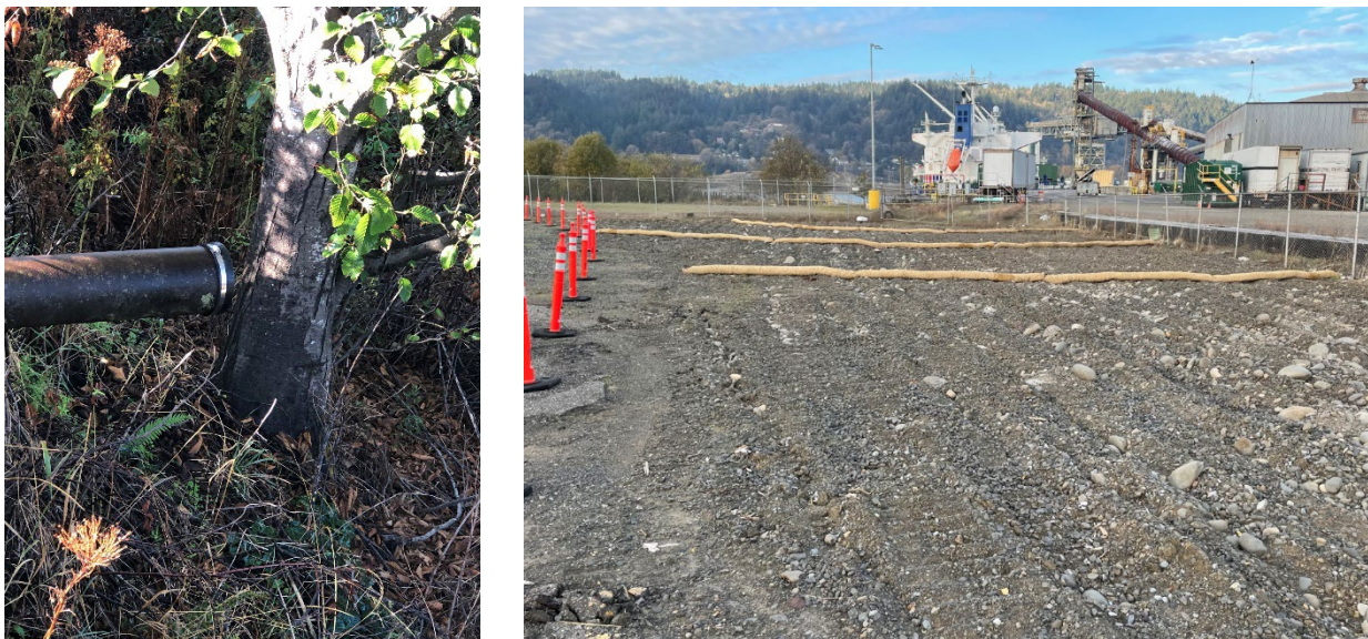
Figure 2. Basin K2 Stormwater SCMs (left: capped Basin K2 outfall; right: scarified surface and wattles)
