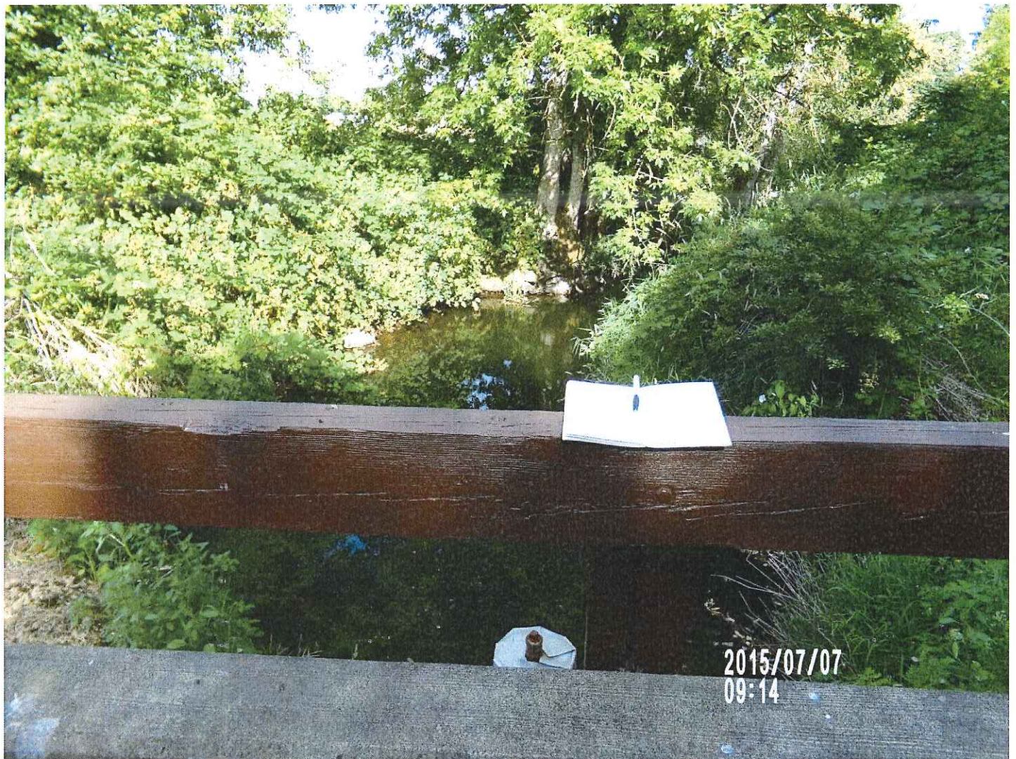
Photo 2. Bear Creek, downstream of the bridge at the facility entrance. The pool of water had no apparent flow.
