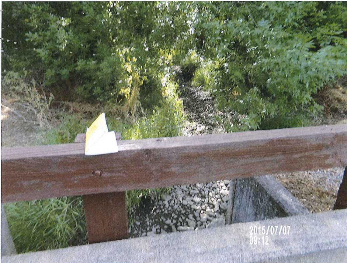
Photo 1. Bear Creek, upstream of the bridge at the facility entrance.
