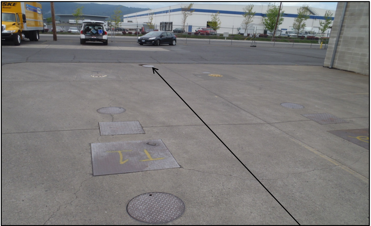
Photograph 1. Looking west at the location of the covers of the two USTs and the Observation Port Cover (background center) between them. 5-6-2013.
