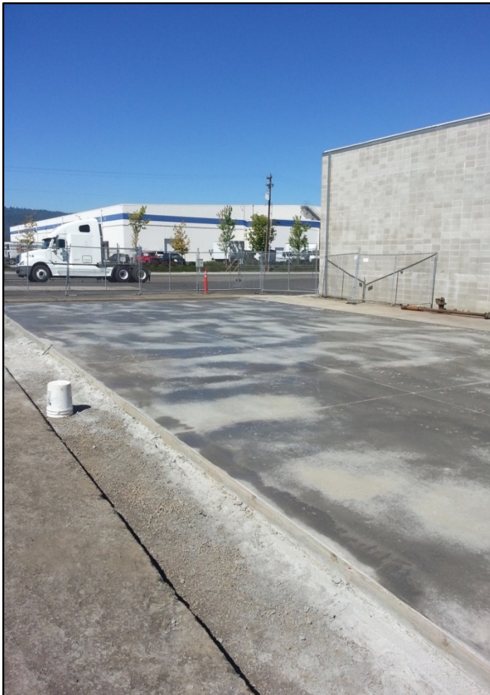
Photograph 8. Looking west just after the new concrete pad has been poured. 9-9-2013
