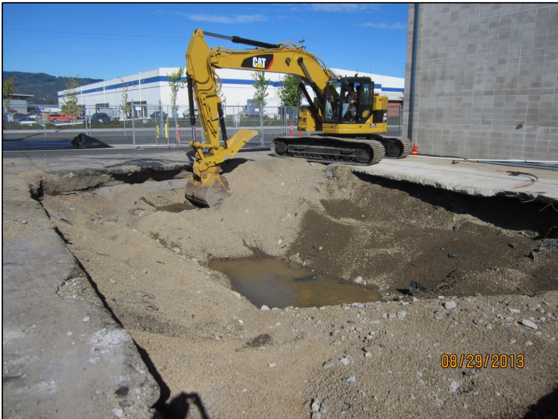
Photograph 5. Looking west as groundwater recharges the recently dewatered excavation following UST removal. 8-29-2013.
