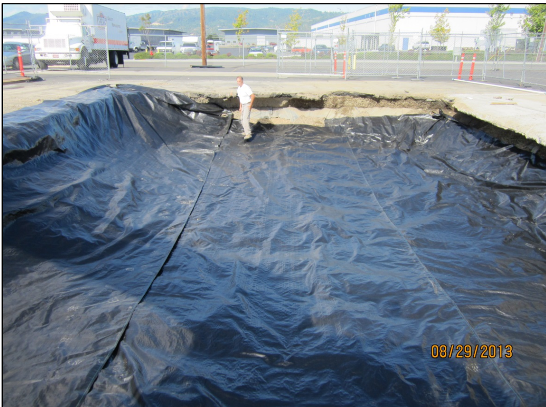
Photograph 6. Looking west at laying the liner prior to backfilling. 8-29-2013.
