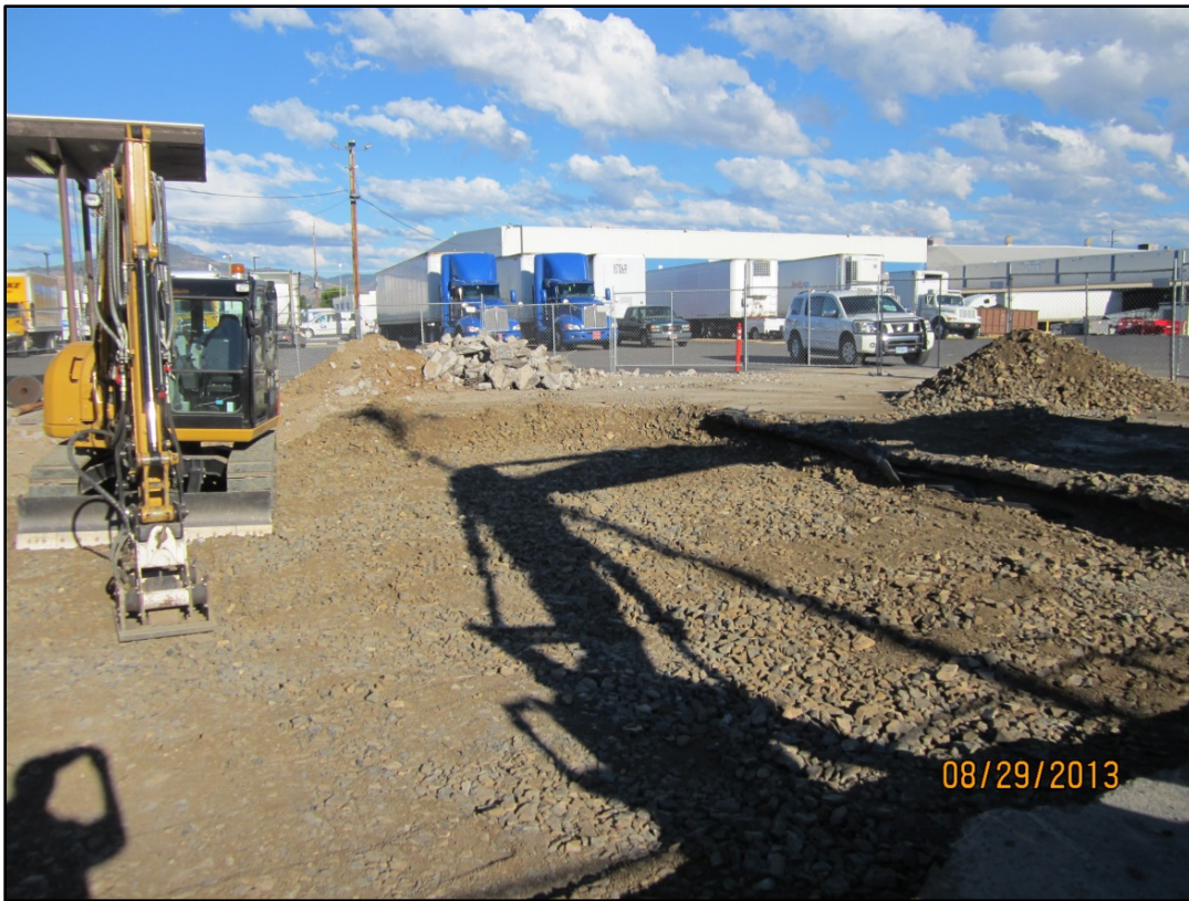
Photograph 7. Looking east as backfill is compacted. 8-29-2013.
