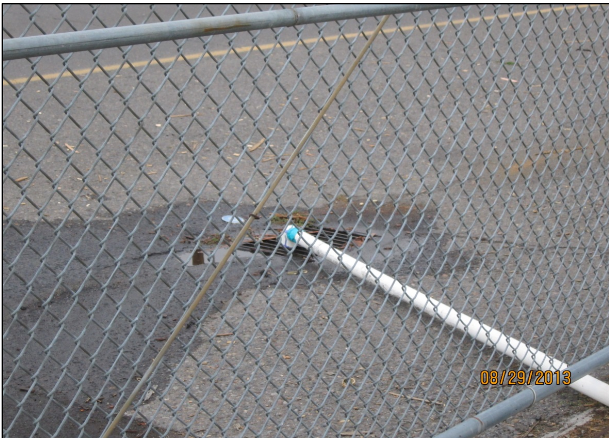
Photograph 4. Dewatering to the nearby storm drain along Joseph St. 8-29-2013.
