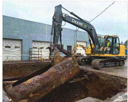
An environmental consultant removing an old steel underground storage tank.
