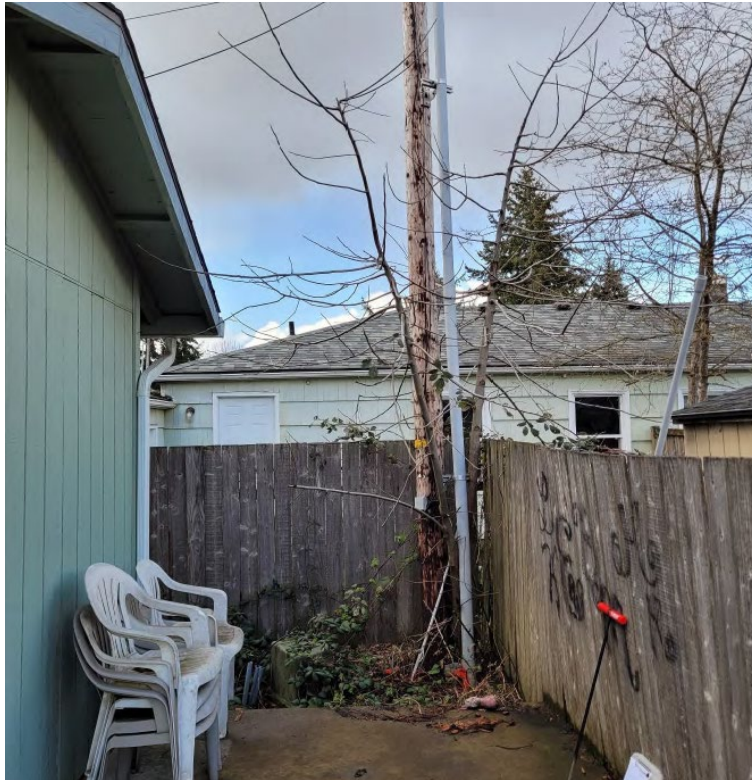
Photograph shows the east side of the ADU and the northeast corner of the property, which contains a power pole and a small area of soil to be removed. The tree shown will be removed but its stump removal will be the responsibility of the earthwork contractor. The power utility may need to be contacted to assist with removal in this area. Photograph taken facing north.
