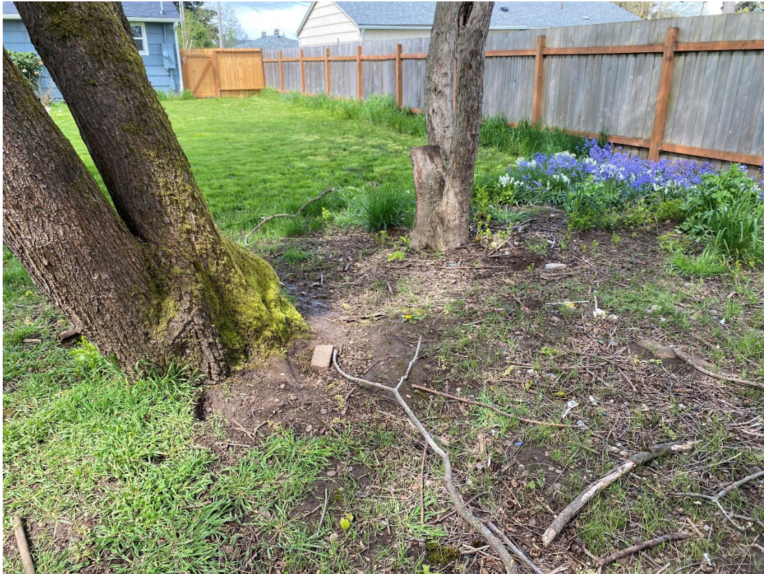
Photograph shows the north side fence to be partially removed for access. Removed fence will be replaced. Photograph taken facing northwest.
