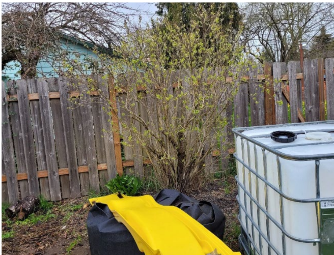
Photograph shows a shrub to be removed from the backyard and replaced (along with all shrubs on this fence line) following remedial action. Photograph taken facing north.
