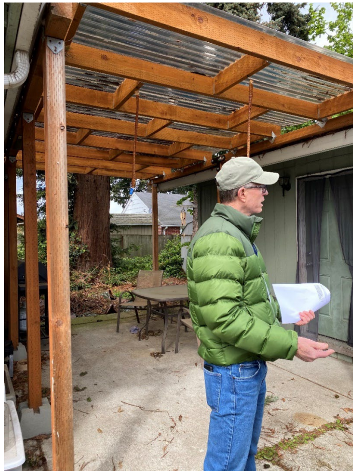
Photograph shows the overhead cover between the house and the ADU, which may need to be removed for equipment to access the west side of the yard. Photograph taken facing northeast.
