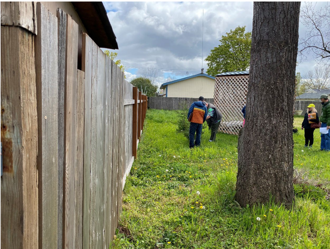
Photograph shows the other side of the structure to be removed for excavation, plus a tree that will be removed prior to remedial action. The stump removal will be the responsibility of the earthwork contractor. Photograph taken facing east.
