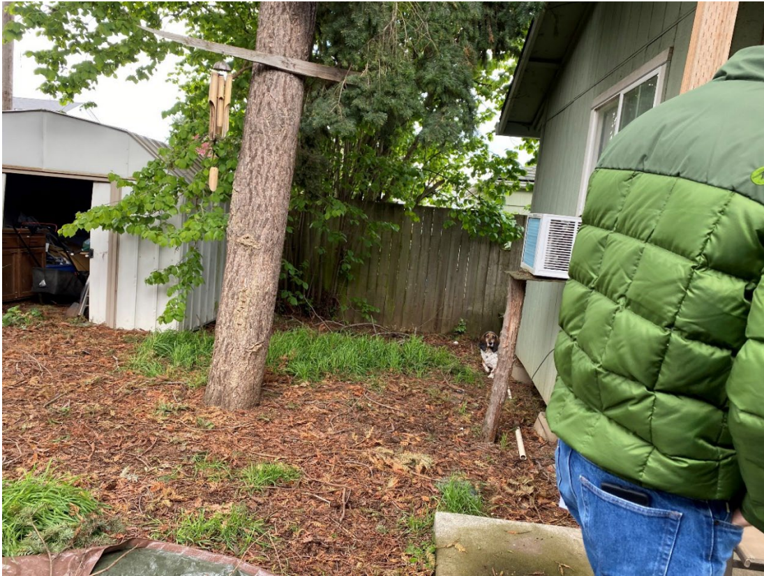
Photograph shows the west side of the ADU and east side of the shed to be removed from the property. The tree shown will be removed prior to remedial action but its stump removal will be the responsibility of the earthwork contractor. Photograph taken facing north.
