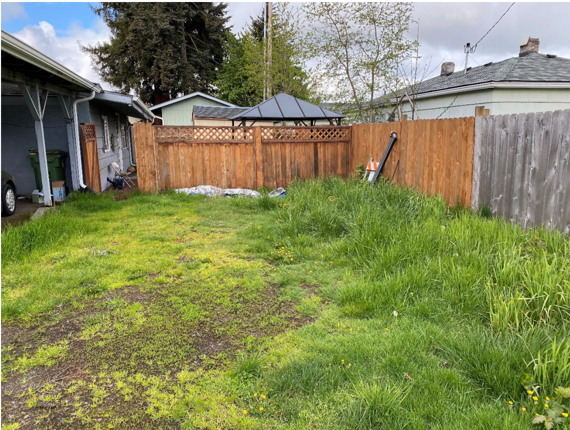
Photograph shows the access point to the north side of the backyard. The fence will need to be removed and replaced for access. Photograph taken facing west.
