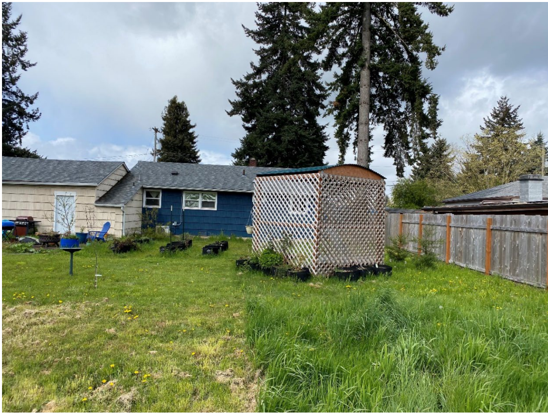
Photograph shows structure to be removed for excavation (will be rebuilt after remedial action) and north side fence to be removed for access. Any removed fencing will be replaced. Photograph taken facing west.
