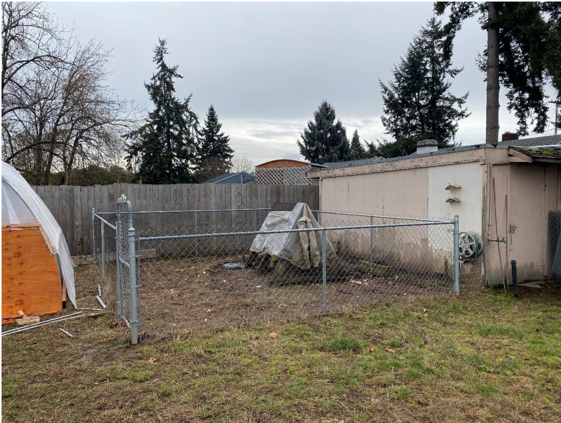
Photograph shows the chain-link fence pen that will be removed to provide access to the backyard. The fence behind it (between DU-15 and SO-07) will also be removed. Any removed fences will be replaced. Photograph taken facing south.
