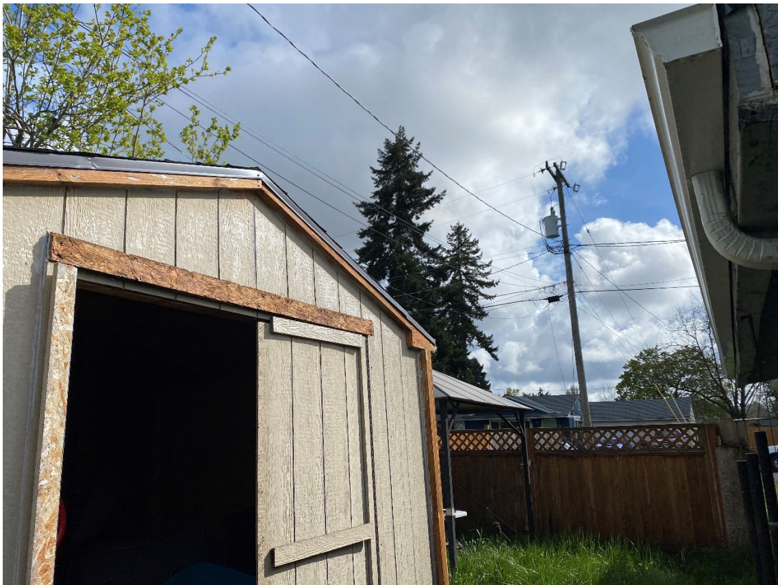
Photograph shows shed to be removed (not replaced) from the northside backyard. Photograph taken facing southeast.
