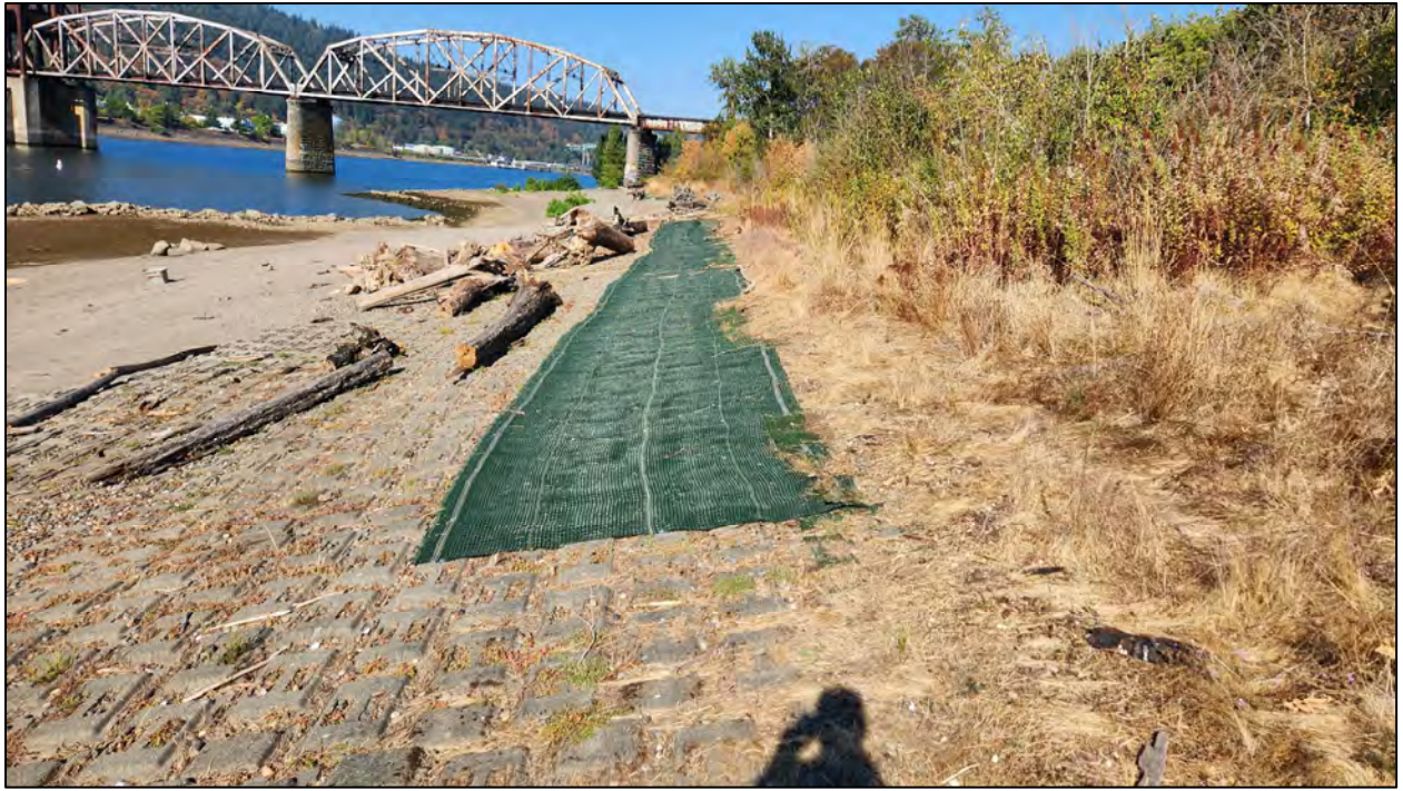
Photograph 5: TRM repair area in on northern end of Willamette River shoreline at the site. View facing north.
