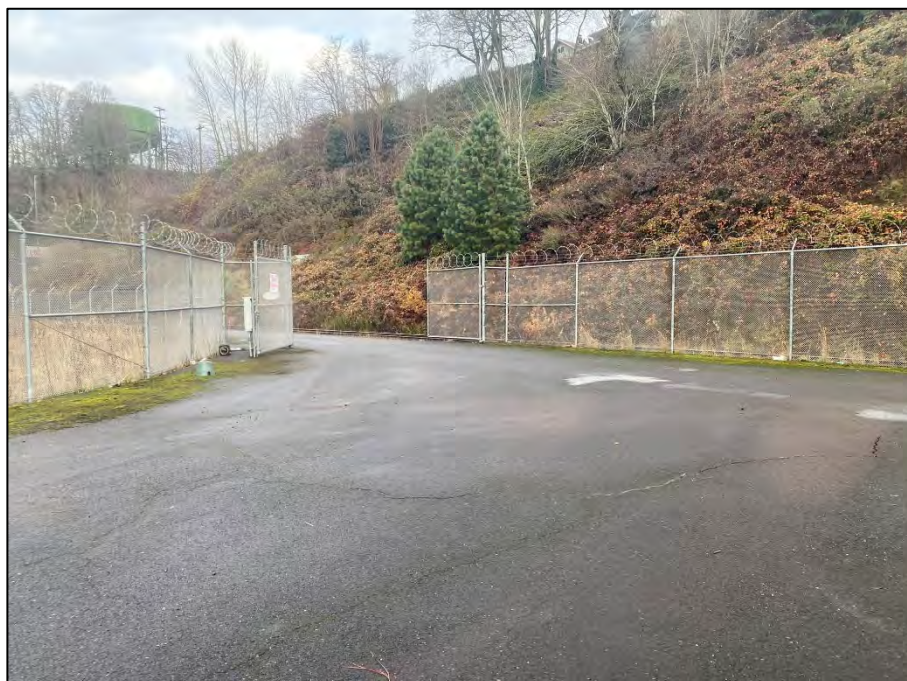
Photograph A4: Main entrance gate found unlocked and open upon arrival to the site for trash dumpster emptying. December 2022.
