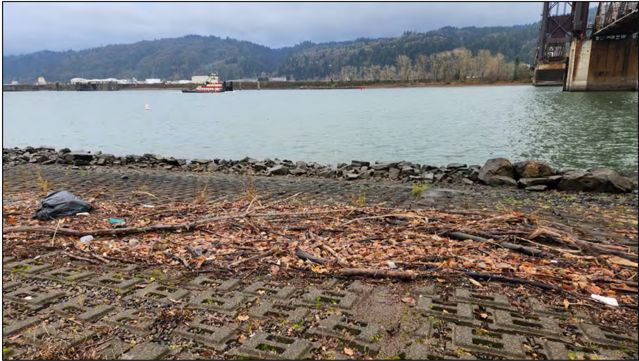
Photograph 3: ACB matting where shrub trees were removed during O&M visit. View facing west southwest.
