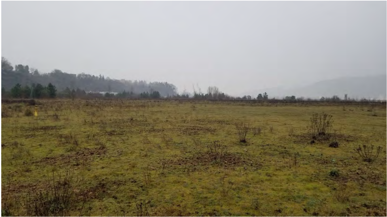
Photograph 7: View of the soil cap from the center of the cap facing southeast.
