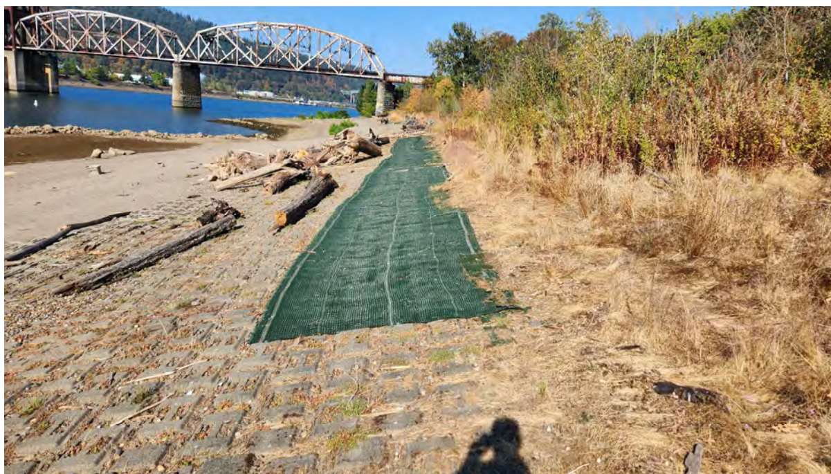
Photograph A12: TRM replacement repair area along Willamette River Shoreline. September 2022.
