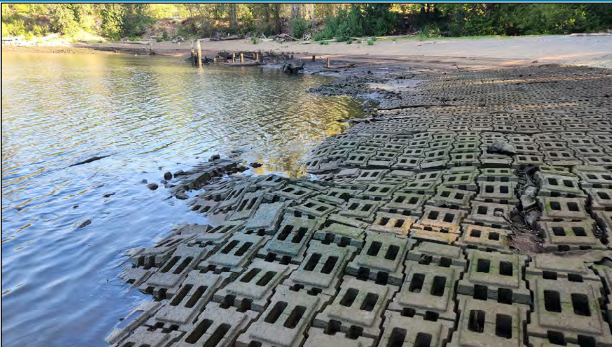
Photograph A7: Undulations and unconformities in ACB in Willamette Cove. September 2022
