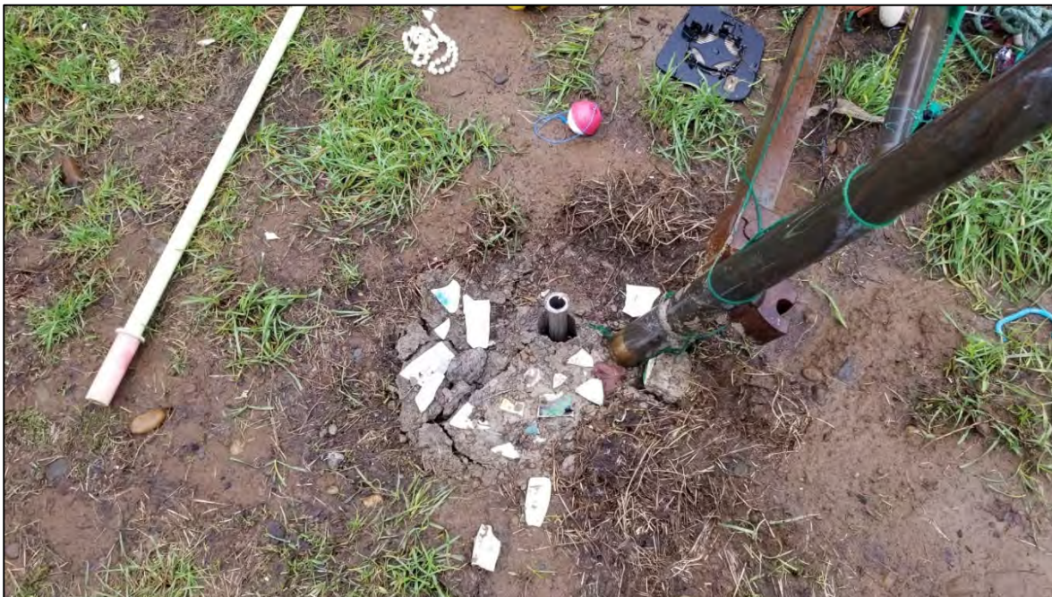
Photograph A3: A portion of the “art installation” that was cemented into the soil cap. March 2022.
