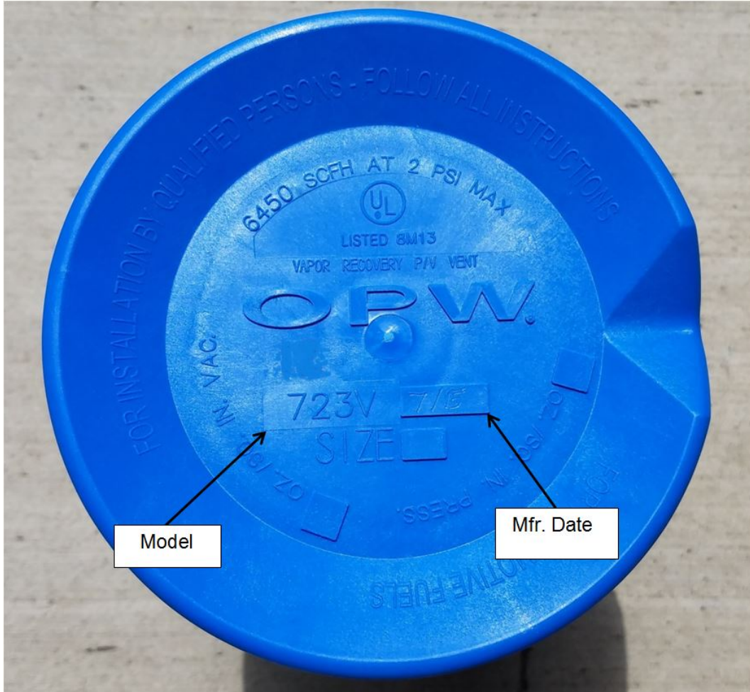
OPW Model 723V P/V Vent Valve
