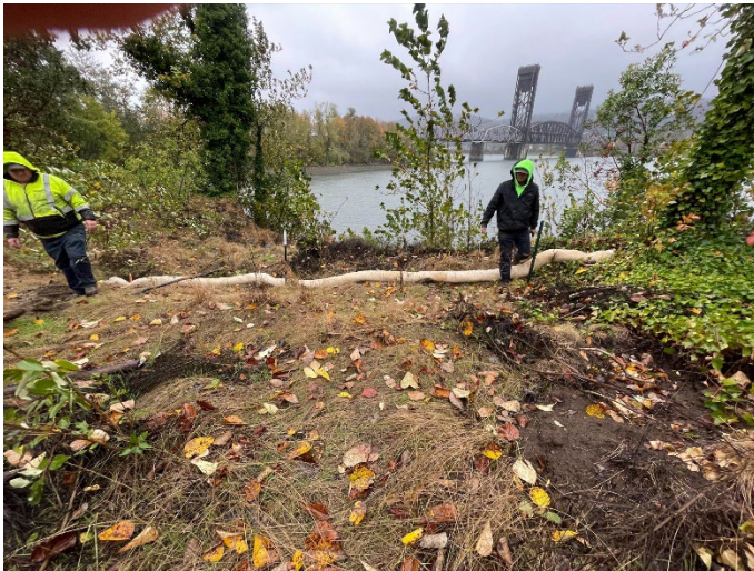
Installation of straw wattles near top of bank
