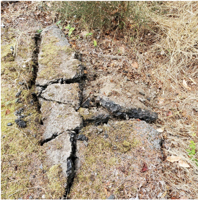
Edge of pavement in DU-23. Pavement is approximately 2-3 inches thick and easily removed using the excavator.
