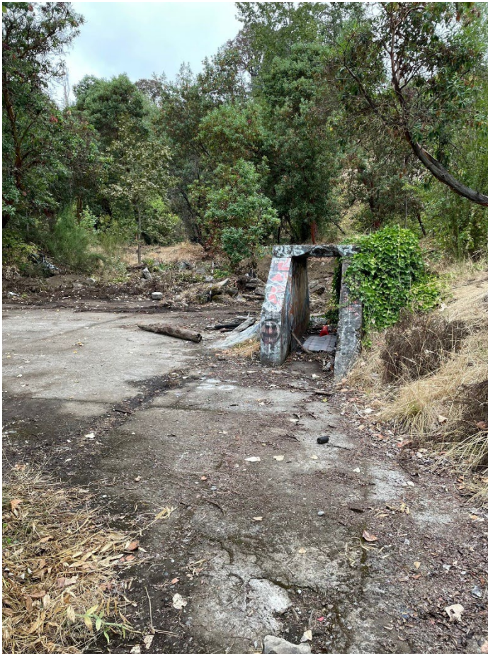
Concrete in DU-16. Slab in foreground appears to be continuous to the north beneath the rubble in background, view is to north.
