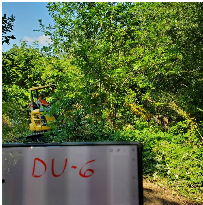
DU-6 vegetation clearing
