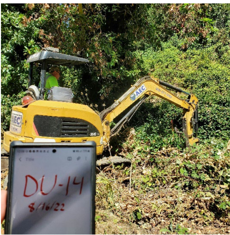
Excavating increment for DU-14
