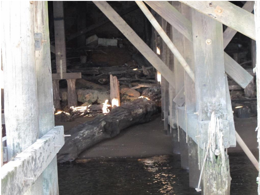
PIER 51 CLOSE UP
