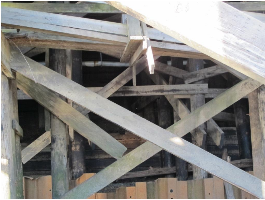
PIER 33 CLOSE UP
