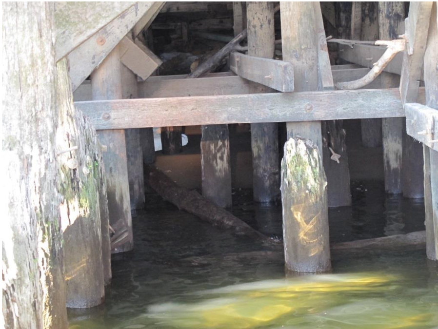
PIER 44 CLOSE UP
