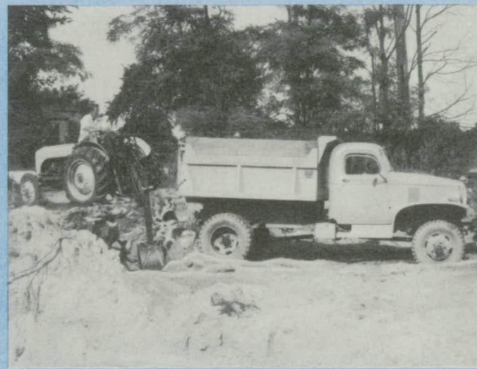
Digging irregular shaped hole from one position.
