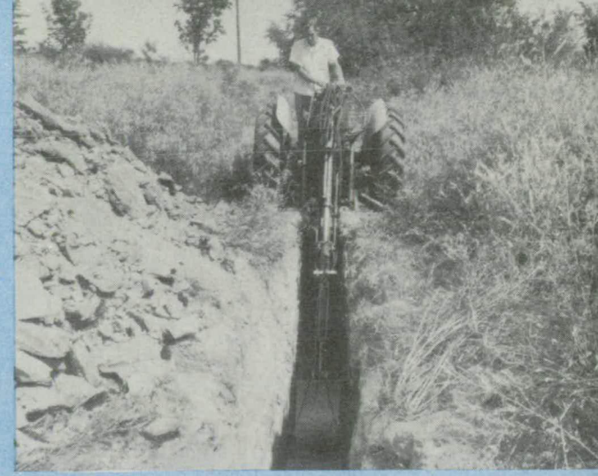
Digging and loading with back hoe bucket.
