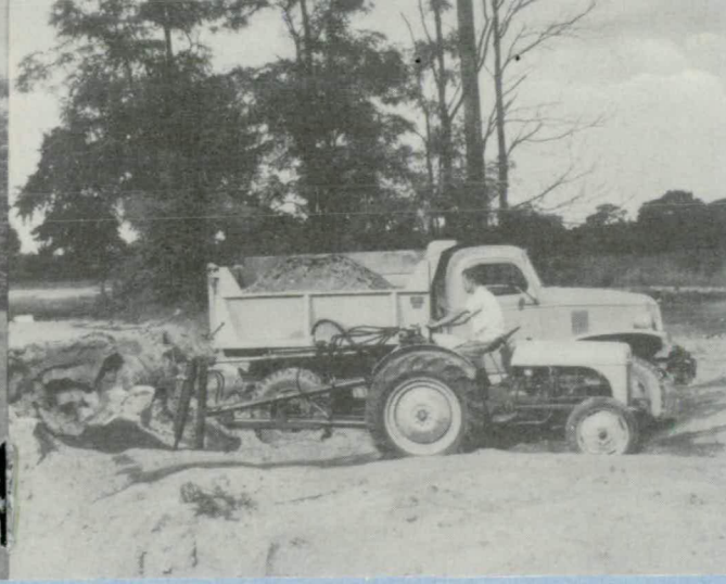
Digging and loading with back hoe bucket.
