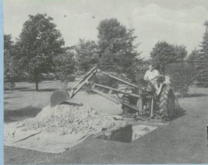
Basement dug from four positions of tractor.
