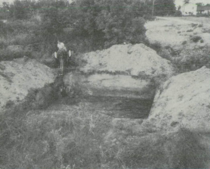
Basement dug from four positions of tractor.
