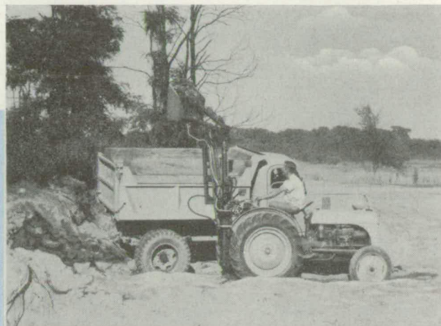
Loading clearance with loading shovel, 10 feet
