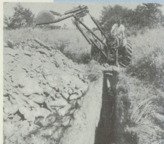
Maximum digging depth, 8 feet
