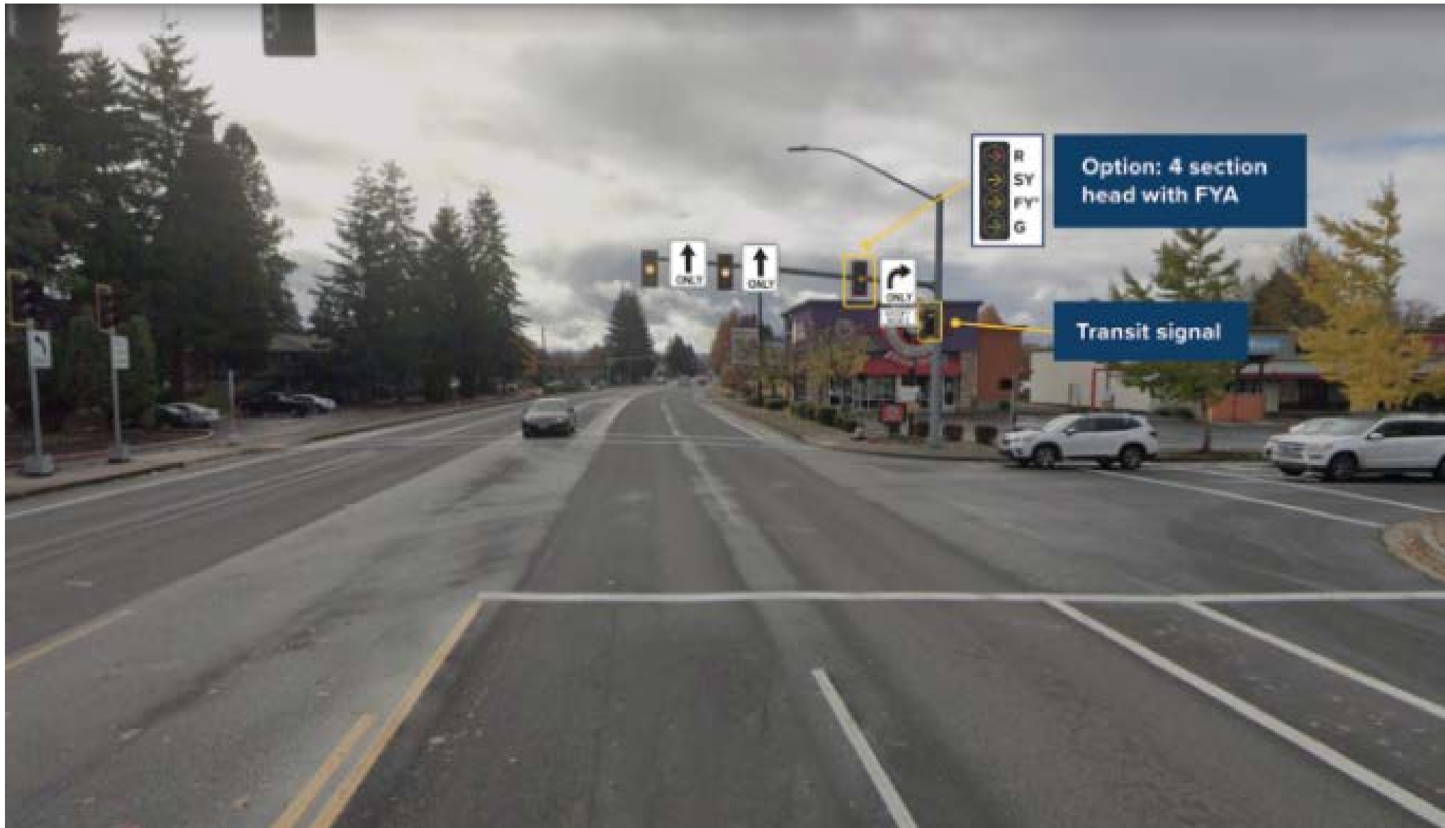
EXAMPLE SIGNALIZED INTERSECTION TREATMENT INSTALLATION (APPLIES TO QUEUE JUMP AS SHOWN OR THROUGH BAT LANES)
