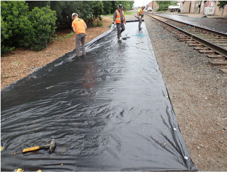
Using a pneumatic nail/staple gun to secure the long edges of the geotextile in chip bedding (left) and gravel ballast (right) – view northwest.
