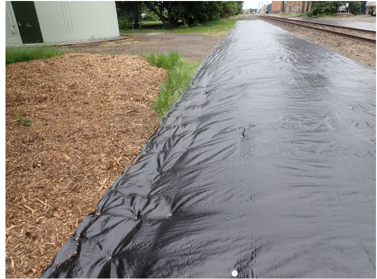
Multiple rows of staples were used to secure the west long edge of the geotextile in wood chip bedding.
