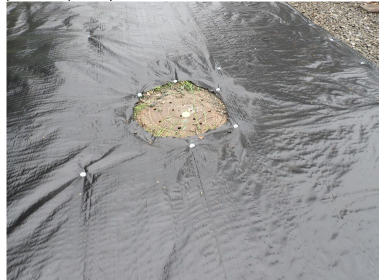
Geotextile was fitted around a manhole cover to ensure it could be accessed, if needed..
