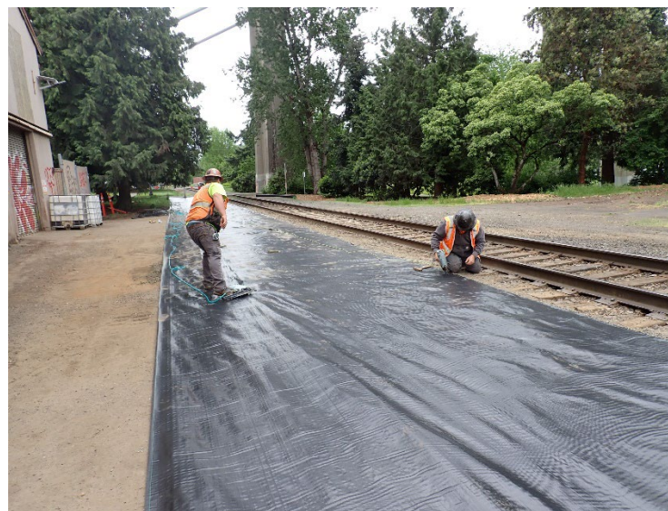
The geotextile was installed against, and secured to, the edge of the asphalt pavement west of the PIW building – view southeast.
