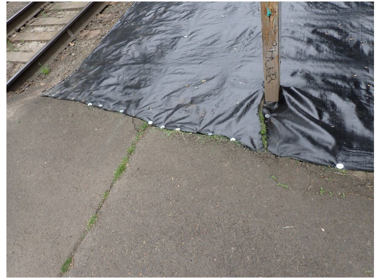
Close-up showing the short edge of geotextile secured to asphalt pedestrian pathway.
