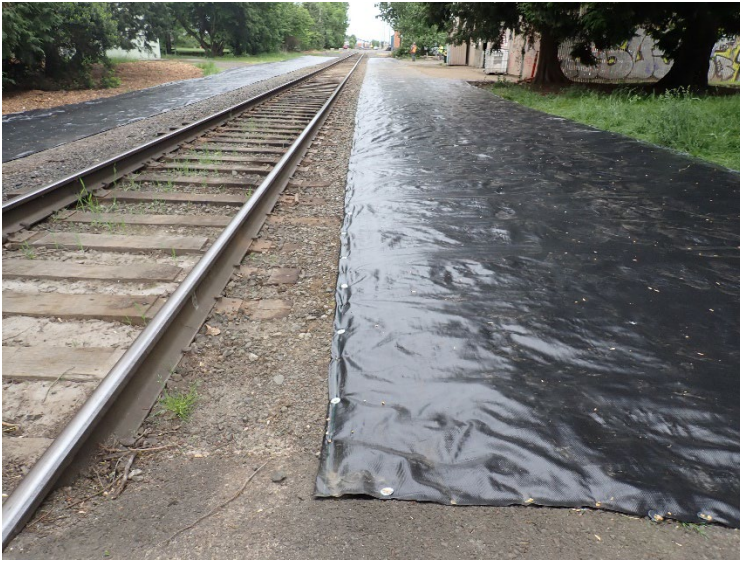
Completed temporary mitigation on the upgradient east side of the railroad ROW – view northwest.
