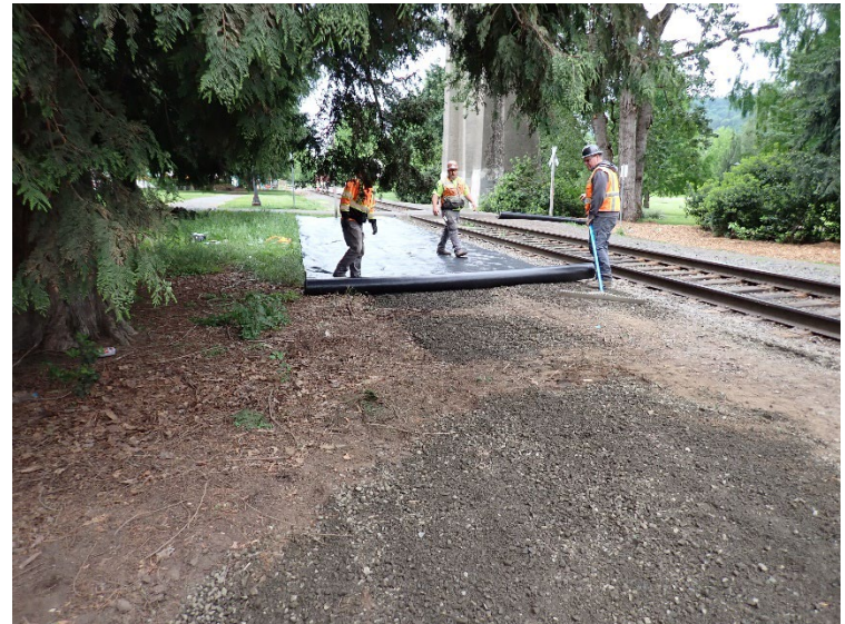
Deploying a 12-foot-wide roll of heavy-duty geotextile starting at the southeast (uphill) side of railroad ROW.
