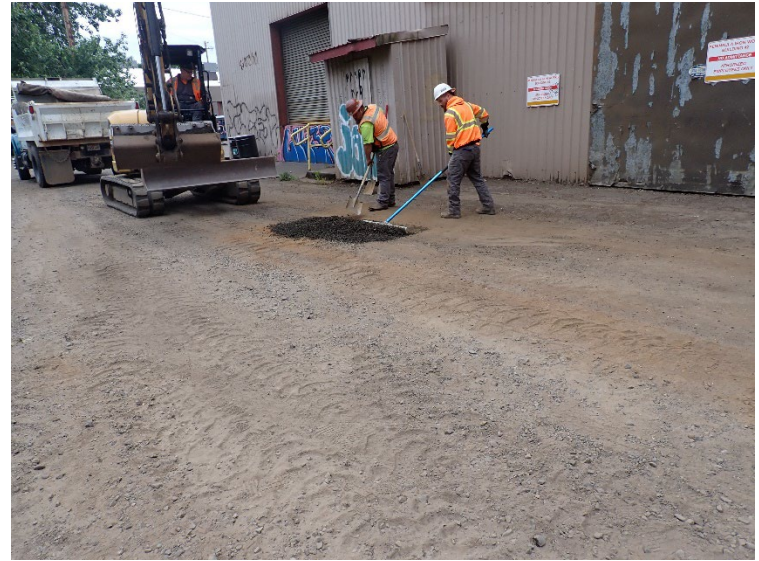
Workers filling a low spot next to PIW building with clean imported crushed rock prior to geotextile installation.
