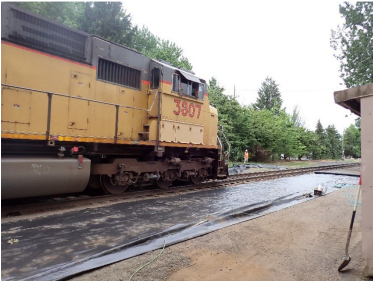
Rail Pros removed derailment measures and asked workers to stand back 8 feet while a north-bound train passed through the work area.
