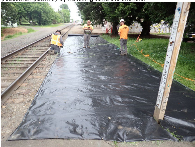
Using a pneumatic nail gun to secure the long edges of the fabric in gravel (left) and grass landscaped areas (right) – view northwest.
