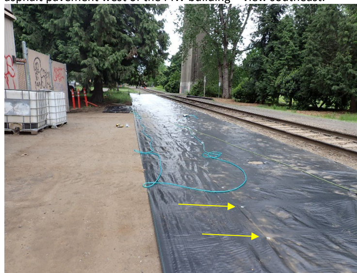
Nails fitted with washers were used to secure the middle of the geotextile.
