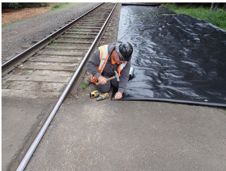
Securing the southeast end of the geotextile to the asphalt-paved pedestrian pathway by installing concrete anchors.
