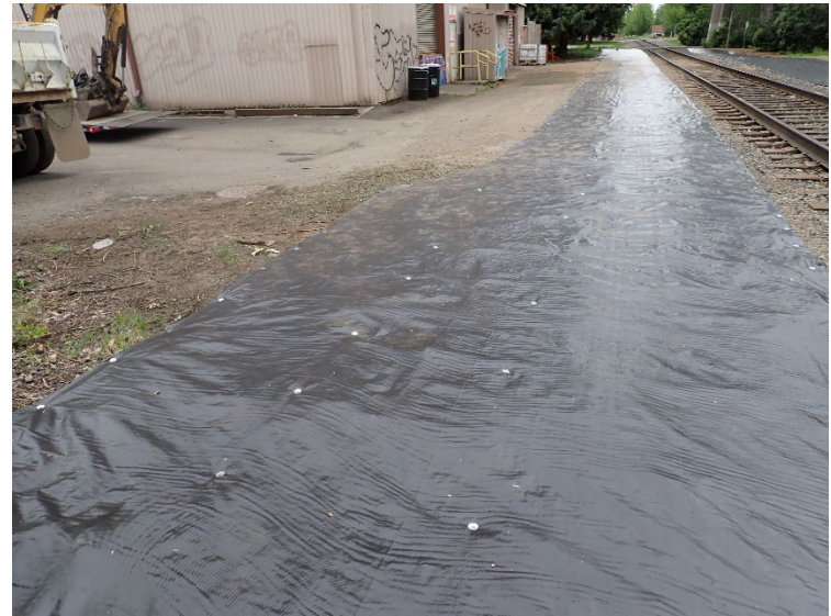
Completed temporary mitigation on the upgradient east side of the railroad ROW – view southeast.
