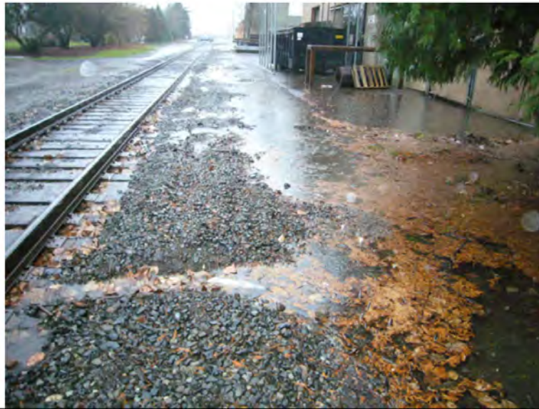
Photograph 1: Extensive Ponding Adjacent to the West Side of the PIW Building and Along the N. Bradford Street ROW circa 2012
