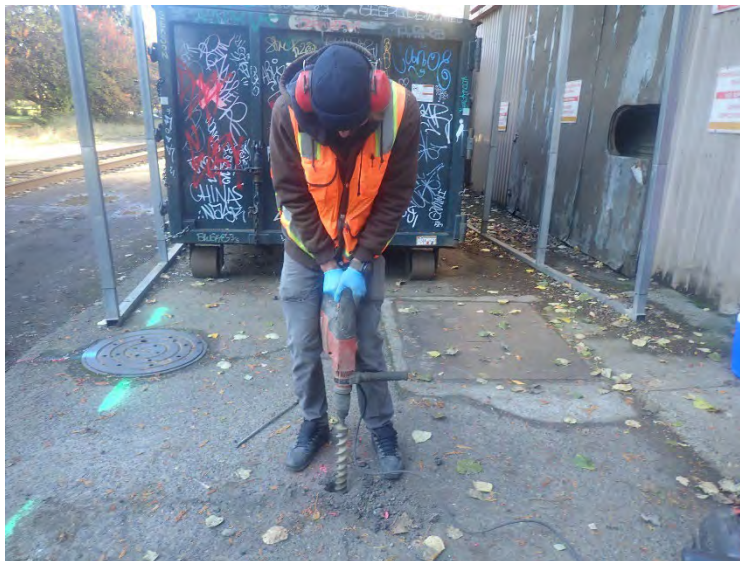
A roto hammer was used to penetrate the concrete apron at boring B04 on west side of PIW bldg.
