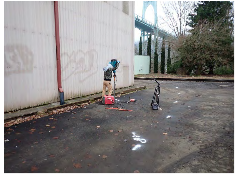
Drilling B41 on the north side of the PIW building, looking west.
