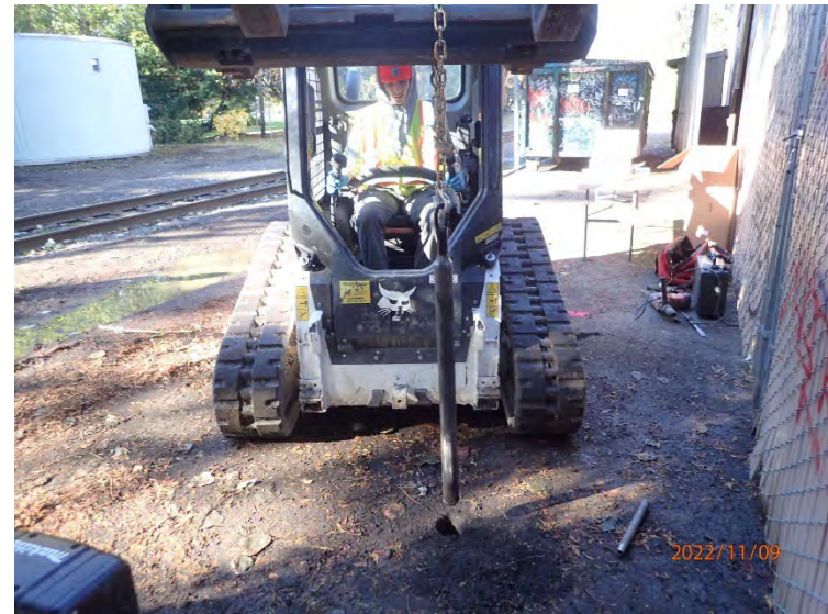
Using a skid steer to retrieve DPT sample core from boring B05 along the west side of the PIW building at B01.
