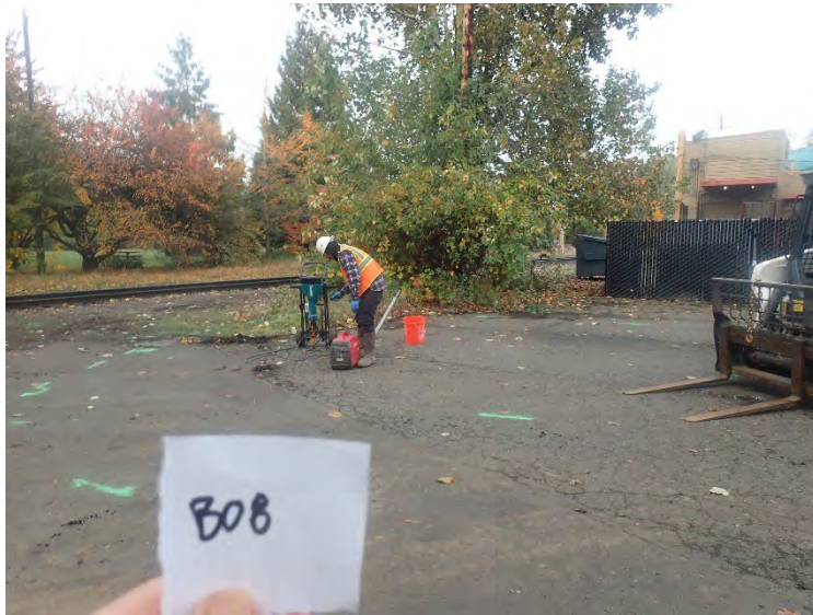
View of B08 at west end of N. Alta Avenue ROW.
