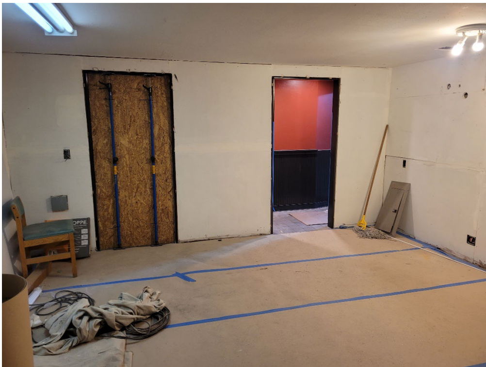
Looking South in existing prep kitchen ingress and egress points.
