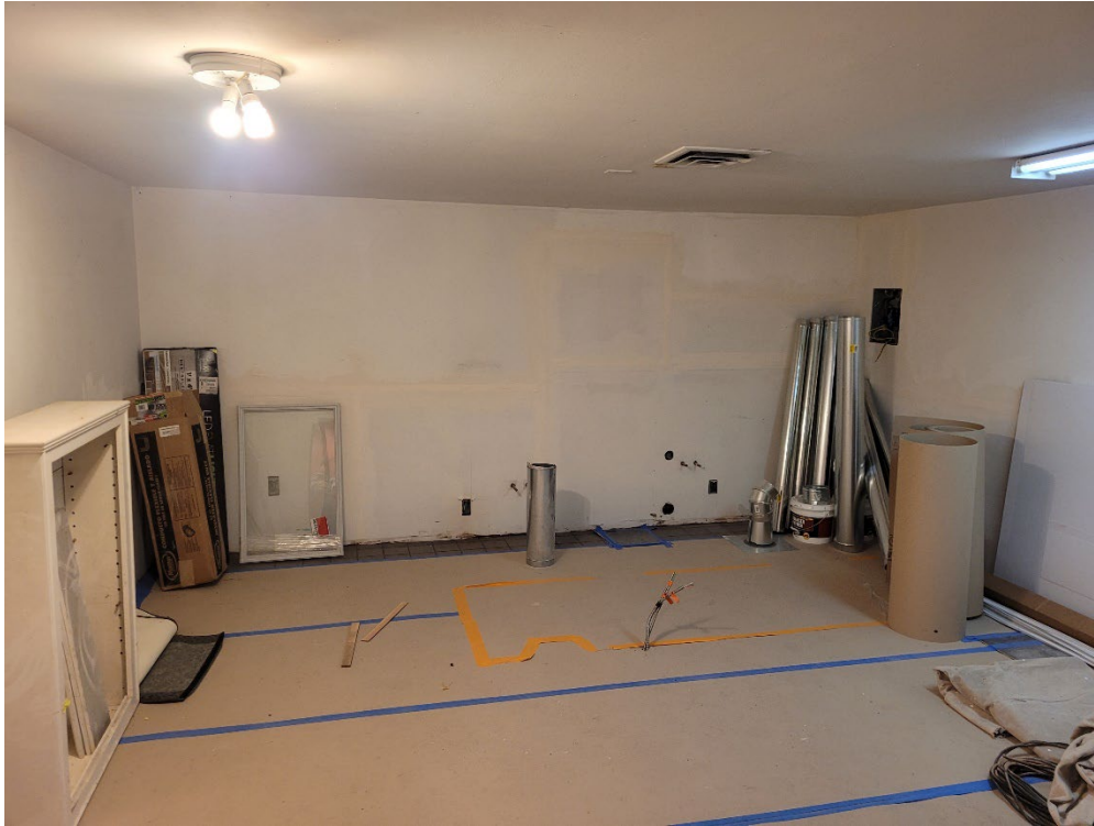
Looking North in existing prep kitchen rough-in.
