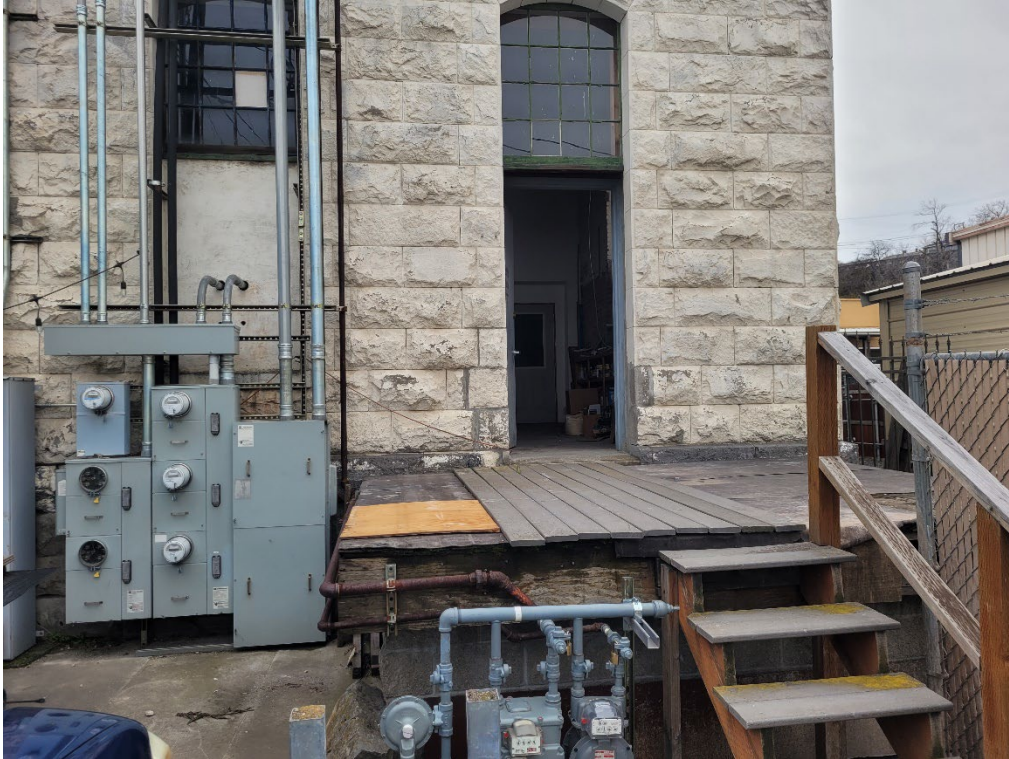
Existing shipping and receiving dock and current Natural Gas utility location.
